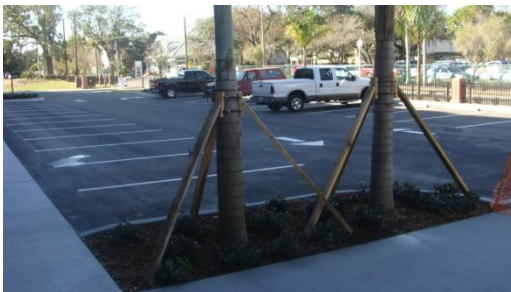
West side, parking
