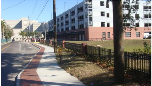
West side, towards North
