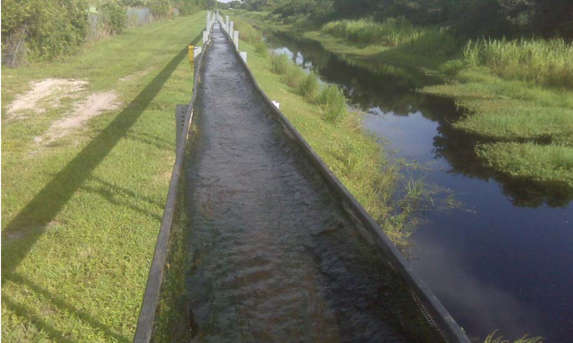
Figure 1: Powell Creek ATSTM (PC-ATS) Mobile Pilot Unit in Operation
