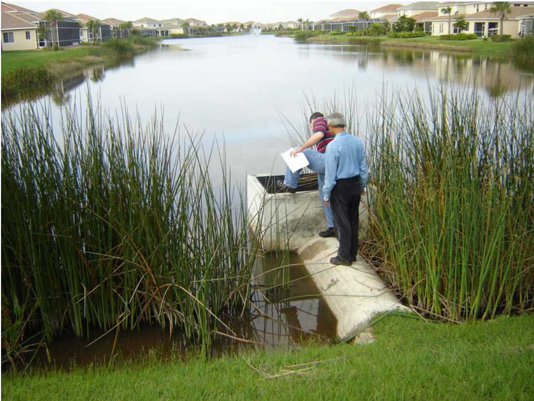
Laguna Lakes – Outfall Control Structure
