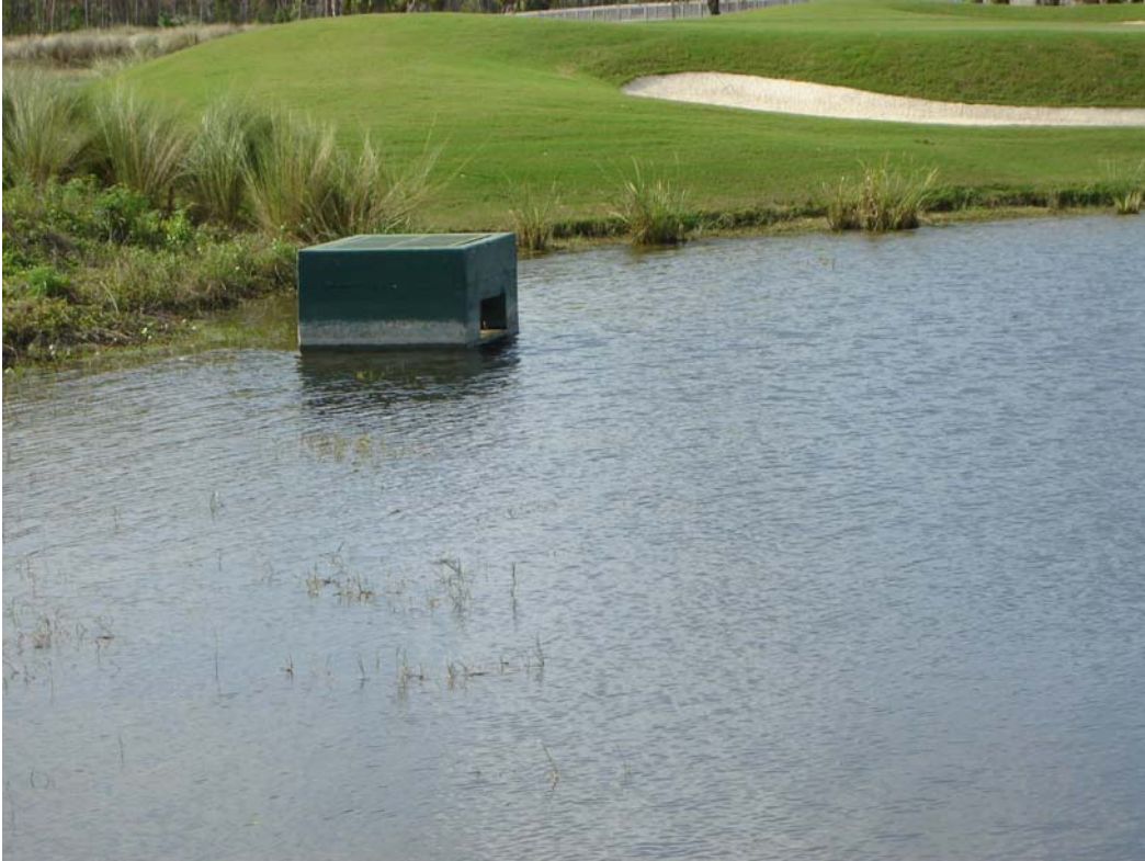
The Brooks – Outfall Control Structure
