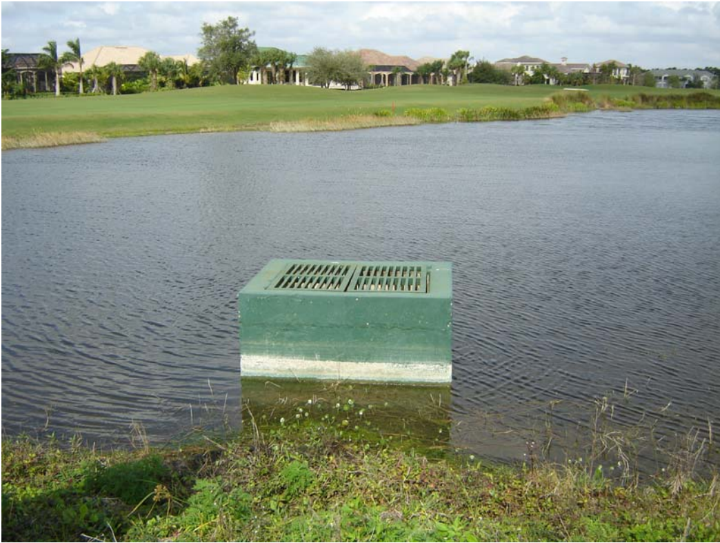
The Brooks – Outfall Control Structure
