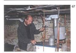
Recommended:[67] A professional energy auditor analyzes the performance of an existing furnace to ensure it is operating efficiently.
