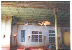
**Recommended:** [62-63] Carefully installed new mechanical ductwork is barely visible in the elaborately decorated ceiling of this historic theater.
