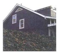
Recommended: [55-57] Wood vents in the gable ends of a historic house and a barn and cast-iron oval vents in a masonry foundation traditionally helped air circulate.
