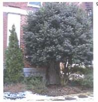
Not Recommended: [97] This tree, which was planted too close to the building, has caused the masonry wall to retain moisture that damaged the mortar and required that the brick be repointed in this area.
