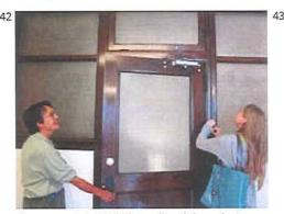
Recommended: [43] The wall and door glazing ensures that the corridor receives natural daylight and the operable transom helps air to circulate in this historic office building.
