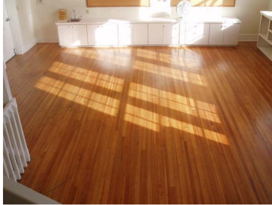
New Floor in Munchkin Room, Boca Grande
