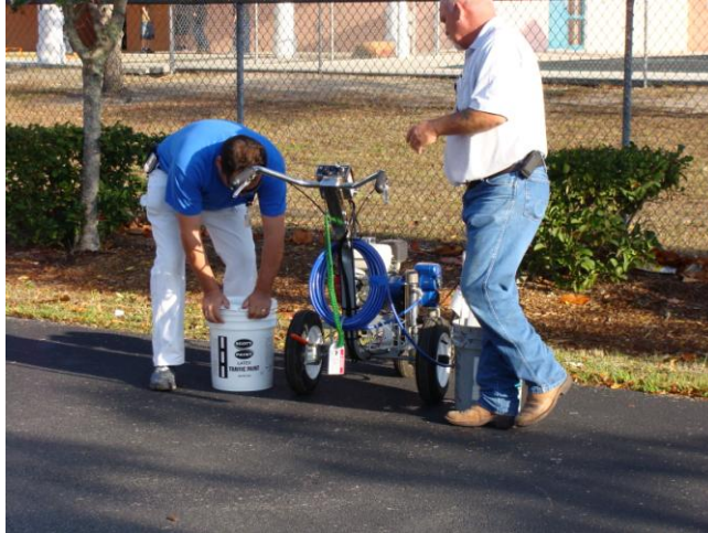
Restriping Machine Being Set Up
