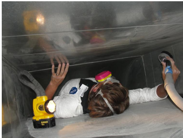
A trades person cleaning ventilation ducts
