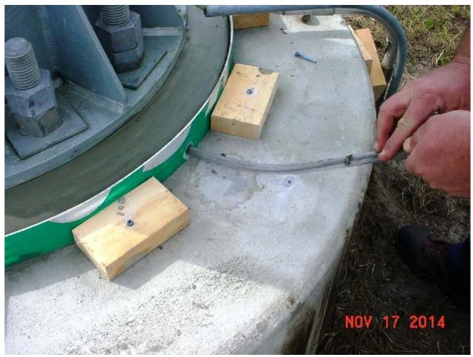
When the grout is set enough remove rod base plate, rod, and tube from the foundation.
