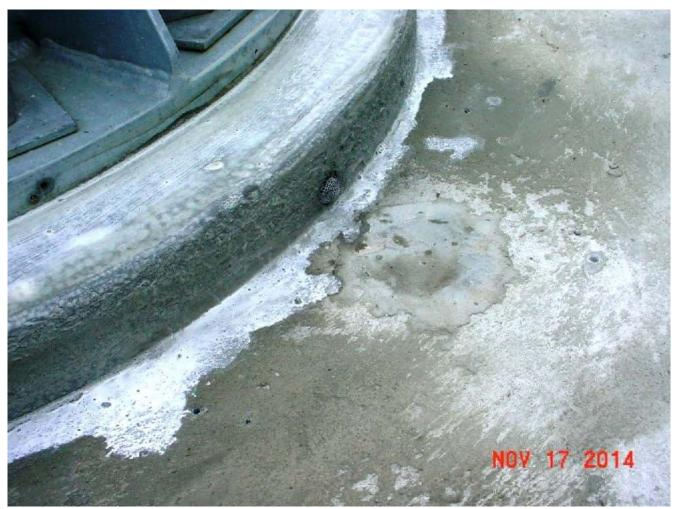
The preformed screen is then inserted into the drain hole to keep out debris and vermin.
