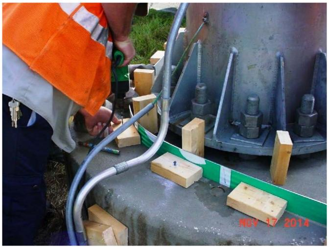
The form is then installed to the top of the foundation with tap-cons and spacer blocks.
