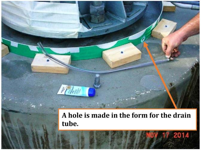
A ¼ inch rod is pre-formed with a base plate and inserted inside the tube to hold the tube in the proper position until the grout has set.
