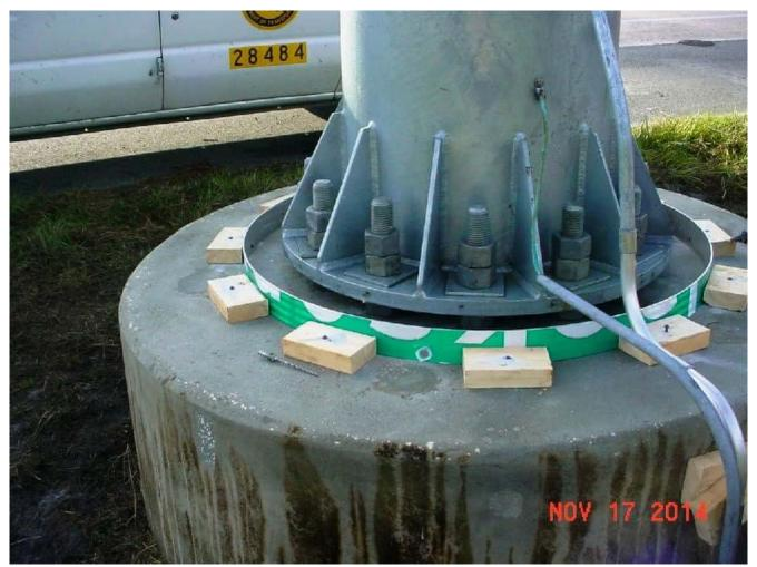
The form is now installed where the top of the form is above the bottom of the structure base plate.
