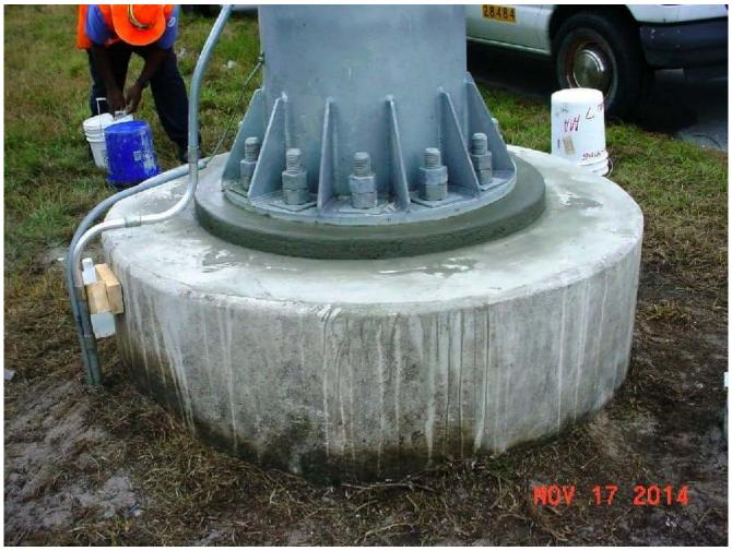
After the grout has cured, remove the form.
