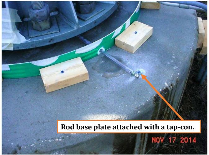
The lubricated tubing is then installed on the rod and inserted thru the form and the base of the rod is screwed to the top of the foundation to hold it in place.
