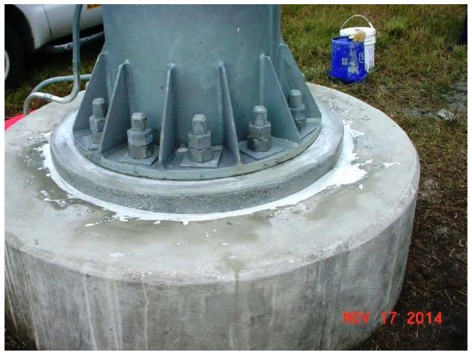
The grout is then sealed with a curing compound.
