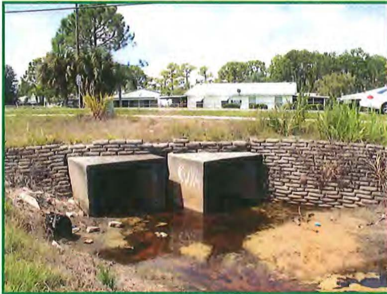
Double 7 ft x 5 ft concrete box culvert
