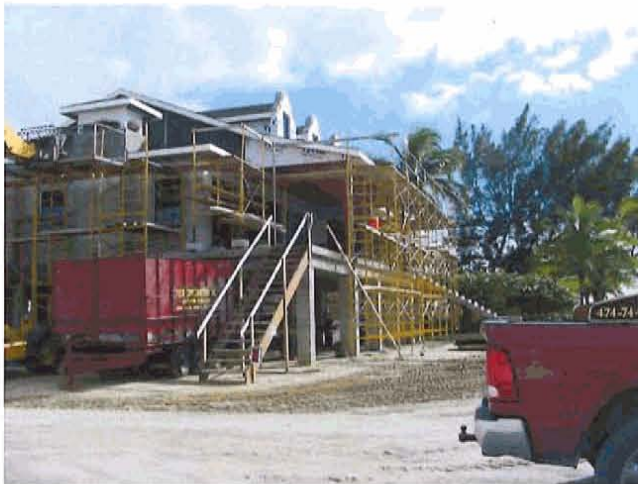
NW Corner at Banyan St and Beach Side Elevations
