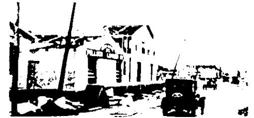
Pollock Lumber Company, started in 1923 in East Fort Myers (Board & Bartlett)
