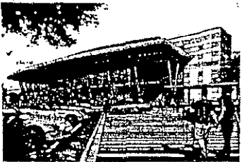
Orange Co. Convention Center W. Entrance Upgrade Orlando, Florida
