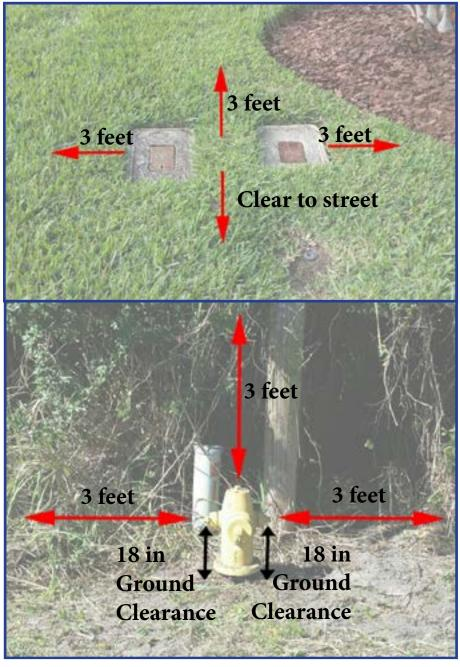
Clearance must be maintained around fire hydrants and meter boxes.
