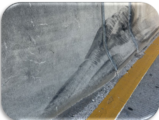
Figure 149: Typical Traffic Island Barrier Scrape
