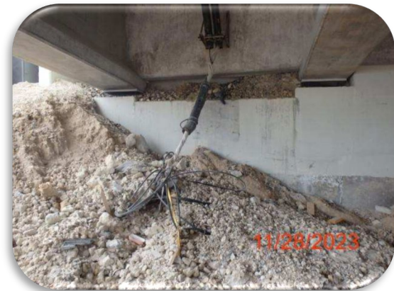
Figure 204: Sanibel Bridge, Structure A – Abutment Adjacent Junction Box Defects
