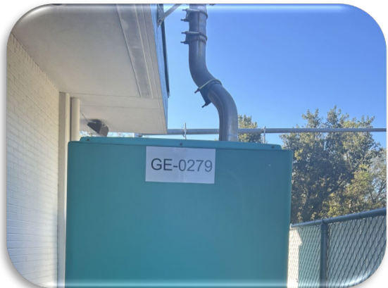
Figure 233: Generator Exhaust Pipe Extension
