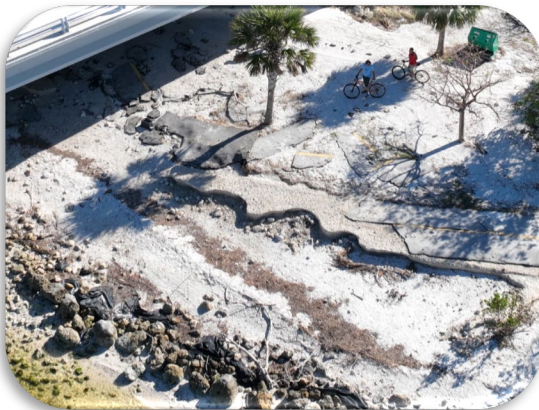
Figure 221: Sanibel Bridge, Structure C – Loss of Eastbound Approach Pedestrian Walkway
