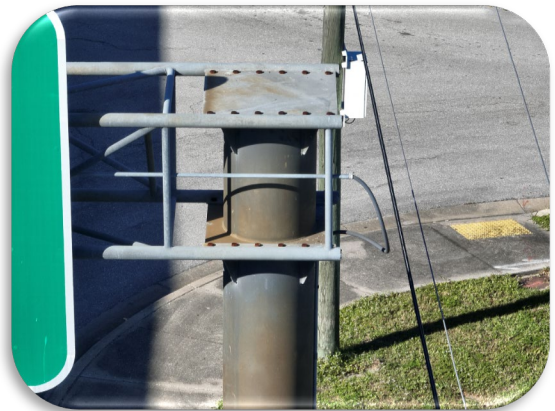
Figure 48: Cape Coral -WB OSS 0.6 Miles from Plaza - Loss of Galvanization on Upright
