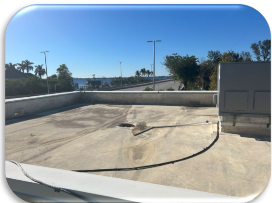
Figure 13: Resealed Roof Over Conference Room
