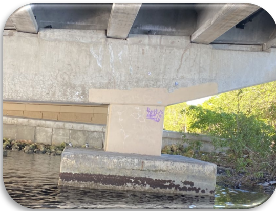
Figure 138: Midpoint Bridge – Pier Cap Cracking and Painted Graffiti
