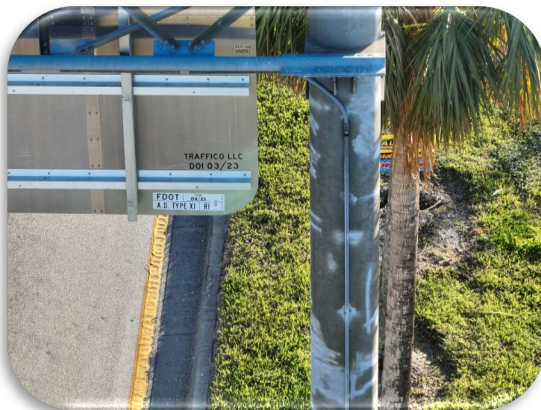
Figure 118: Midpoint - WB OSS 3.125 Miles from Plaza – Typical Galvanizing Spray Rehab
