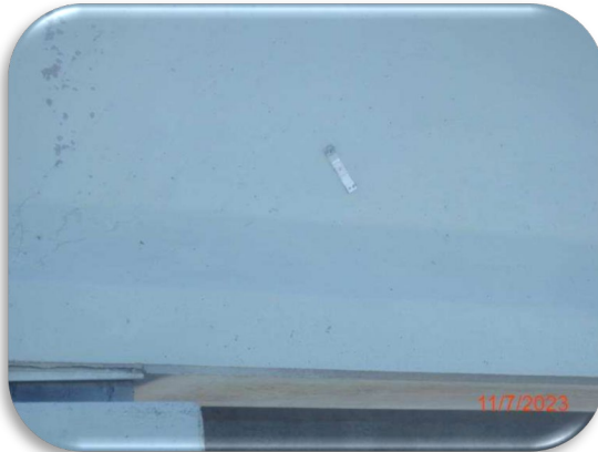
Figure 189: Sanibel Bridge – Typical Crack Width Monitor Gauge
