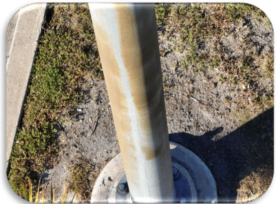
Figure 40: Cape Coral -WB OSS 1-1/4 Miles from Plaza - Loss of Galvanization on Upright
