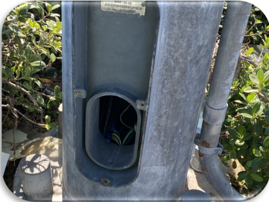
Figure 185: Sanibel - Signalization Structure 100-yards from Plaza – Missing Handhole Cover
