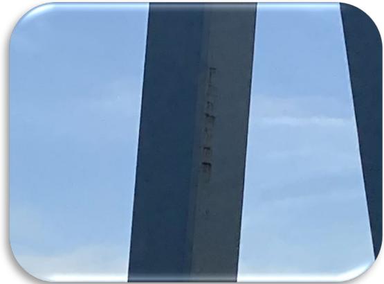
Figure 202: Sanibel Bridge, Structure A – Column Spalls with Exposed Reinforcement
