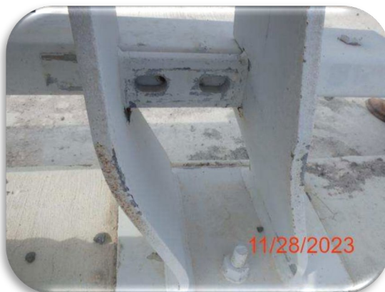
Figure 213: Sanibel Bridge, Structure B – Bent Bridge Rail Bracket
