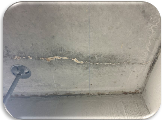
Figure 85: Concrete Ceiling Crack
