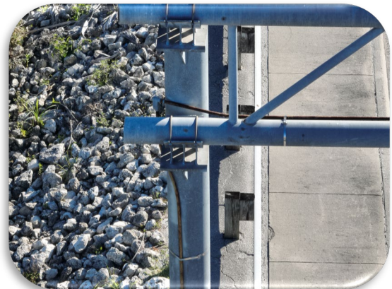
Figure 42: Cape Coral -WB OSS 1-1/4 Miles from Plaza – Electrical Conduit Corrosion
