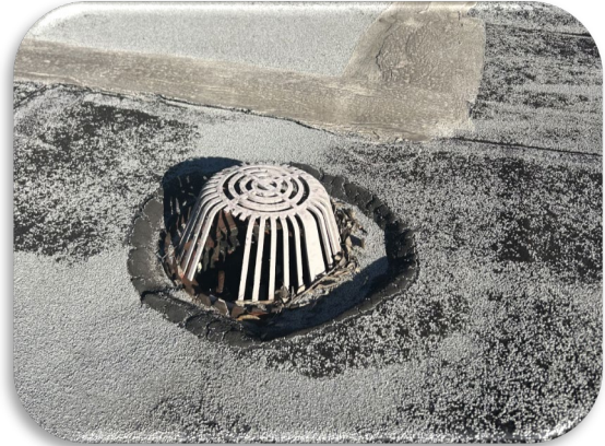
Figure 235: Typical Clear Roof Drainage Inlet
