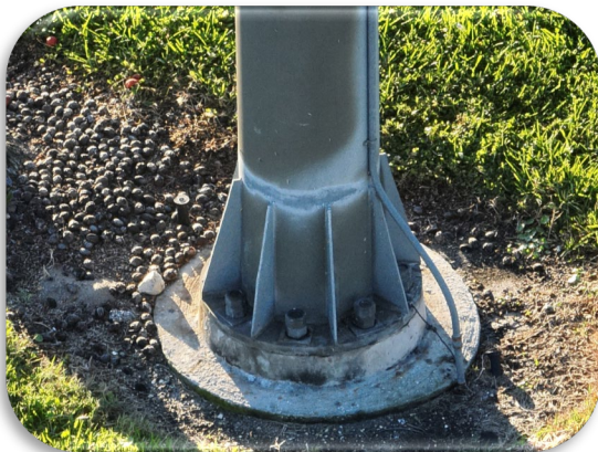
Figure 114: Midpoint - WB OSS 3 ¼ Miles from Plaza – Typical Galvanizing Spray Rehab
