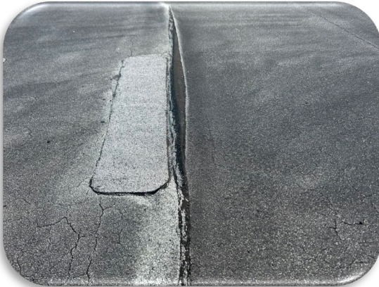
Figure 18: Toll Canopy Roof Covering Lifted at Seams
