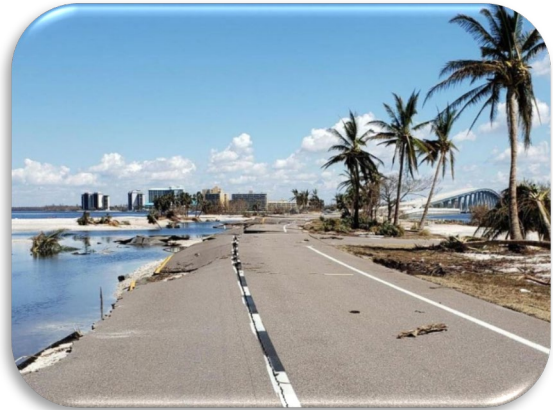
Figure 198: Sanibel Bridge – Hurricane Ian Damage
