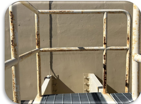
Figure 89: Toll Gantry Stairs Corrosion
