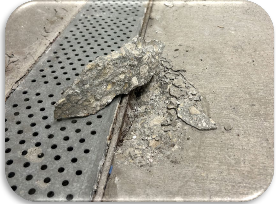
Figure 83: Concrete Spalling at Trench Drain Edge
