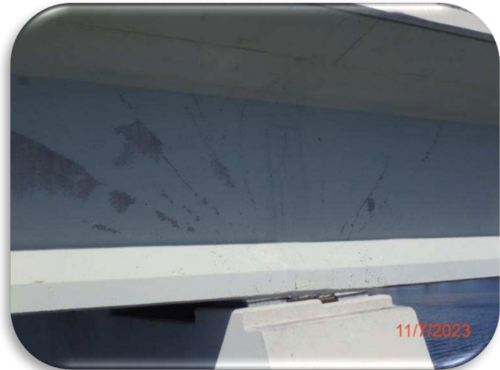
Figure 190: Sanibel Bridge – Typical Beam End Cracking
