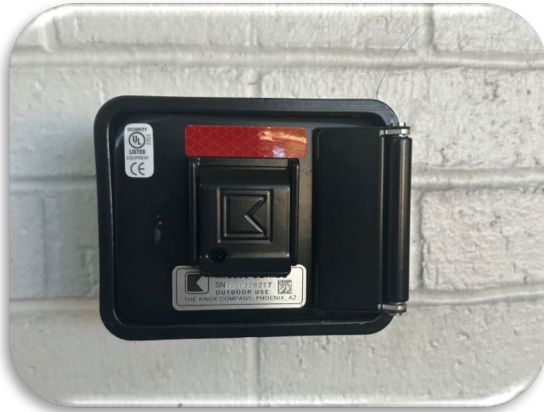
Figure 226: Emergency Service Lock Box
