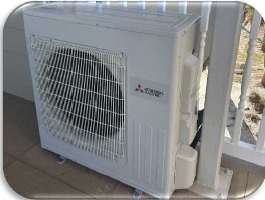
Figure 153: Typical New A/C Condensing Unit
