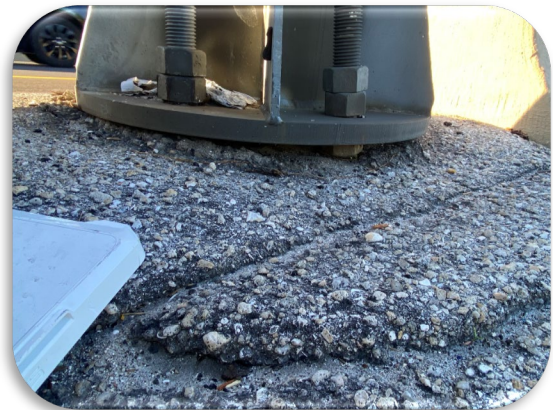
Figure 127: Midpoint - WB OSS 1 Mile from Plaza – Compromised Structural Grout Pad
