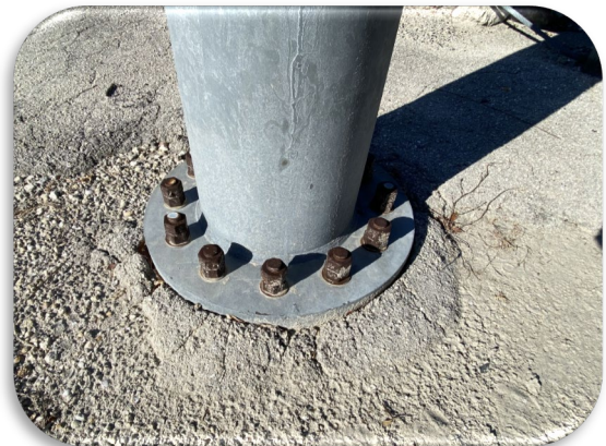
Figure 46: Cape Coral -WB OSS 1 Mile from Plaza – Upright Anchor Bolt Corrosion
