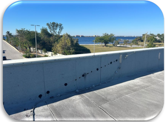
Figure 29: Toll Canopy Roof Lightning Rod System
