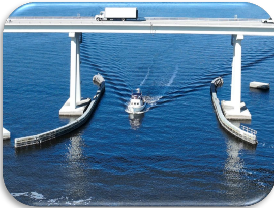
Figure 201: Sanibel Bridge, Structure A – General Fender System Layout
