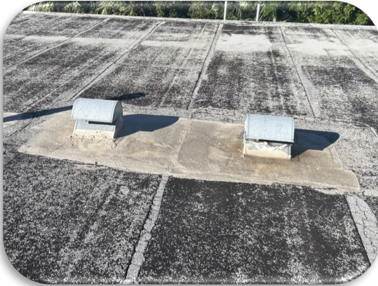
Figure 234: Typical Repaired Roof Patch Condition
