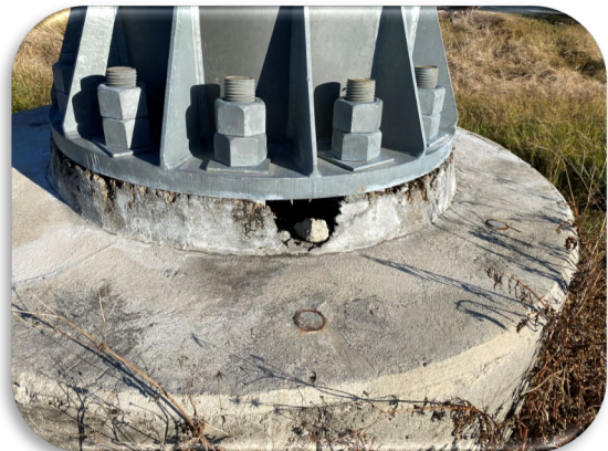
Figure 133: Midpoint - WB OSS ¼ Mile from Plaza – Compromised Structural Grout Pad
