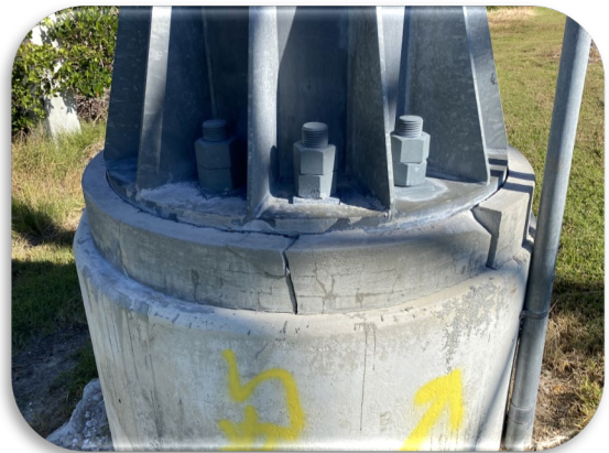
Figure 172: Sanibel - WB OSS 1 ½ Miles from Plaza - Structural Grout Pad Cracking
