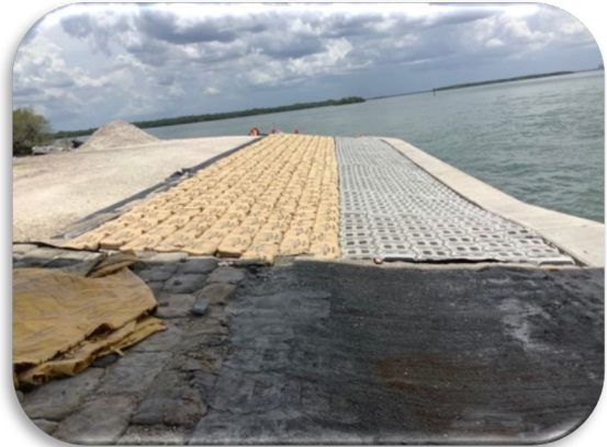
Figure 206: Sanibel Bridge, Structure A – Articulating Concrete Block Matting Installation
