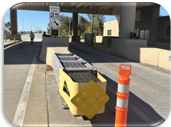
Figure 23: Impact Attenuator
