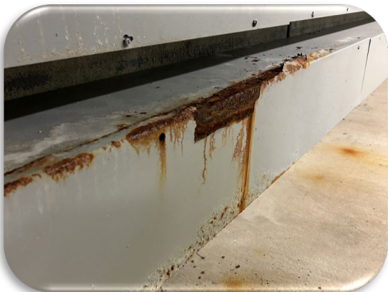
Figure 84: Metal Conduit Chase Corrosion
