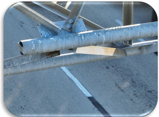
Figure 115: Midpoint - WB OSS 3 ¼ Miles from Plaza – Typical Truss Chord Loss of Galv. and Corrosion
