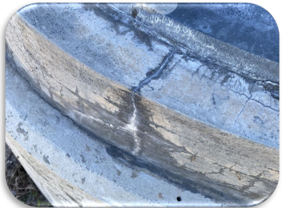
Figure 176: Sanibel - WB OSS 1 Mile from Plaza - Structural Grout Pad Cracking
