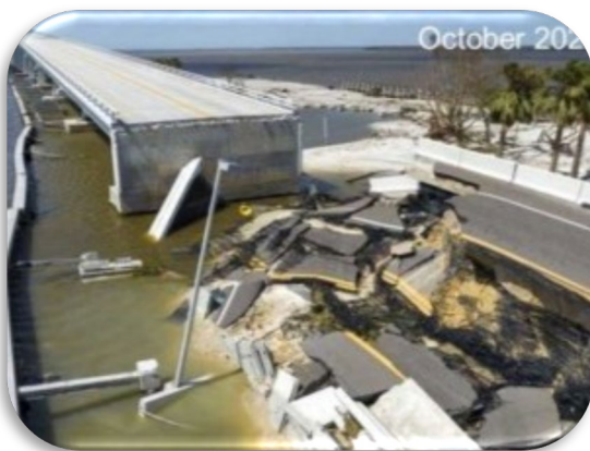
Figure 195: Sanibel Bridge – Hurricane Ian Damage
