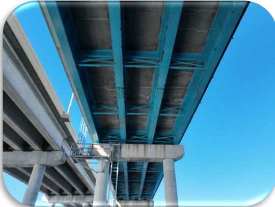
Figure 57: Cape Coral Bridge Westbound – Main Span Steel Girder Corrosion
