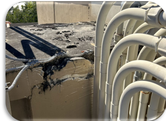
Figure 91: Toll Gantry – East Side Lightning Protection Anchorage Spalling
