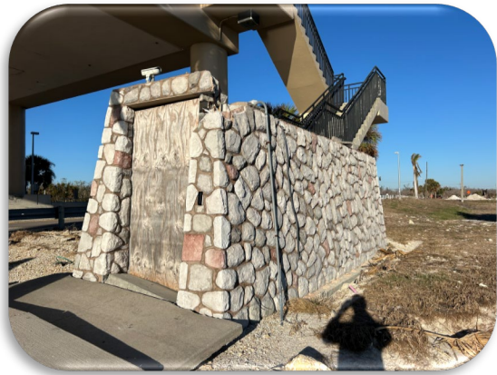
Figure 152: South Stairwell Instability
