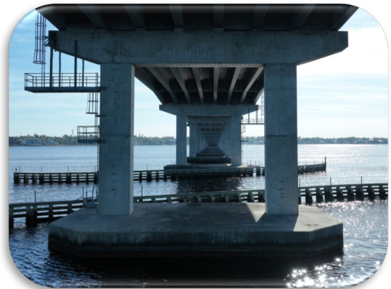
Figure 141: Midpoint Bridge– General Substructure Geometry at Main Span
