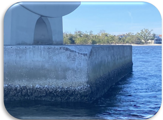
Figure 220: Sanibel Bridge, Structure C – Typically Footing Corner Spall
