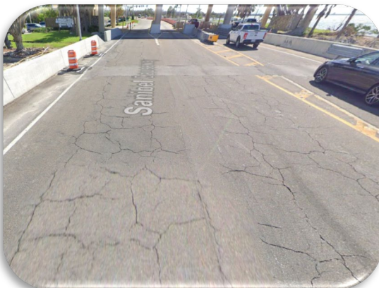
Figure 169: Representative Pavement Distress and Cracking Near Toll Plaza – August 2024
