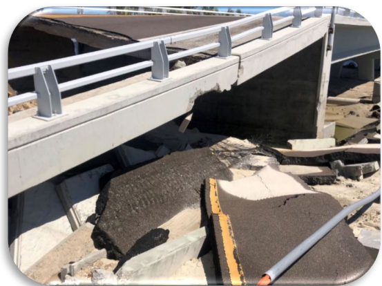
Figure 196: Sanibel Bridge – Hurricane Ian Damage
