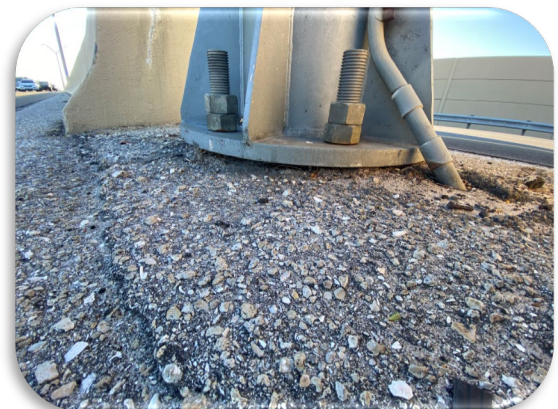
Figure 131: Midpoint - WB OSS ½ Mile from Plaza – Compromised Structural Grout Pad
