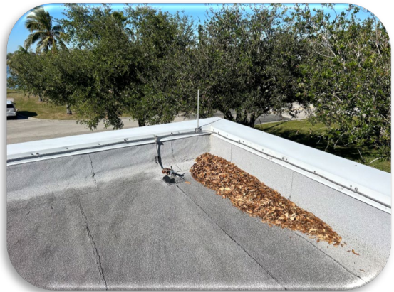
Figure 81: Administration Building Roof Vegetation
