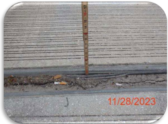
Figure 222: Sanibel Bridge, Structure C – Joint Strip Seal Pulled Out of Armor
