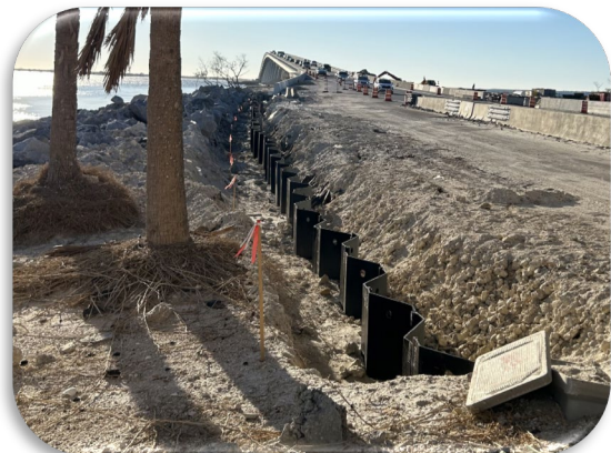
Figure 170: Active Seawall and Rubble Riprap Construction West of Toll Plaza
