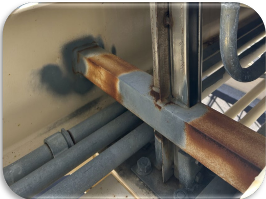
Figure 90: Toll Gantry – East Side Member Corrosion
