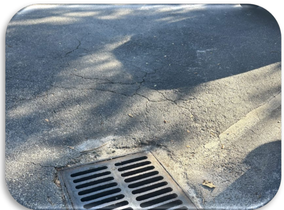
Figure 249: Typical Pavement Distress Around Drainage Inlet
