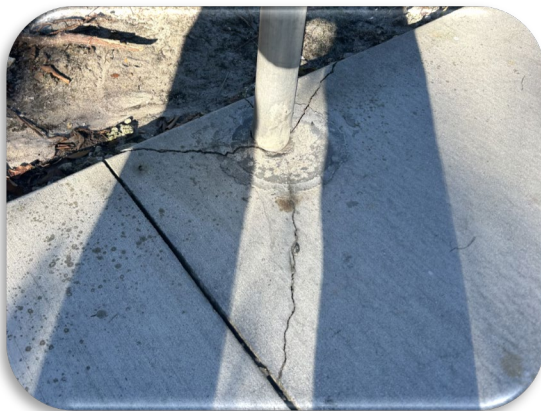
Figure 248: Concrete Sidewalk Spalling at Handrail
