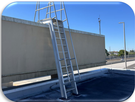
Figure 80: Toll Canopy Roof Access Ladder
