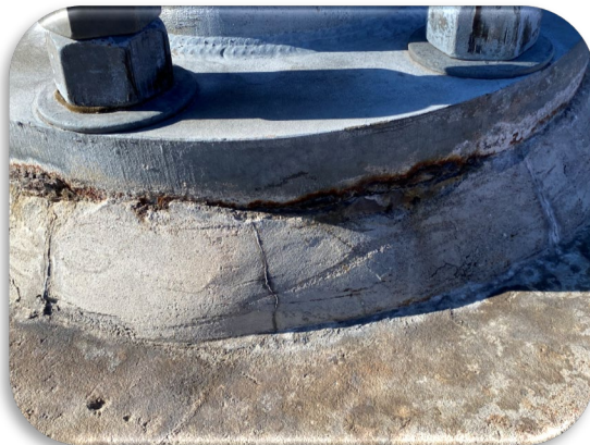
Figure 41: Cape Coral - WB OSS 1-1/4 Miles from Plaza – Baseplate Corrosion
