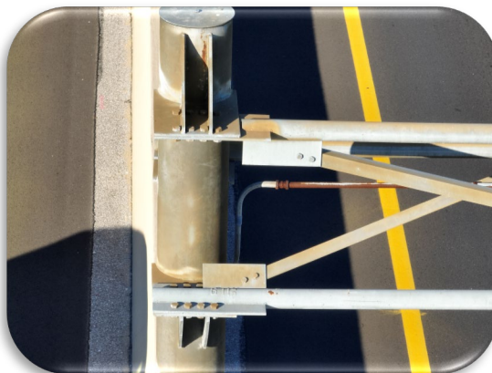
Figure 130: Midpoint - WB OSS ½ Mile from Plaza – Upright Surface Corrosion and Lighting Conduit Corrosion
