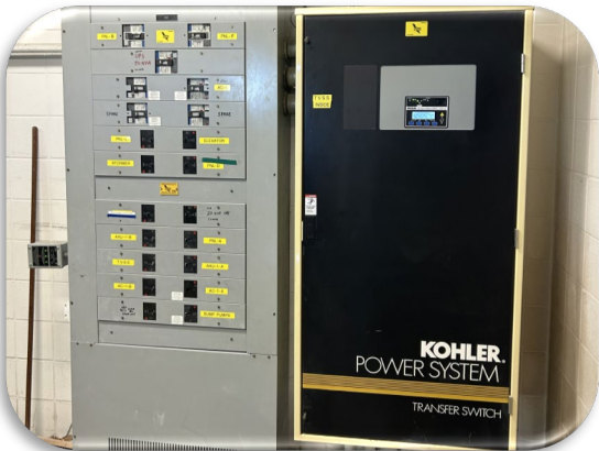
Figure 96: Standby Transfer Switch
