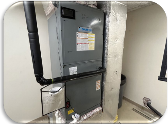
Figure 154: Typical New A/C Handling Unit
