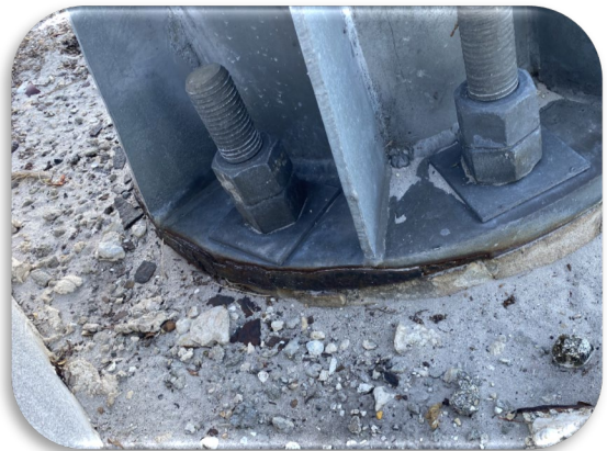
Figure 113: Midpoint – WB OSS 3 ¼ Miles from Plaza - Upright Baseplate Corrosion
