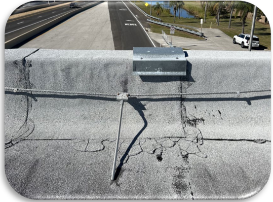
Figure 79: Typical Toll Canopy Roof Lightning Protection System Dismounted
