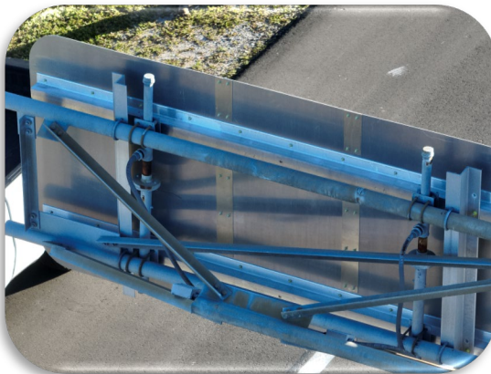
Figure 126: Midpoint - WB OSS 1 Mile from Plaza – Typical Lighting Conduit Corrosion
