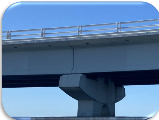
Figure 191: Sanibel Bridge – Typical Beam End Painting
