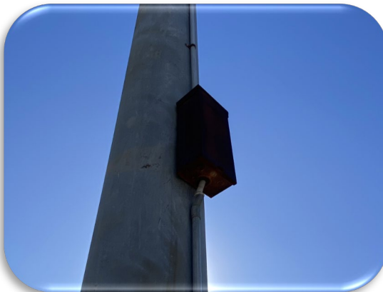
Figure 45: Cape Coral - WB OSS 1 Mile from Plaza – Electrical Panel Box Corrosion
