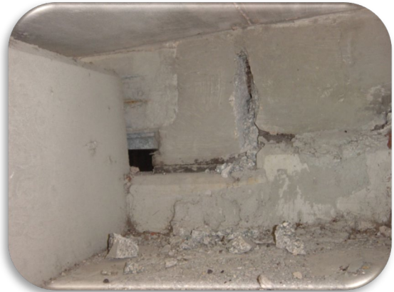
Figure 194: Sanibel Bridge – Typical Closure Pour Failure at Continuity Diaphragm
