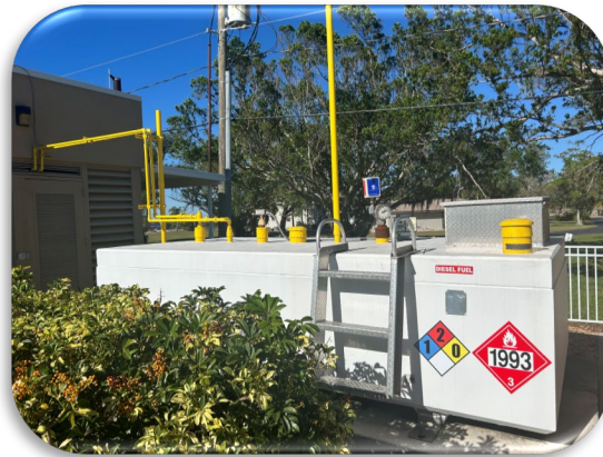
Figure 27: Recently Painted Diesel Fuel Tank
