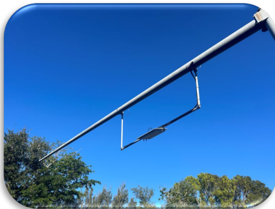
Figure 252: Miscellaneous Structure Arm & Transponder Equipment
