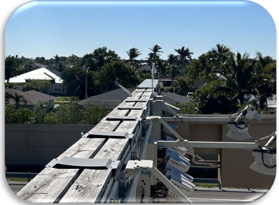
Figure 87: Toll Gantry – West Side Missing and Loose Flashing at Coping
