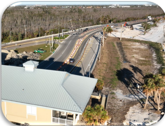
Figure 167: Typical MOT During FDOT Construction – East Side Approach to Toll Plaza
