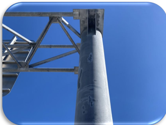
Figure 177: Sanibel - WB OSS 1 Mile from Plaza - Typical Galvanizing Spray Rehab
