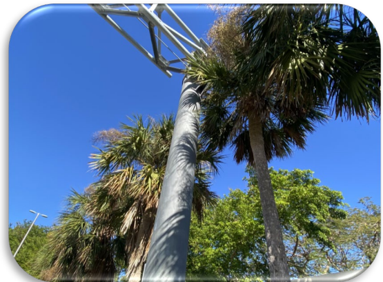
Figure 54: Cape Coral -WB OSS 100 Yards from Plaza – Vegetation Adjacent to Right Upright
