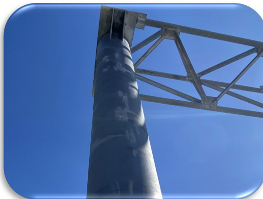
Figure 181: Sanibel - WB OSS ½ Mile from Plaza - Typical Galvanizing Spray Rehab
