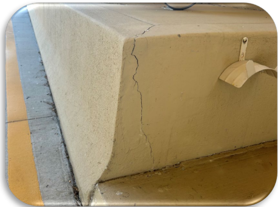
Figure 21: Moderate Cracks in Westbound Traffic Barrier Island
