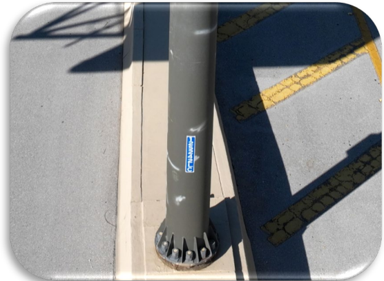
Figure 52: Cape Coral -WB OSS 1/4 Miles from Plaza – Galvanizing Paint Maintenance on Upright
