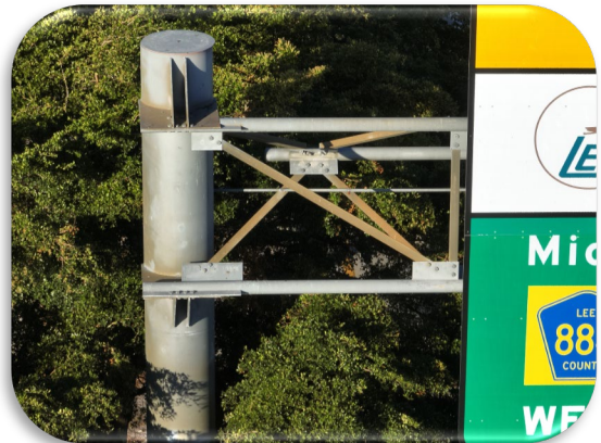
Figure 121: Midpoint – WB OSS 3 Miles from Plaza – Surface Corrosion on Truss Angles
