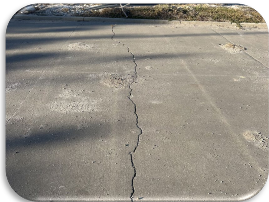
Figure 162: Concrete Pavement Crack
