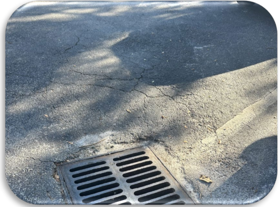
Figure 247: Typical Pavement Distress Around Drainage Inlet
