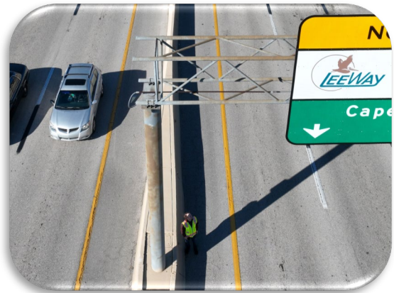
Figure 44: Cape Coral -WB OSS 1 Mile from Plaza - Loss of Galvanization on Upright and Truss Chords
