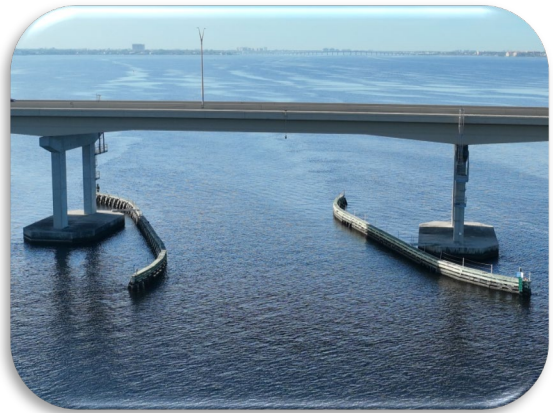
Figure 139: Midpoint Bridge – Fender System Alignment
