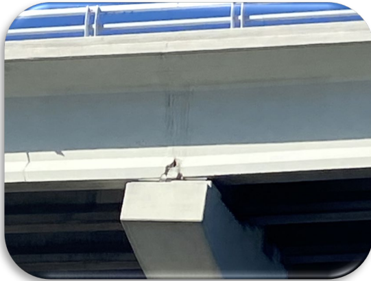
Figure 193: Sanibel Bridge – Typical End Diaphragm Spalling at Exterior Beam
