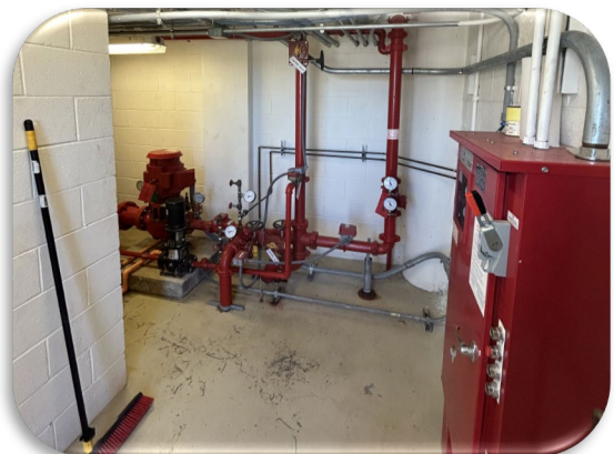
Figure 156: Fire Pump
