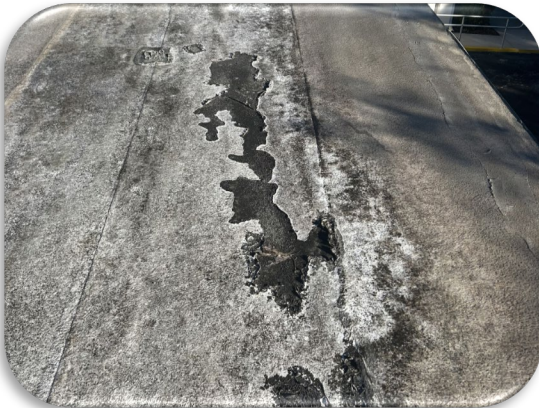
Figure 236: Deteriorating Roof Patching in Need of Repair
