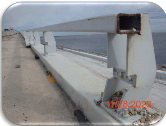
Figure 203: Sanibel Bridge, Structure A – Bridge Railing Impact Damage
