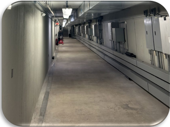
Figure 82: Access Tunnel with Lane Controller Cabinets
