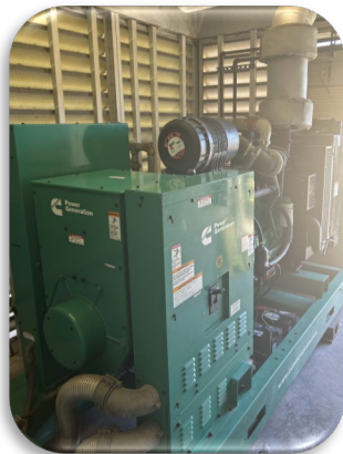
Figure 26: Standby Generator
