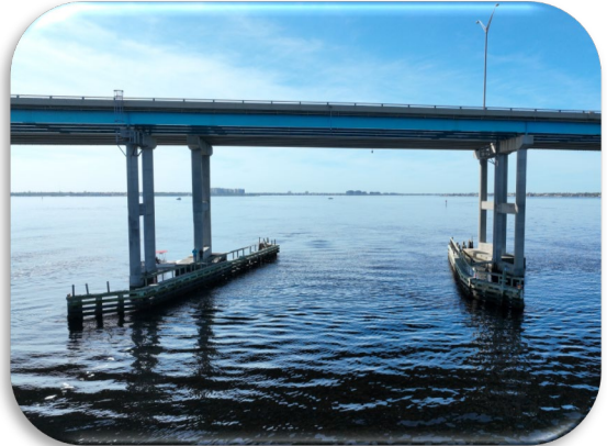
Figure 58: Cape Coral Bridge Westbound – Fender System Alignment and General Deterioration
