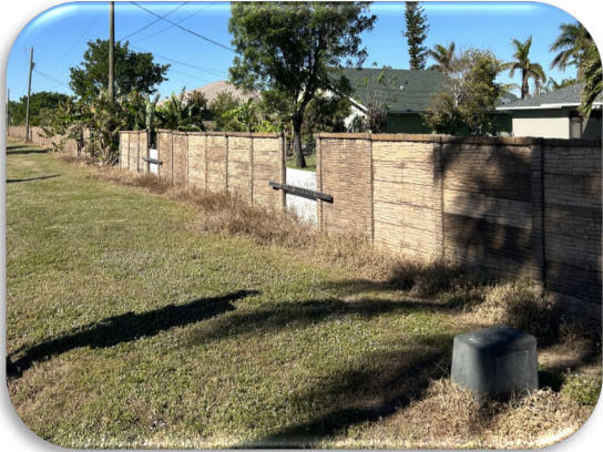
Figure 110: Northwest Solider Pile Noise Wall Damage
