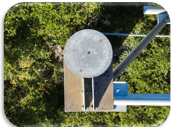
Figure 123: Midpoint - WB OSS 3 Miles from Plaza – Surface Corrosion on Upright Connection Plates
