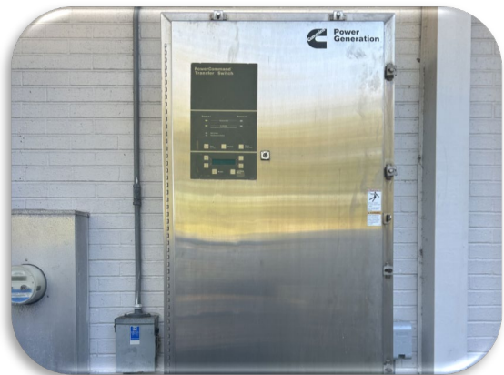
Figure 241: Generator Transfer Switch
