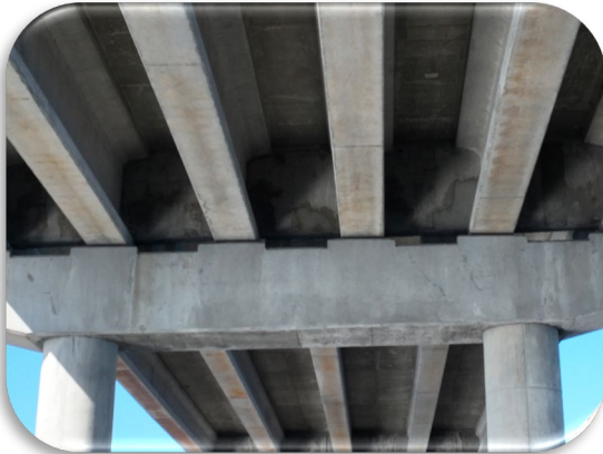
Figure 63: Cape Coral Bridge Eastbound – Typical Diaphragms and Pier Cap Cracking
