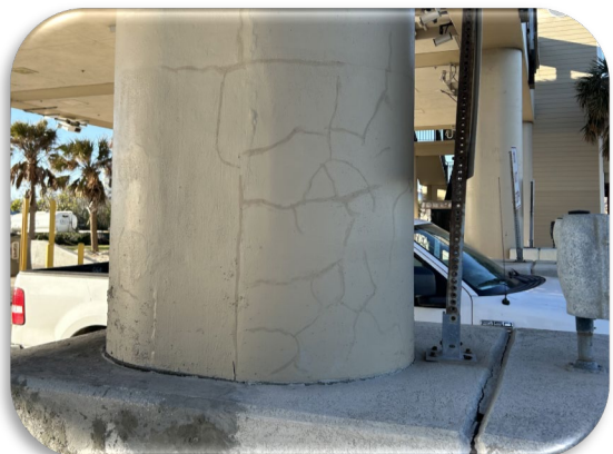
Figure 150: Toll Canopy Column Painted Cracks
