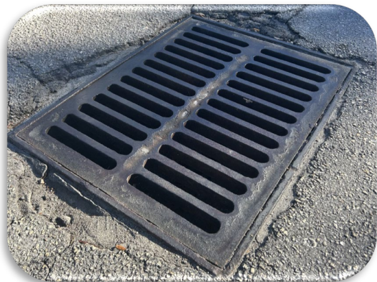
Figure 257: Typical Drainage Inlet Catch Basin
