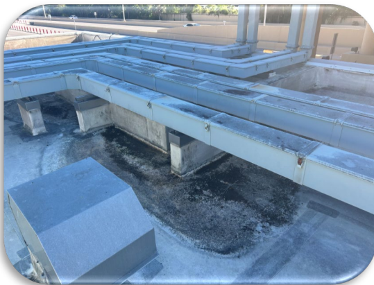
Figure 12: Administration Building Roof - Signs of Ponding
