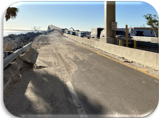
Figure 168: Eastbound Travel Lane Closed and Shifted During FDOT Construction
