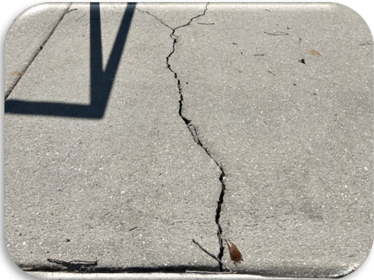
Figure 104: Typical Concrete Sidewalk Cracks
