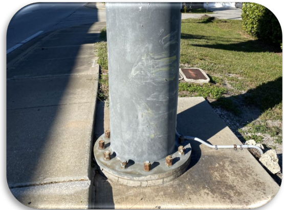
Figure 50: Cape Coral -WB OSS 0.6 Miles from Plaza – Impact Scrapes
