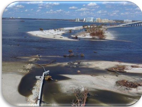
Figure 197: Sanibel Bridge – Hurricane Ian Damage
