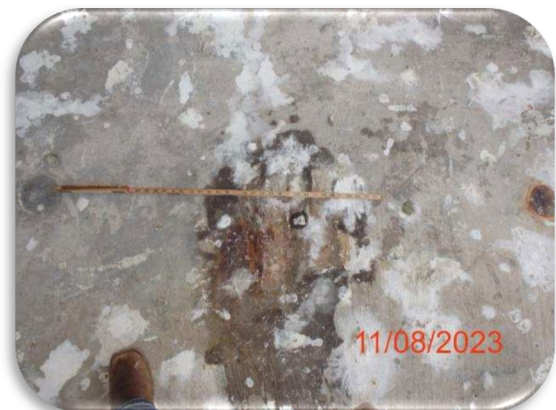
Figure 214: Sanibel Bridge, Structure B – Delaminated and Spalled Patch in Top of Pier Footing
