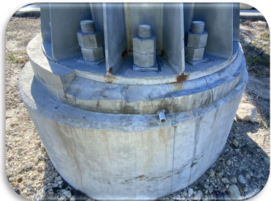
Figure 180: Sanibel - WB OSS ½ Mile from Plaza - Structural Grout Pad Cracking and Section Loss
