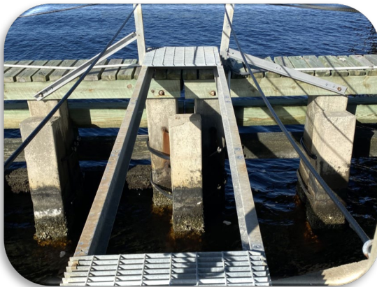
Figure 140: Midpoint Bridge – Fender System Access Ladder Missing Grate
