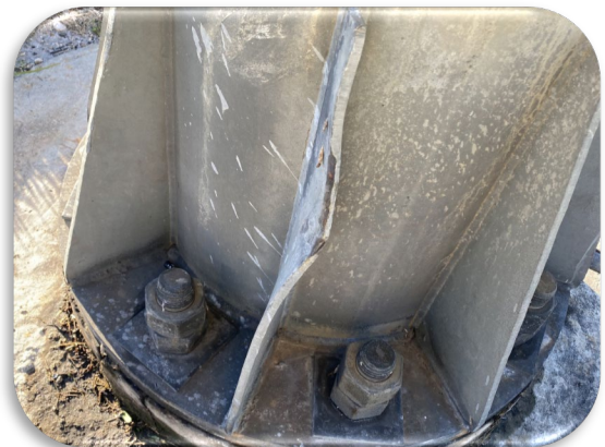
Figure 119: Midpoint - WB OSS 3.125 Miles from Plaza – Distorted Baseplate Vertical Stiffener
