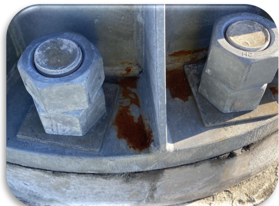
Figure 135: Midpoint - WB OSS 1/8 Mile from Plaza – Baseplate Corrosion
