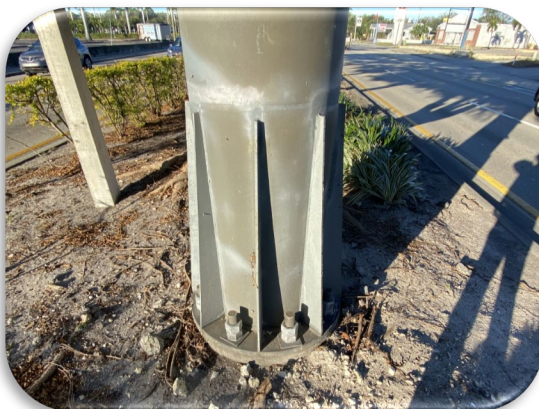
Figure 122: Midpoint - WB OSS 3 Miles from Plaza – Typical Galvanizing Spray Rehab
