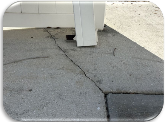
Figure 105: Typical Concrete Sidewalk Cracks at Reentrant Corners
