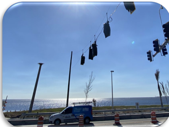
Figure 187: Sanibel - Signalization Structure 100-yards from Plaza – Temporary Signalization
