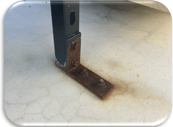
Figure 158: Fuel Storage Tank Support Hardware
