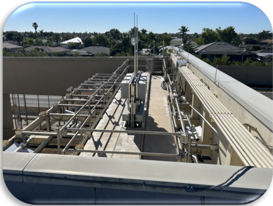
Figure 70: Open Road Tolling Equipment Gantry Structure Above Eastbound Lanes Five and Six
