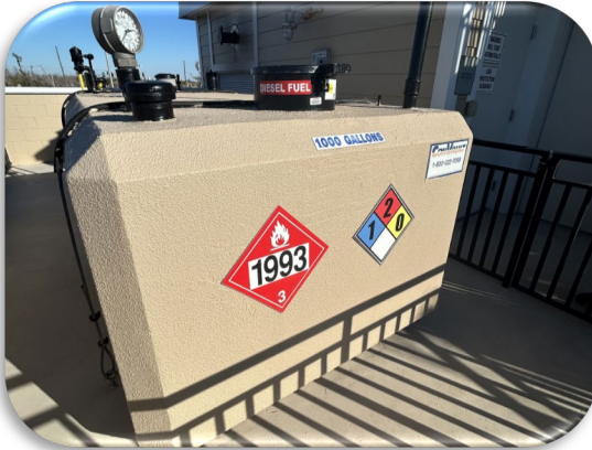
Figure 157: Fuel Storage Tank
