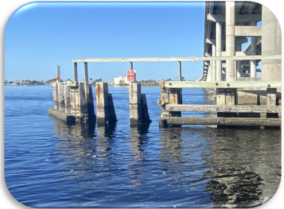
Figure 64: Cape Coral Bridge Eastbound – General Fender System Deterioration
