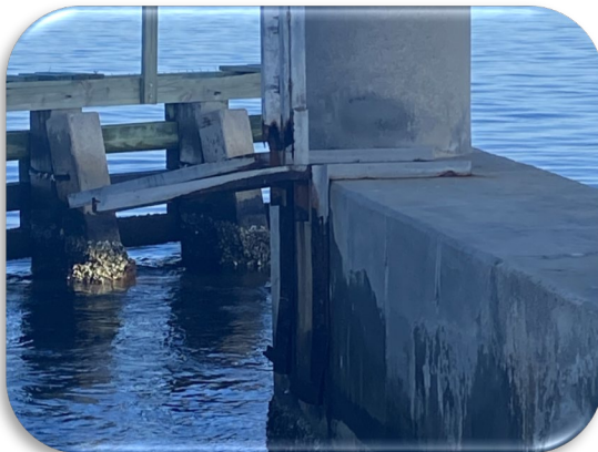
Figure 59: Cape Coral Bridge Westbound – Fender System Access Ladder Corrosion
