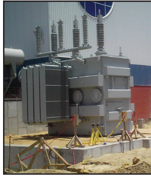
Generator Step-Up Transformer, purchased from General Electric
