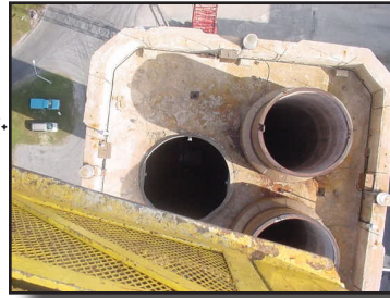
A look at the three flue pipes 275 feet above ground
