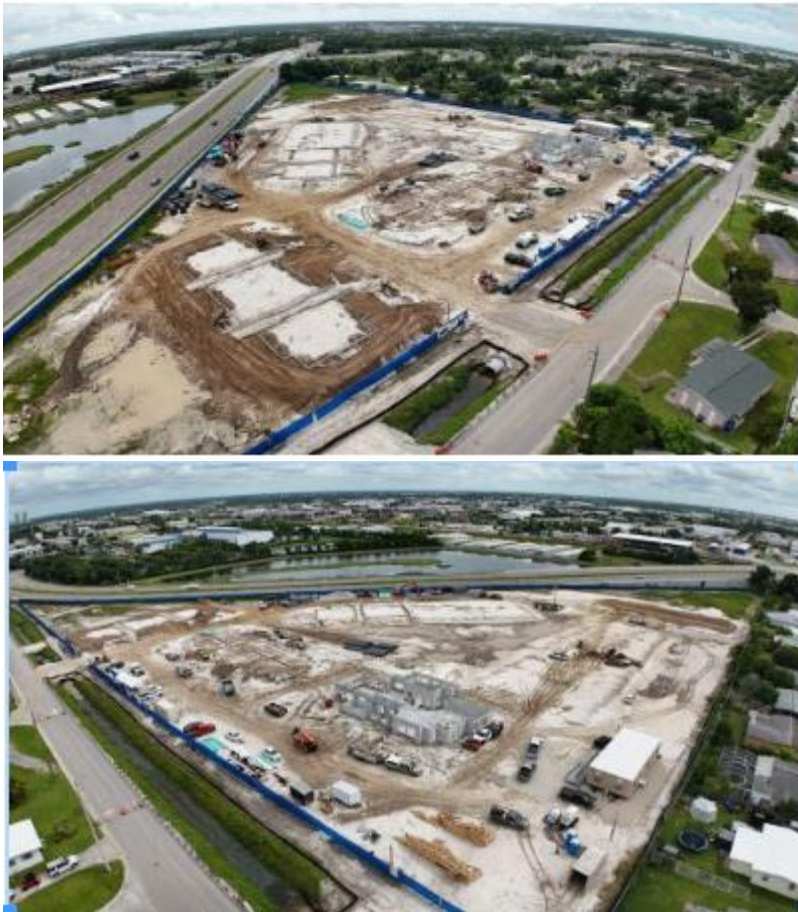
Figure 13. Aerial view of site work progress.
