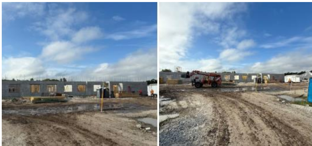
Figure 11. Oak Park construction progress.
