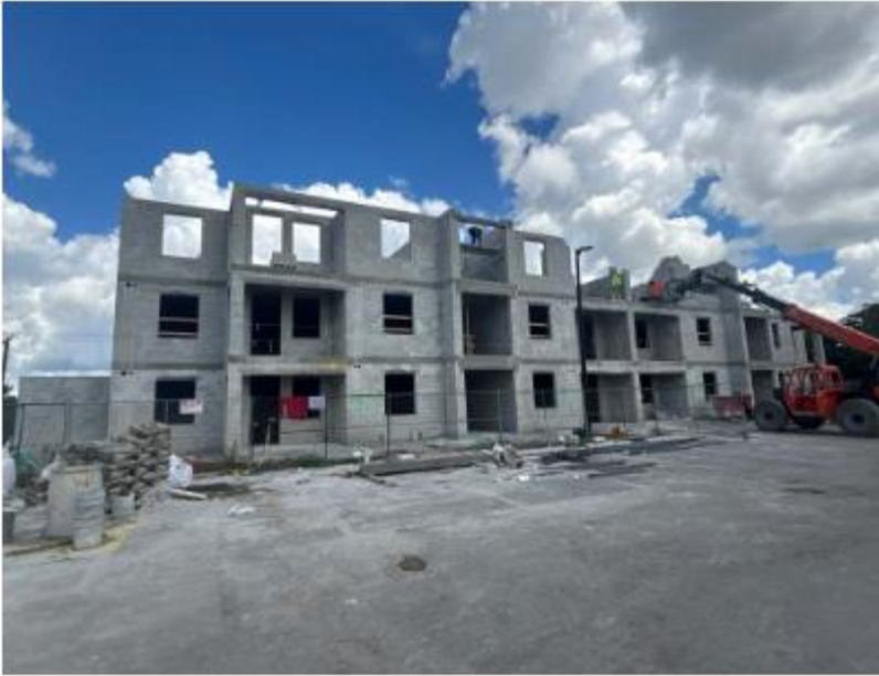
Figure 9. St Peter Claver Housing under construction
