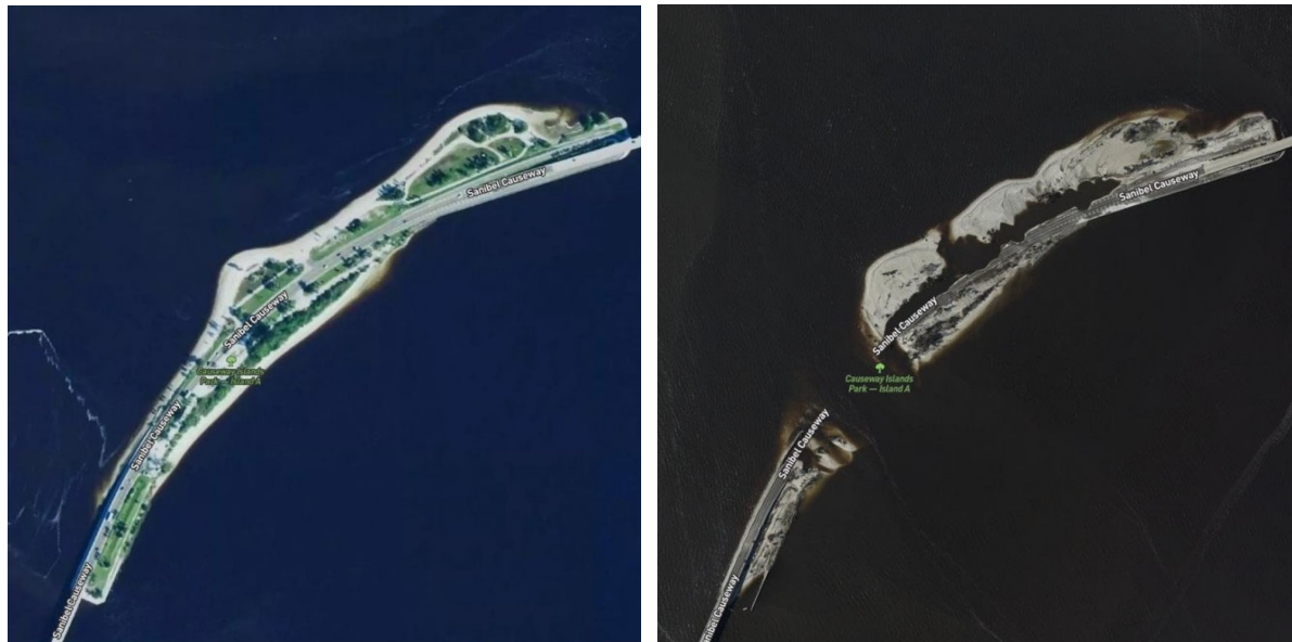
Figure 33 - Before and after imagery of a portion of the Sanibel Causeway, showing the damage of Hurricane Ian 124
