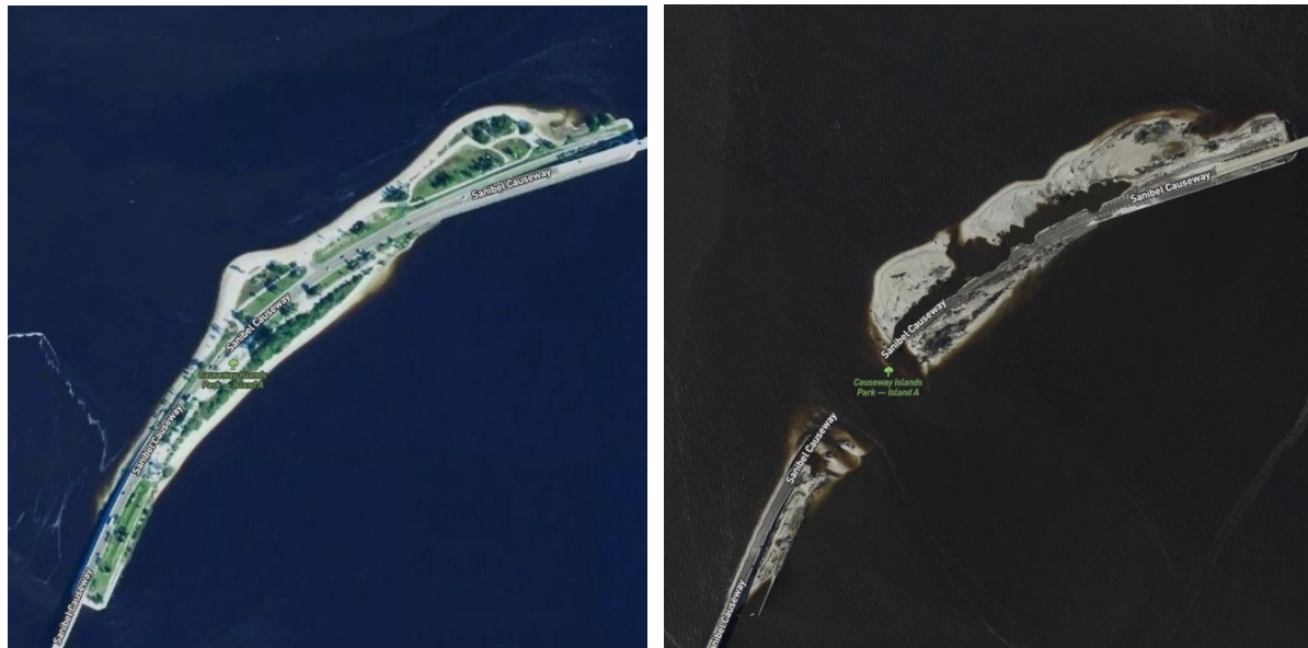
Figure 33 - Before and after imagery of a portion of the Sanibel Causeway, showing the damage of Hurricane Ian 124
