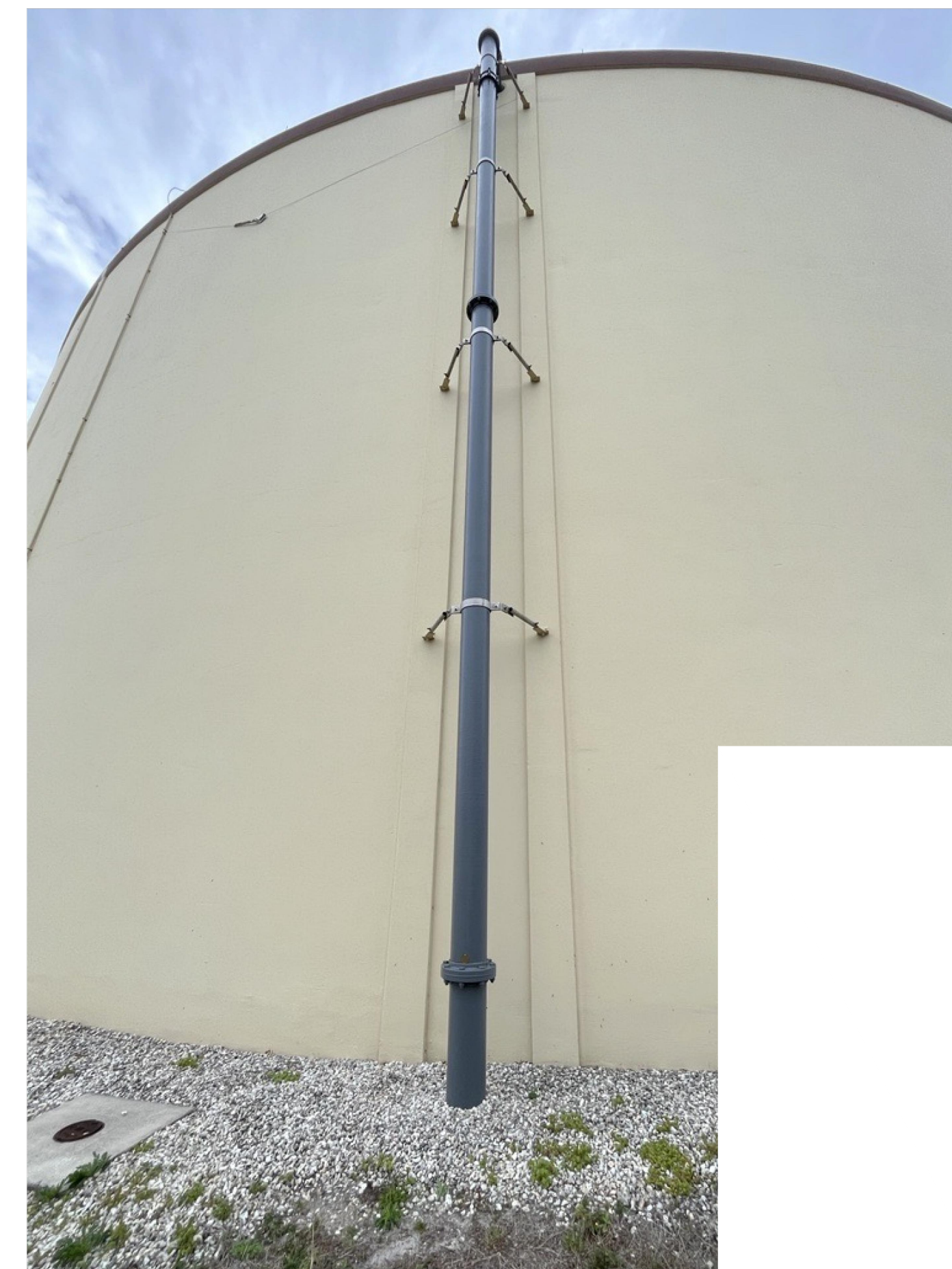
A STORAGE TANK OVERFLOW C-101 NO SCALE
