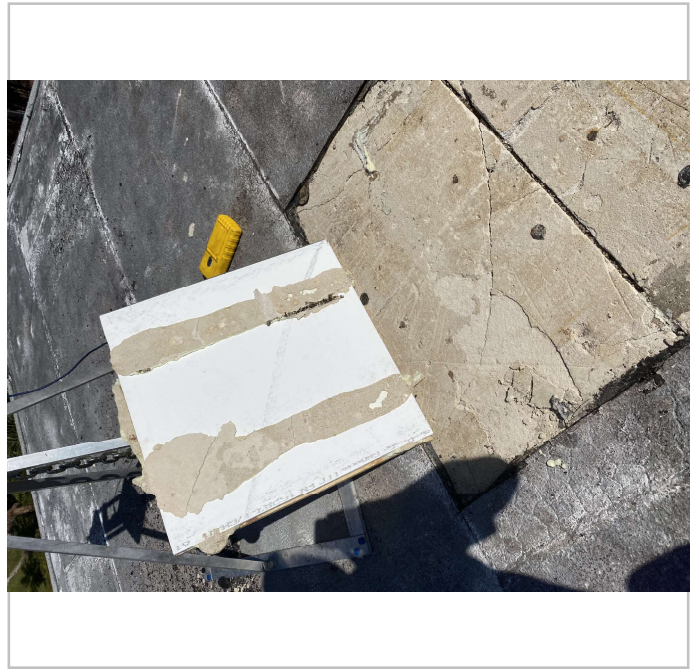
SUBSTRATE FAILURE
