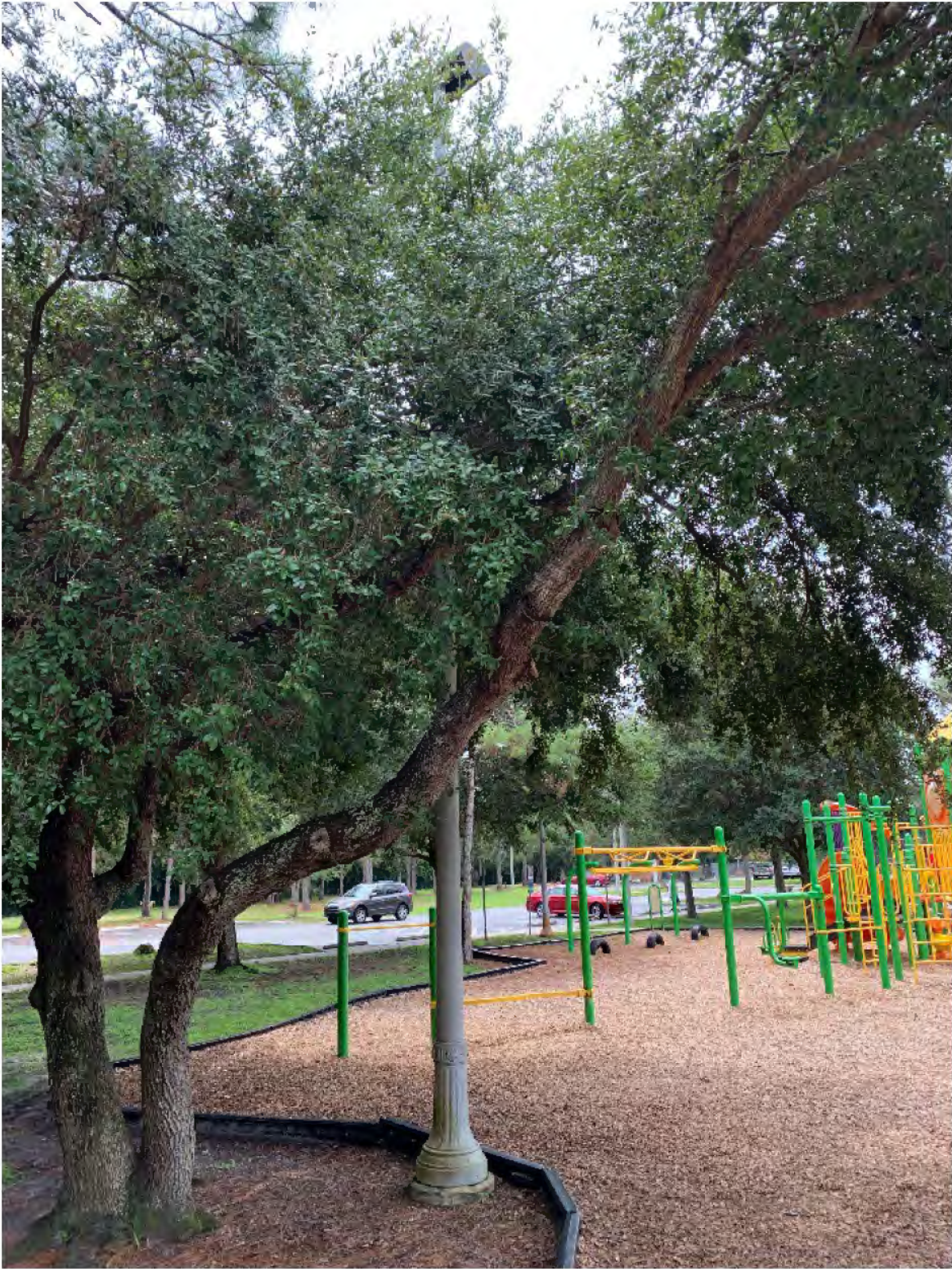
Figure 9. Northeast tree and light pole location (looking southeast)
