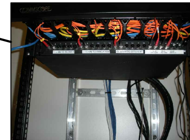
FIBER PATCH PANEL NO SCALE
