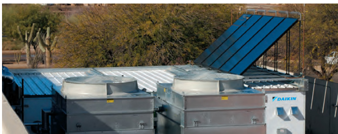
The Modular Central Plant includes solar panels used to heat domestic water, further increasing energy costs savings.
