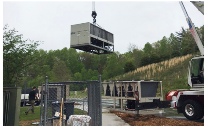
The existing chiller is removed to make way for a new Daikin Trailblazer air-cooled chiller that could save $48,000 in energy costs over seven years.
