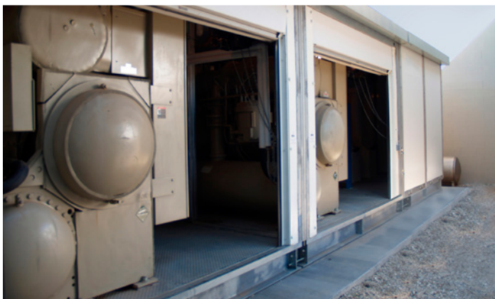
The Modular Central Plant at Chaparral High School features two energy efficient, 475-ton Daikin centrifugal chillers.
