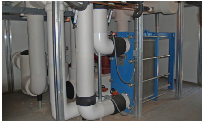
The Modular Central Plant at the school includes a plate-and-frame heat exchanger with secondary pumping.
