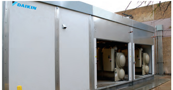
Two 300-ton Daikin Magnitude chillers and cooling towers replaced Pima's outdated chilled water central plant.
