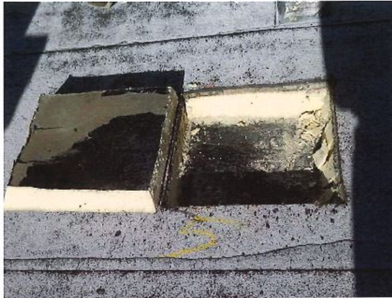
Photo 13 – Other test cuts revealed approximately 35% asphalt adhesion on the isocyanurate facer. We did not encounter full adhesion at any test cuts taken during this site visit.
