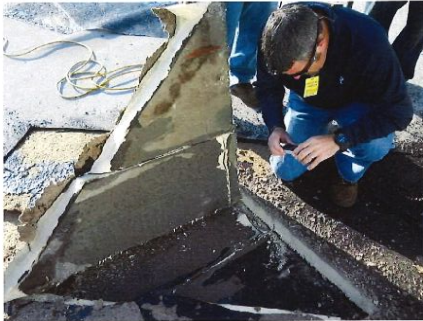
Photo 7 – Upon lifting of the isocyanurate insulation, we observed the bottom facer to be in tact with no evidence of adhered asphalt. This observation is significant because the absence of asphalt on this facer indicates a lack of adhesion to the substrate. Also note the moisture present on the facer. As previously indicated, we believe this moisture contamination is a result of the membrane split.
