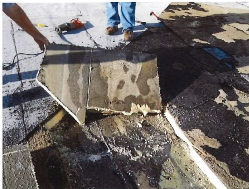
Photo 8 – Additional view of undamaged isocyanurate facer due to inadequate asphalt adhesion.
