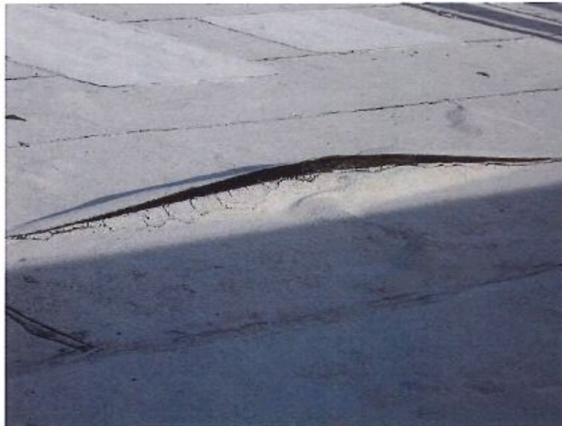
Photo 10 – Close up view of membrane blister
