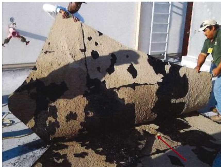
Photo 4 – View of fiberglass felts being peeled off the perlite coverboard. Note the split in the underlying isocyanurate insulation (indicated by arrow).
