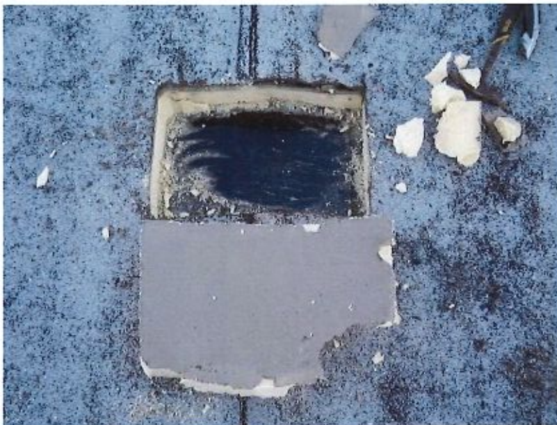
Photo 12 – Due to the inadequate adhesion observed on the southeast corner of the building (Photos 2 through 7), test cuts at blister locations were extended to the deck in an effort to determine the degree of adhesion at these locations. As is evident in this photograph, areas completely void of asphalt were encountered.
