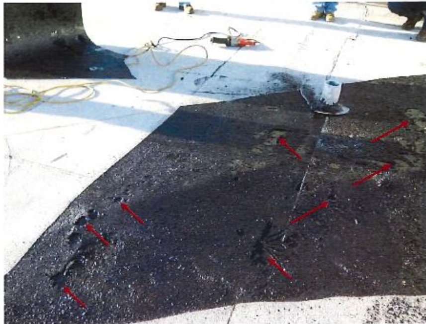
Photo 3 – View of cap sheet peeled away at location of damage observed in Photo 2. Note the voids present (highlighted by arrows) between the fiberglass felts and the cap sheet. These voids contain air which expands and contracts with temperature changes resulting in the formation and growth of blisters.
