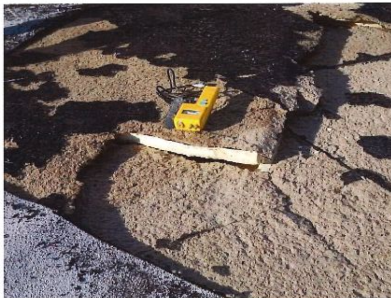
Photo 6 – Close-up view of the split isocyanurate insulation and perlite coverboard.
