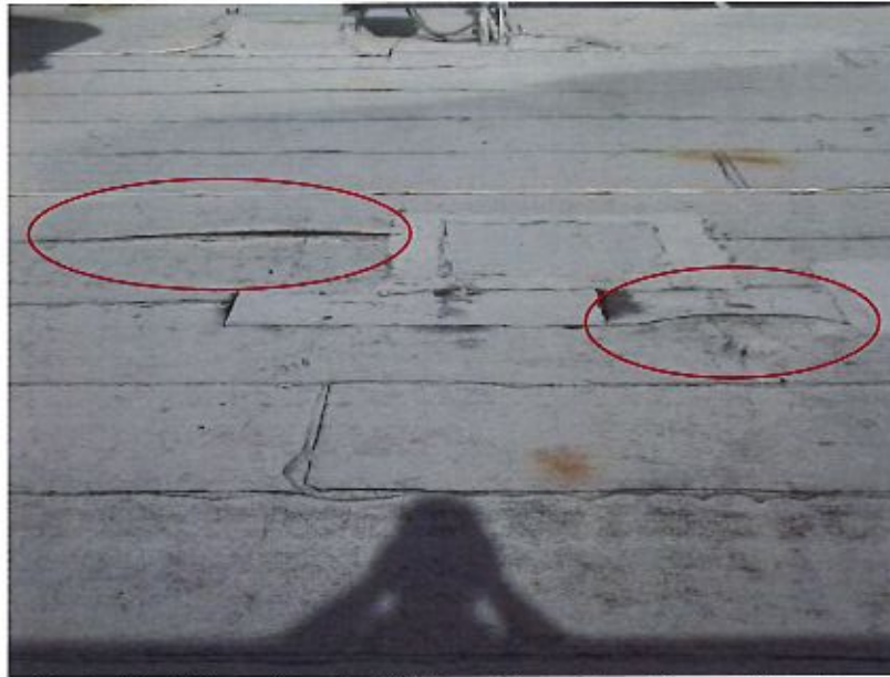
Photo 9 – View of typical blisters throughout the roof system.
