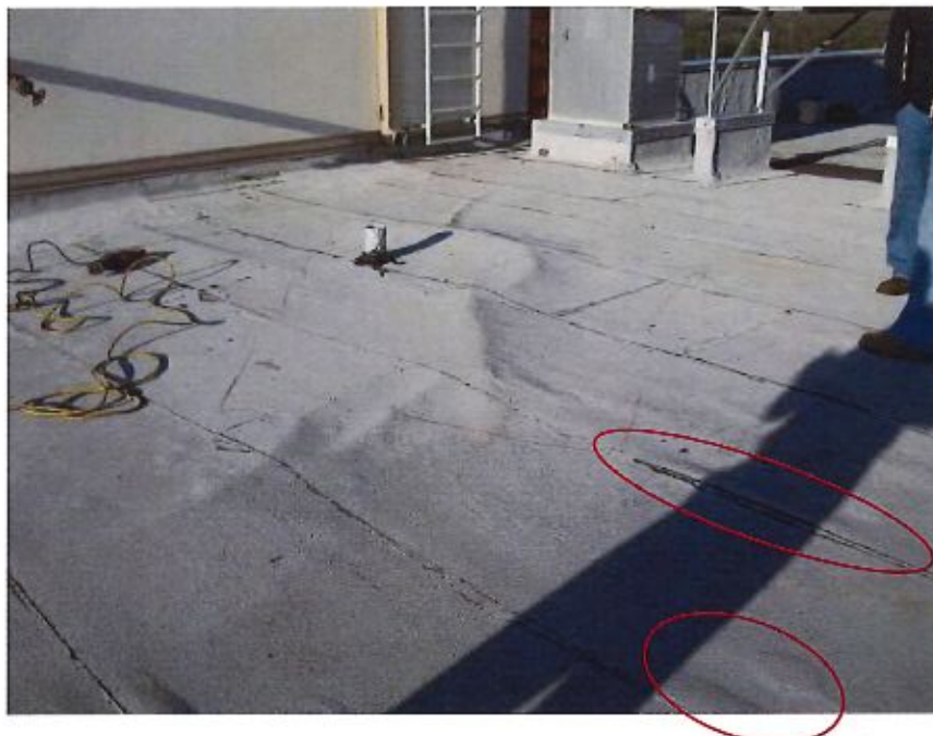
Photo 2 – Overview of area of displaced insulation resulting in roof membrane damage. Additionally, note the formation of blisters illustrated in red. These blisters are widespread throughout the entire roofing system.
