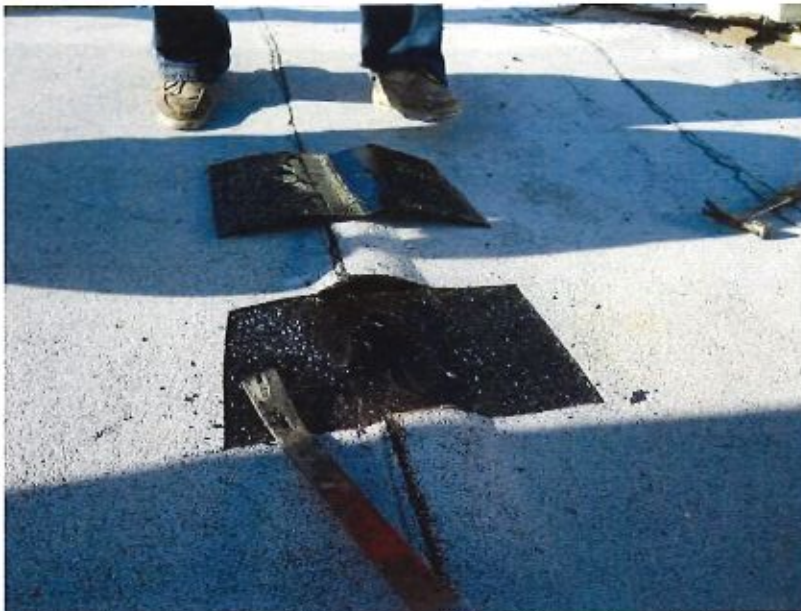
Photo 11 – Test cuts taken across the blister reveal the failure plane between the cap sheet and the upper fiberglass ply. This condition is consistent at all locations cut. Membrane samples were collected, labeled and submitted for laboratory analysis (results of analysis included at the end of this report).
