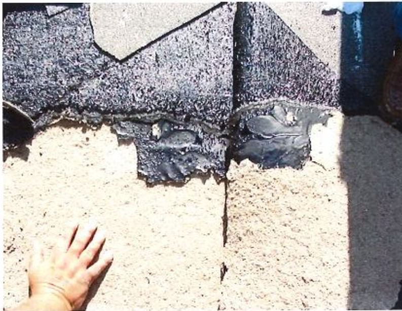
Photo 16 – Of the 5 negative pressure tests performed, only one test did not achieve an “apparent passing” result. The failure occurred near the location of the damaged roof system in the southeast corner of the facility. A test cut at this location revealed the presence of saturated insulation most likely resulting from the damaged roofing membrane. See the following section for a discussion regarding the “apparent passing” of the remaining tests.
