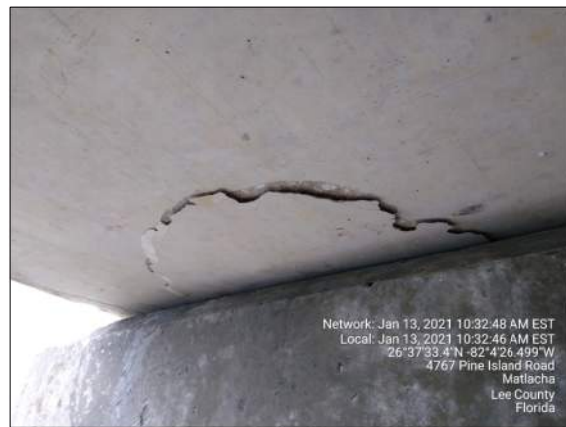
SPAN 1 - BENT 2 - BEAM 9
