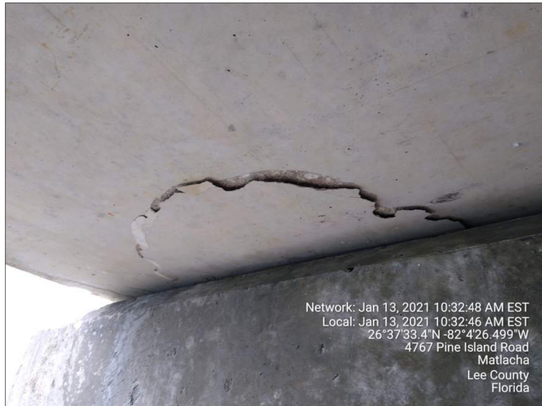
PHOTO SHOWING TYPICAL AREA FOR SPALL REPAIR
