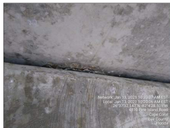
SPAN 2 - BENT 3 - BEAM 5
