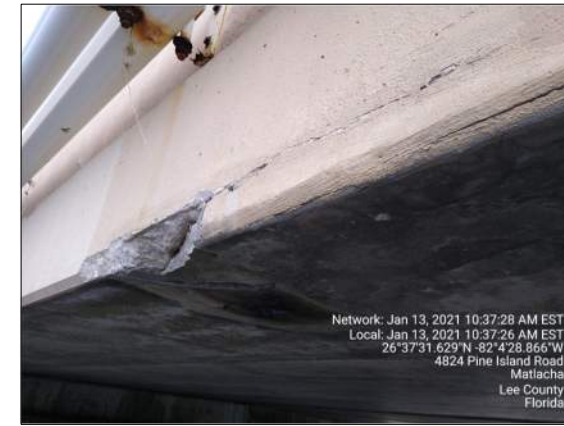
SPAN 1 - BENT 2 - BEAM 1
