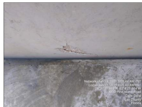
SPAN 7 - BENT 8 - BEAM 9
