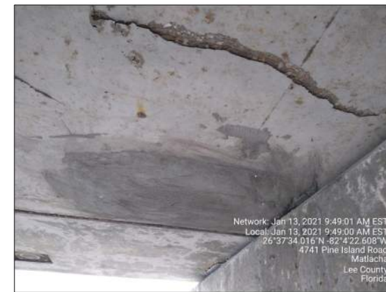
SPAN 4 - BENT 5 - BEAM 8
