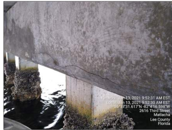
SPAN 4 - BENT 5 - BEAM 4
