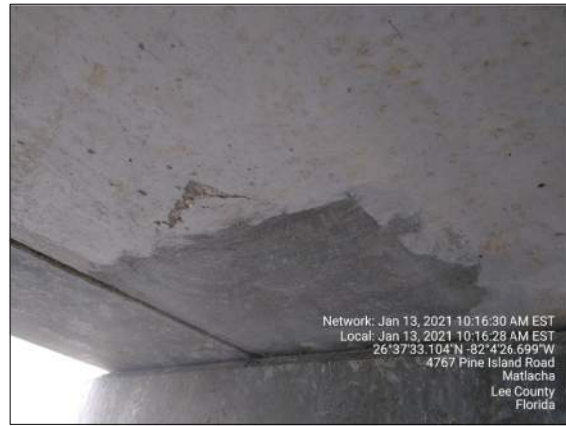
SPAN 2 - BENT 3 - BEAM 8
