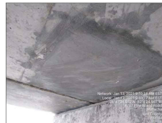
SPAN 4 - BENT 4 - BEAM 8
