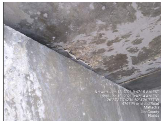
SPAN 4 - BENT 5 - BEAM 9
