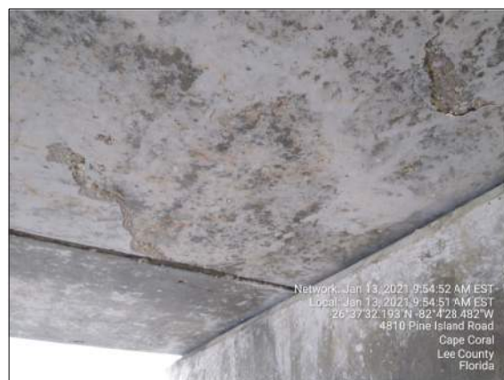
SPAN 4 - BENT 4 - BEAM 2
