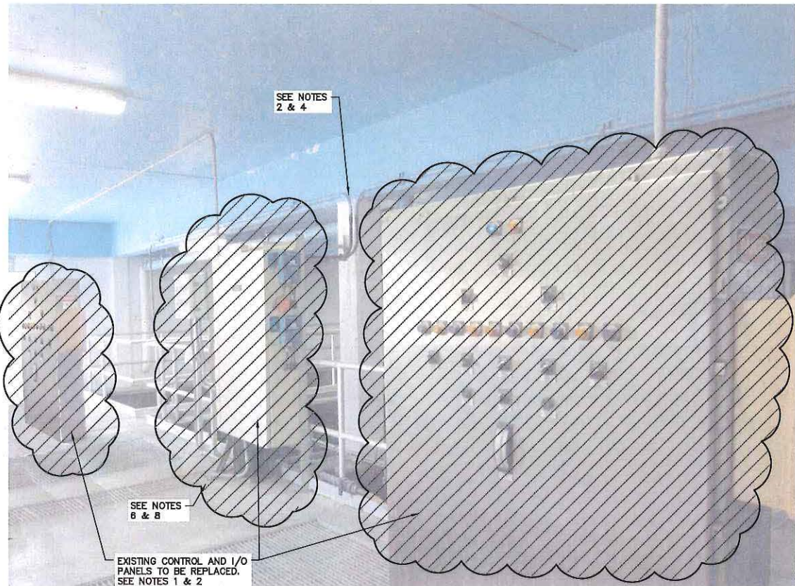
PHOTO 1A / E6 E3 EXISTING FILTER CONTROL PANELS SCALE: NTS AND I/O TERMINAL CABINET
