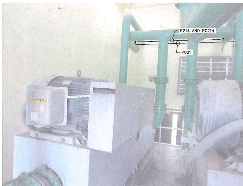
PHOTO 6 ELECTRICAL ROOM PARTIAL LAYOUT SCALE: NTS
