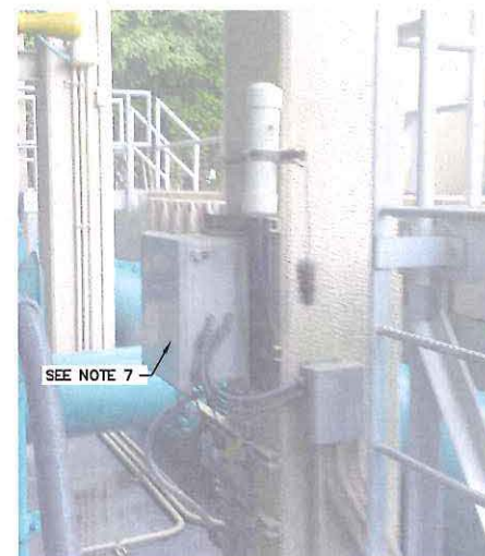
PHOTO 3 / E4 E3 EXISTING CHLORINE ANALYZER SCALE: NTS
