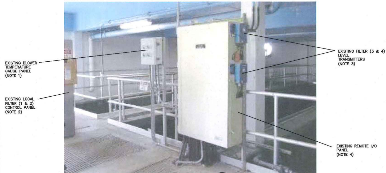
△ FIGURE 1: EXISTING FILTER REMOTE I/O PANEL
