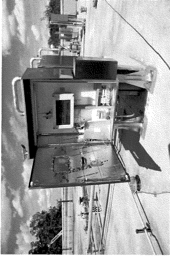
CITY OF TAMPA DAVID L. TIPPIN WTF 316 STAINLESS STEEL ENCLOSURE, SUNSHIELD, STANCHIONS TYPICAL CP FOR OZONE SYSTEM
