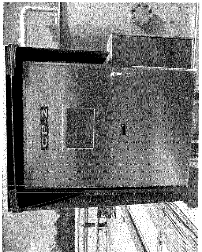
CITY OF TAMPA DAVID L. TIPPIN WTF 316 STAINLESS STEEL ENCLOSURE, SUNSHIELD, STANCHIONS TYPICAL CP FOR OZONE SYSTEM
