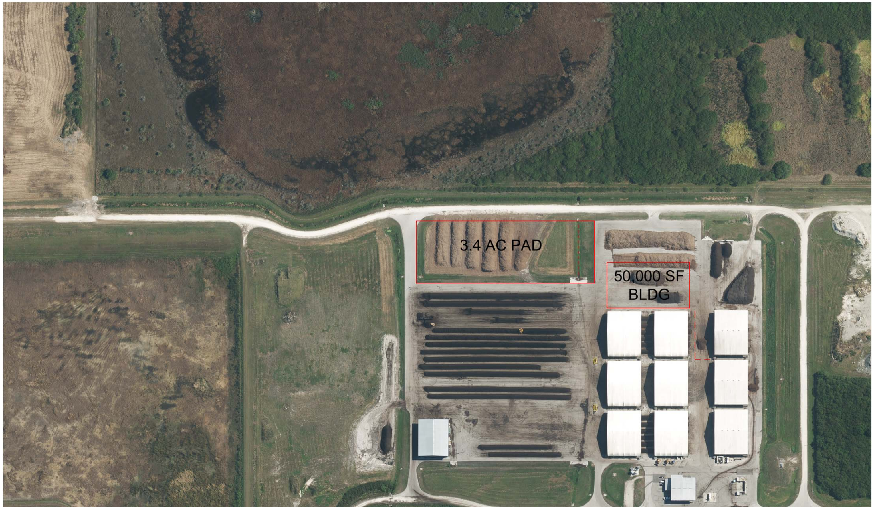
LEE-HENDRY LANDFILL LCCF EXPANSION
