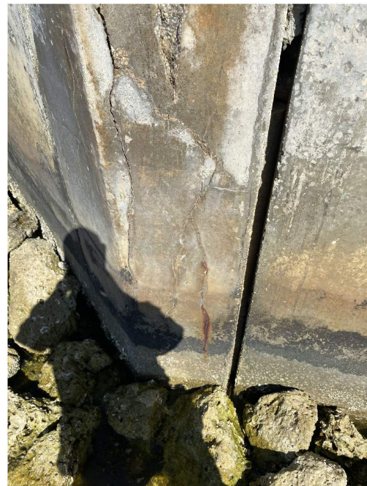
PHOTOS OF BULKHEAD FIRST ANGLE BREAK TO BE REPAIRED
