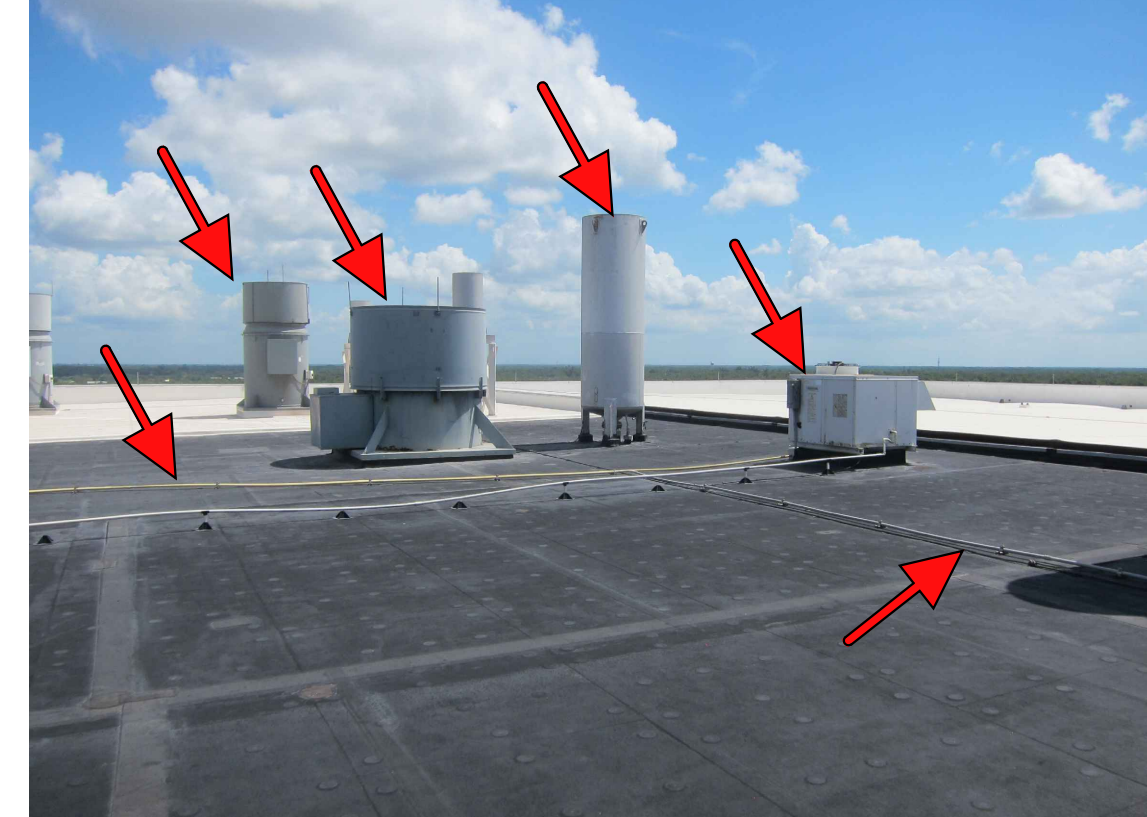
BOILER #1 & #2: EXISTING CONDITIONS OF PENETRATIONS, EQUIPMENT, CONDUIT AND CONDENSATE LINES.
