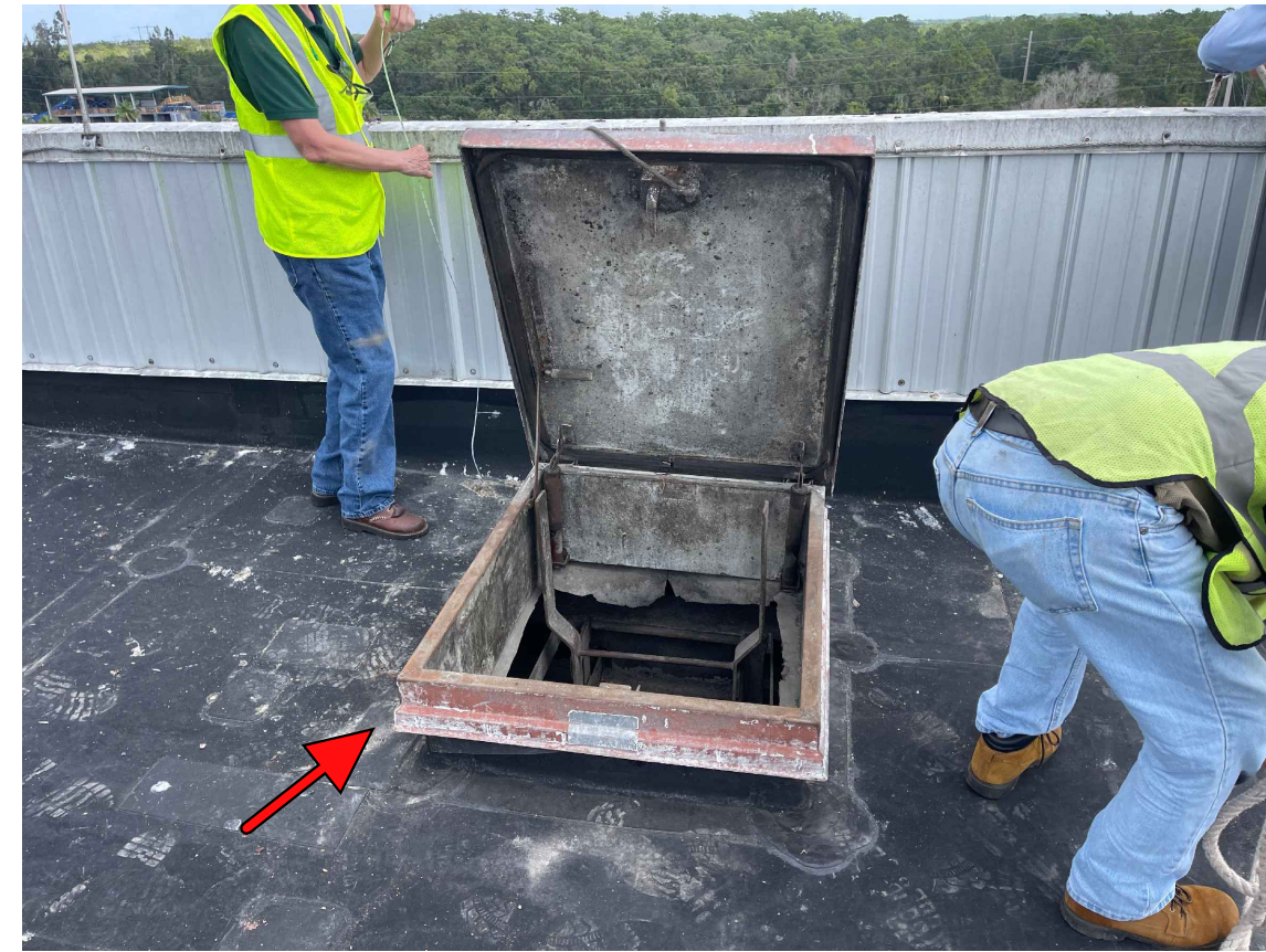
TIPPING FLOOR: EXISTING ROOF HATCH.
