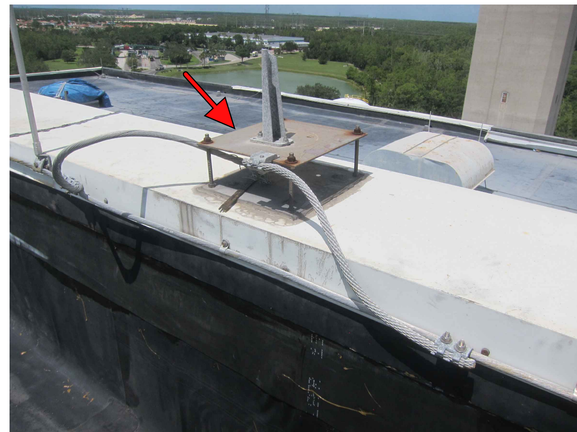
9 BOILER #1 & #2: EXISTING ABANDONED SUPPORT BRACKET OVER PARAPET WALL.
