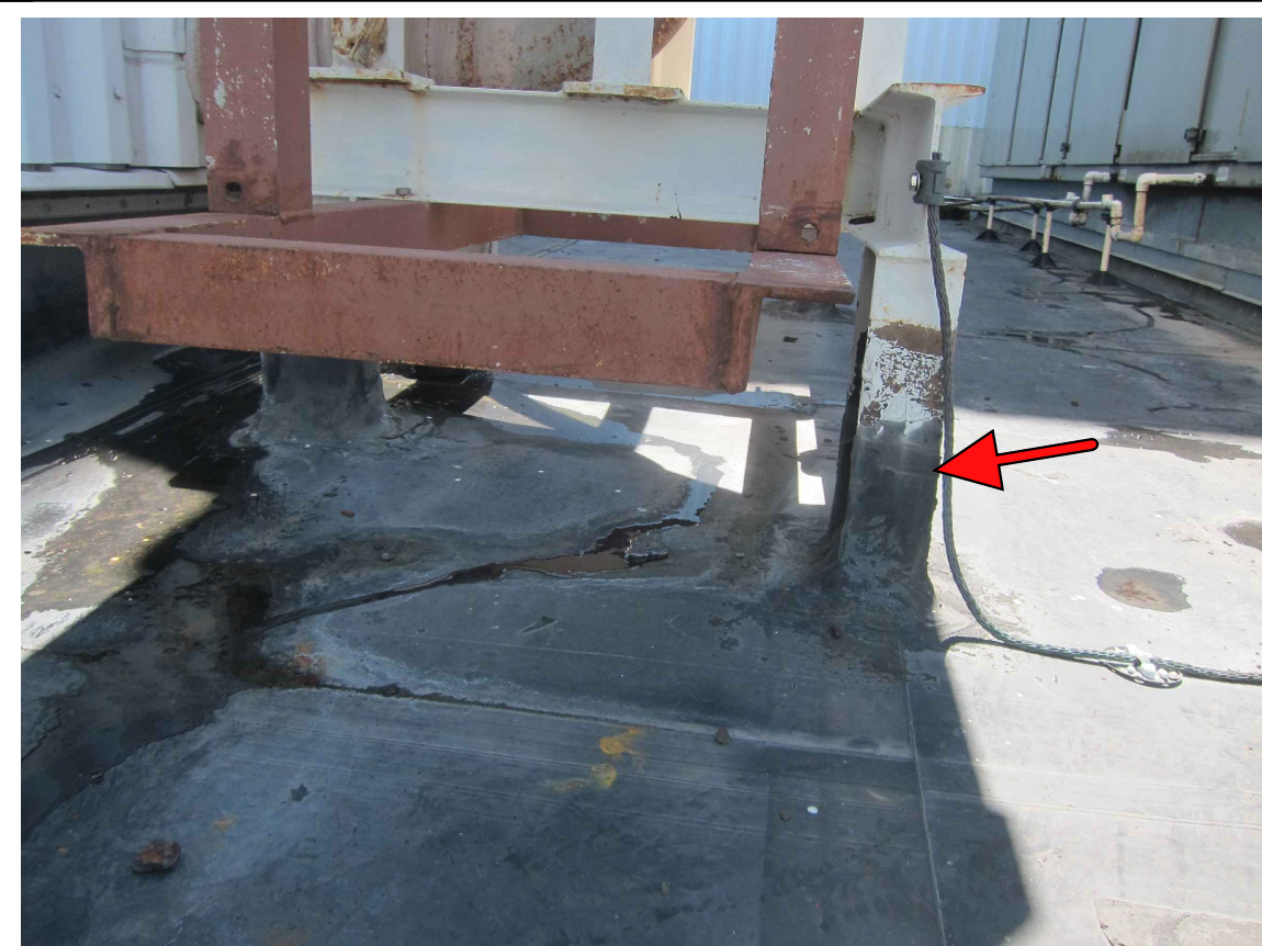
TG #1: EXISTING STRUCTURAL STEEL PENETRATIONS.
