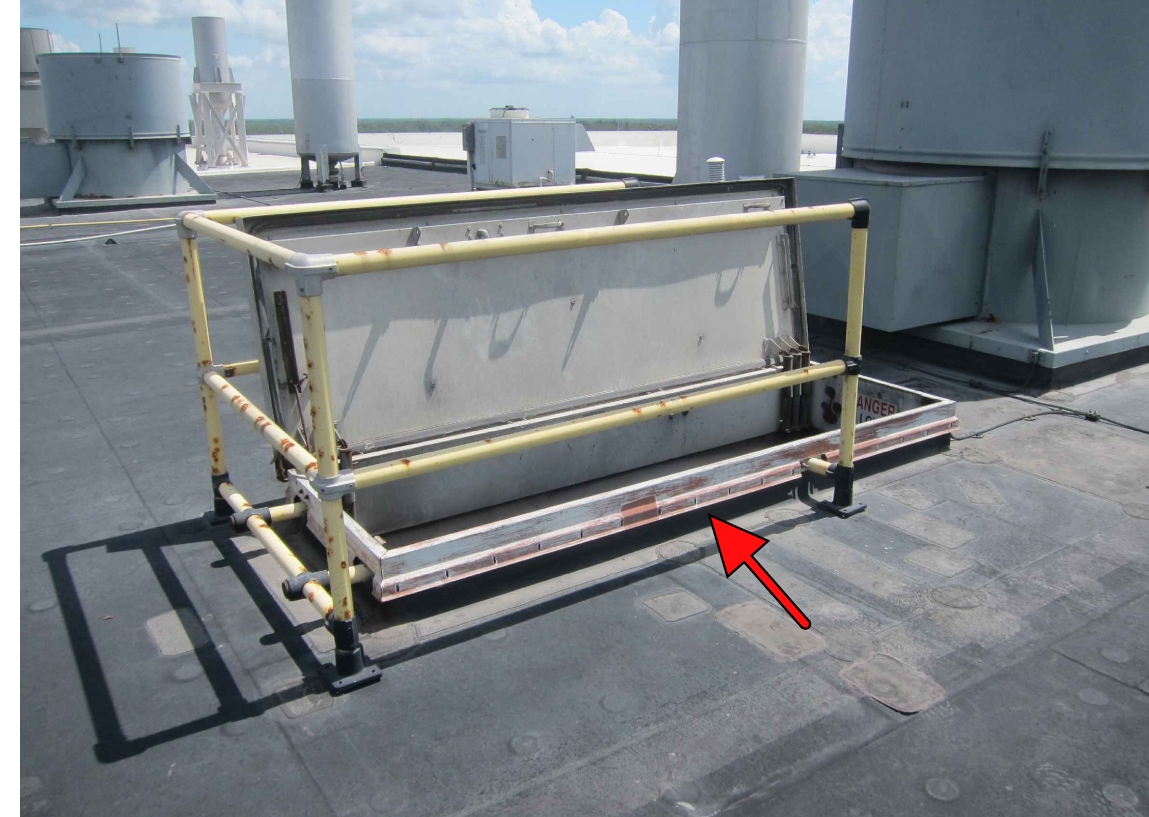
BOILER #1 & #2: EXISTING ROOF HATCH.
