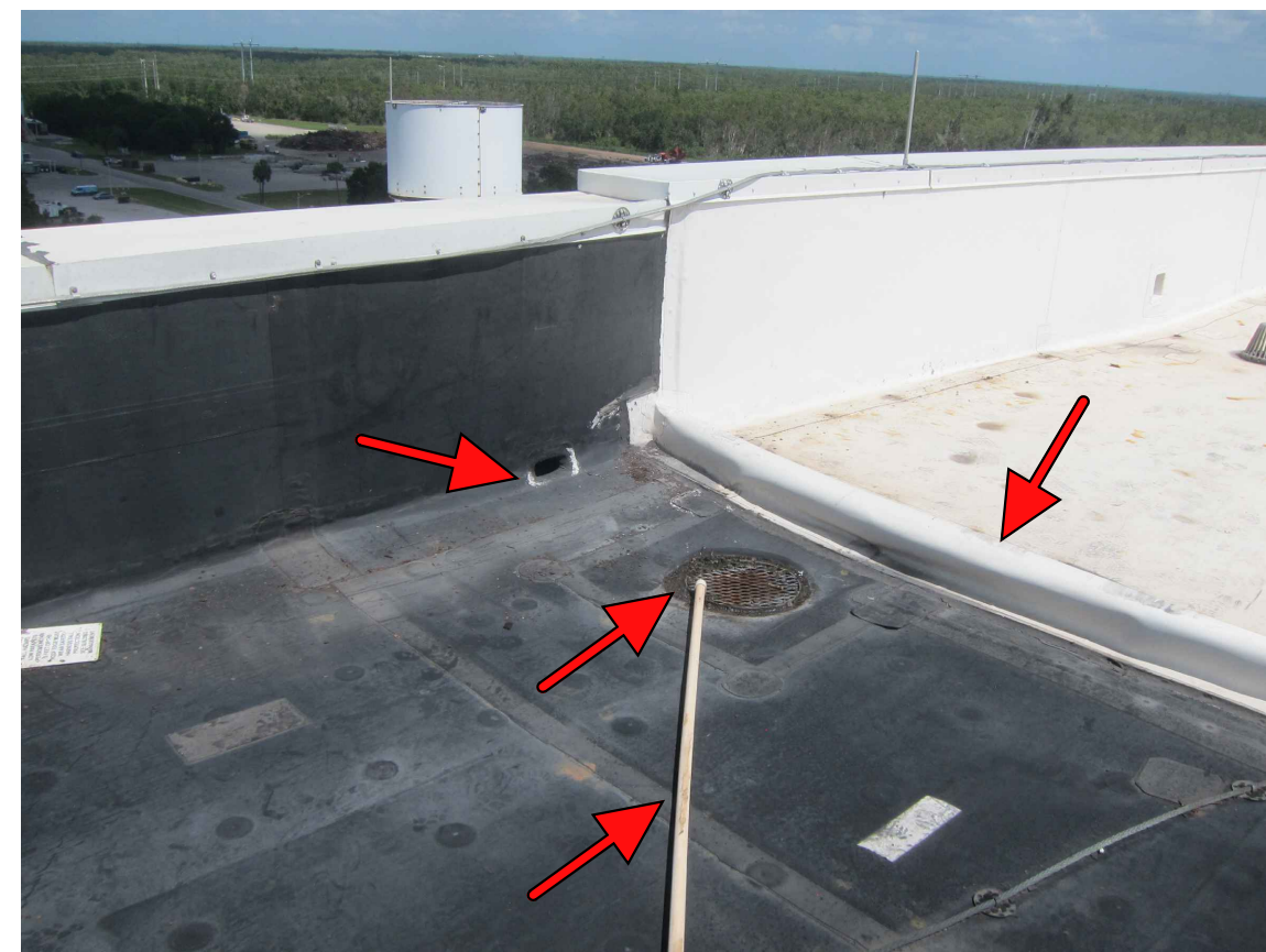
5 BOILER #1 & #2: EXISTING ROOF DRAIN, OVERFLOW SCUPPER, EXPANSION JOINT AND CONDENSATE LINE.
