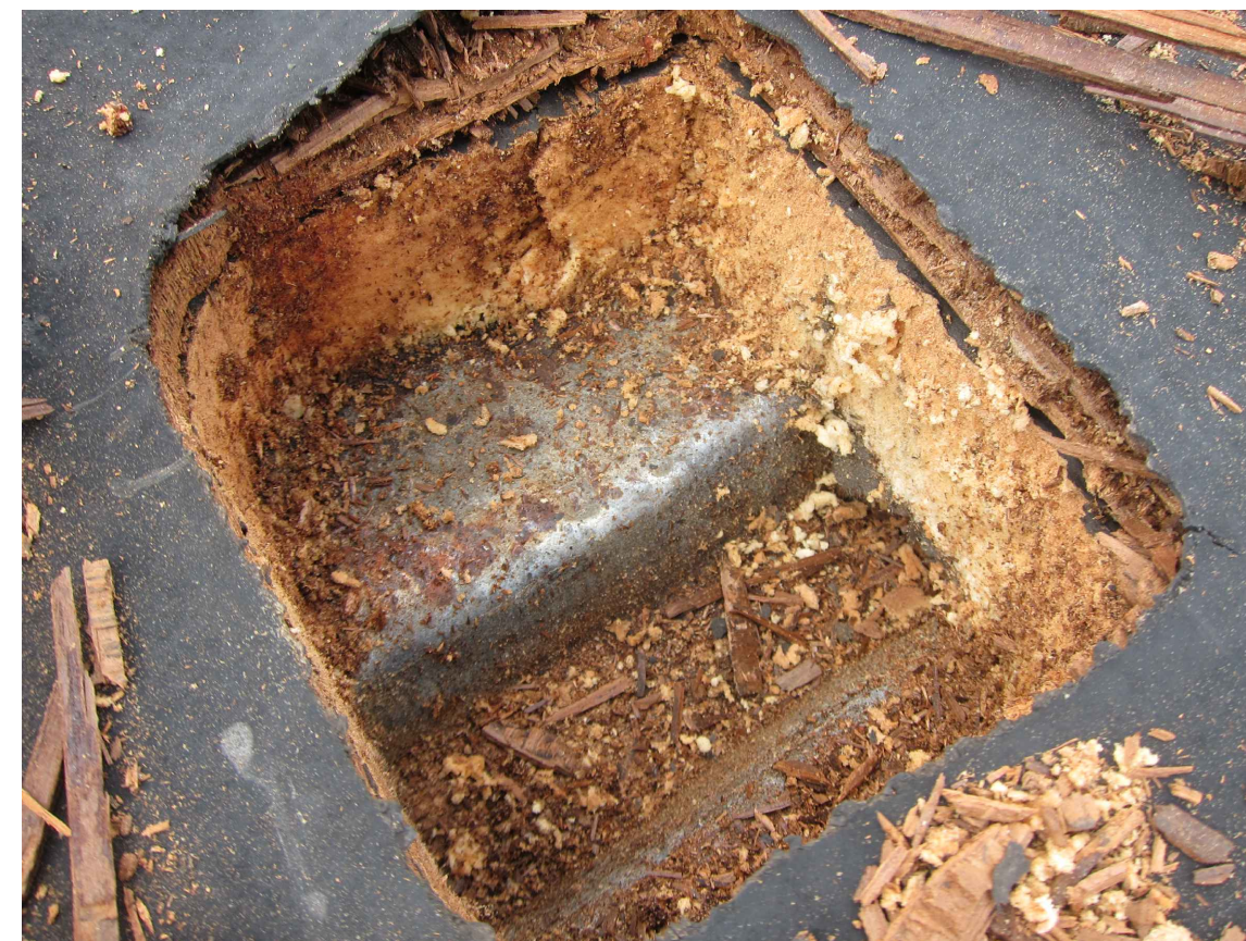
TIPPING FLOOR: ROOF CORE OF EXISTING ROOF SYSTEM. EXAMPLE OF AN AREA OF STEEL DECK THAT REQUIRES CLEANING AND PAINTING.
