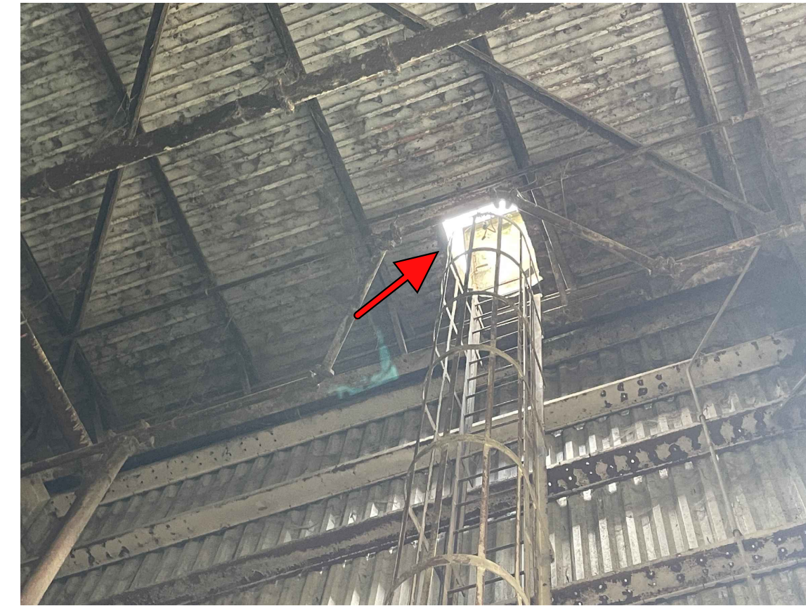
TIPPING FLOOR: EXISTING ROOF HATCH AND LADDER.
