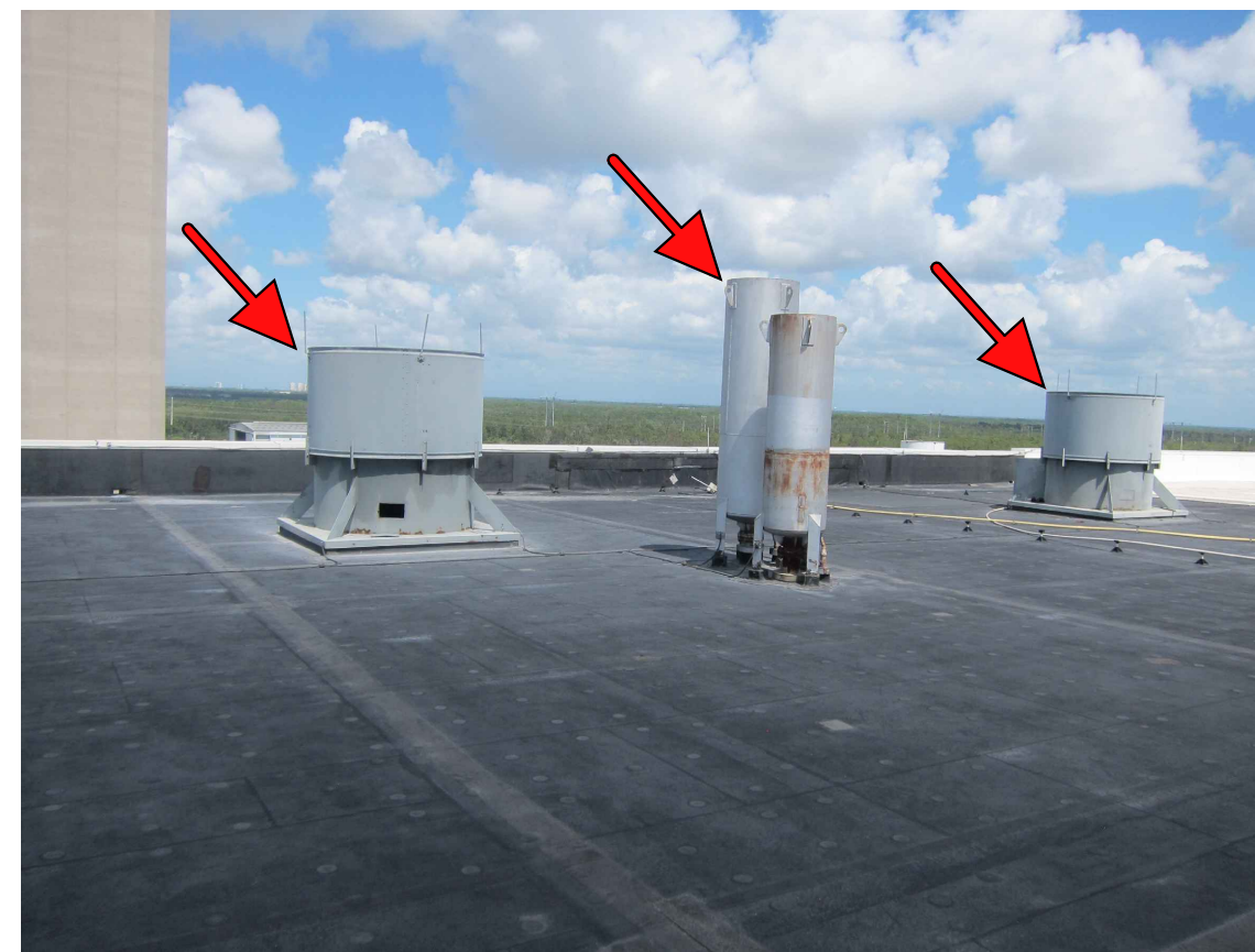
7 BOILER #1 & #2: EXISTING STACKS.
