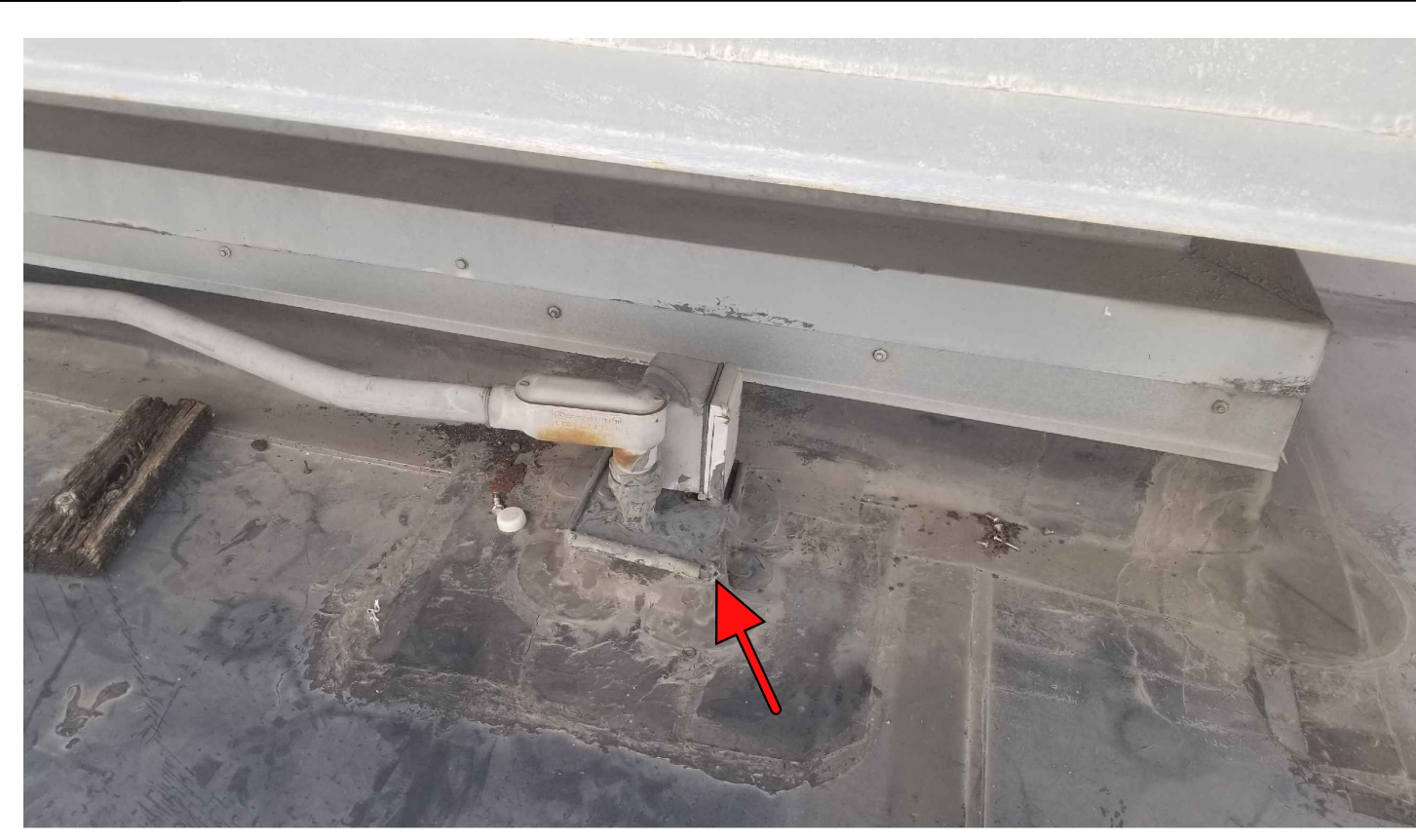
TG #1: EXISTING PITCH PAN WITH ELECTRICAL SERVICE.
