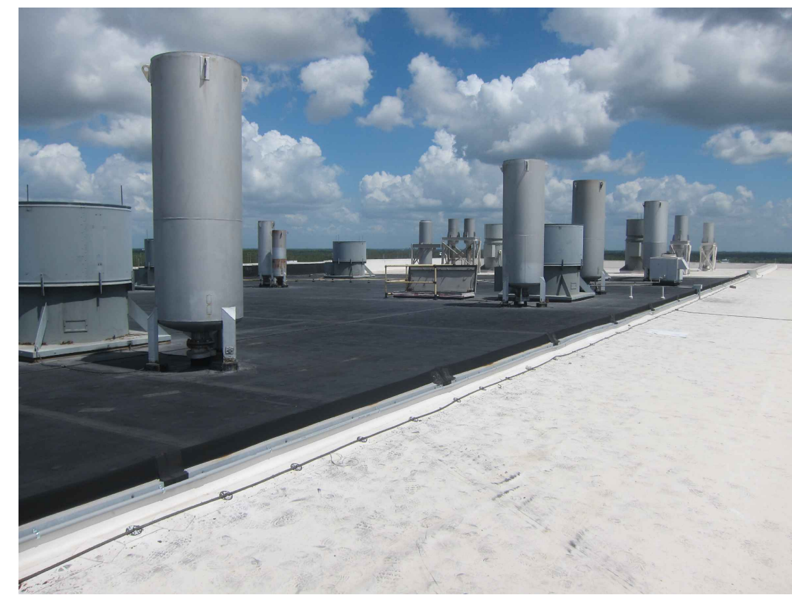
2 BOILER #1 & #2: EXISTING CONDITIONS OF PENETRATIONS, STACKS, EQUIPMENT AND EXPANSION JOINT.
