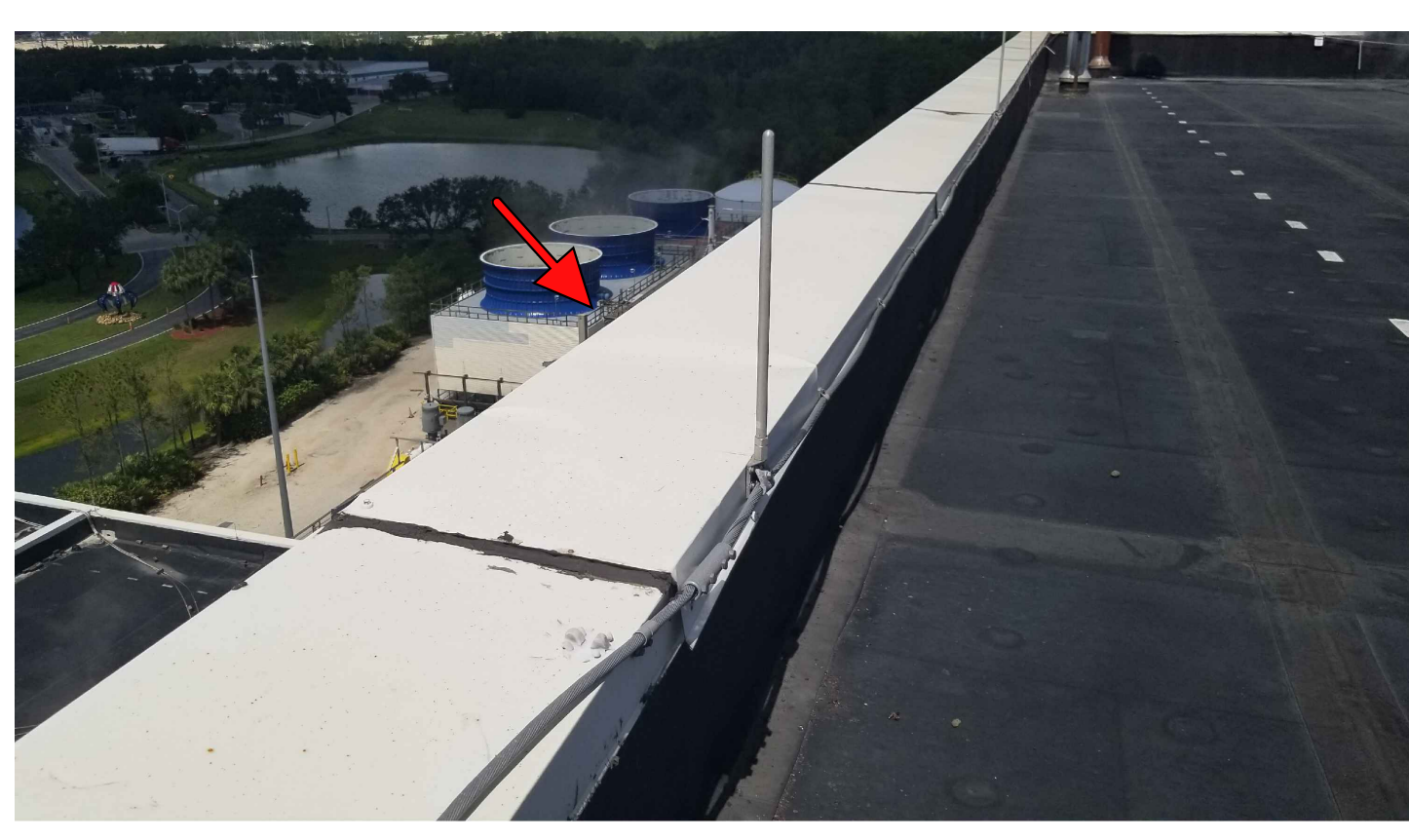
10 BOILER #1 & #2: EXISTING PARAPET WALL.
