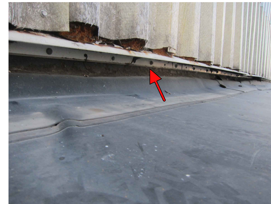
TG #1: EXISTING COUNTER-FLASHING CONDITION BELOW METAL PANEL SIDING.
