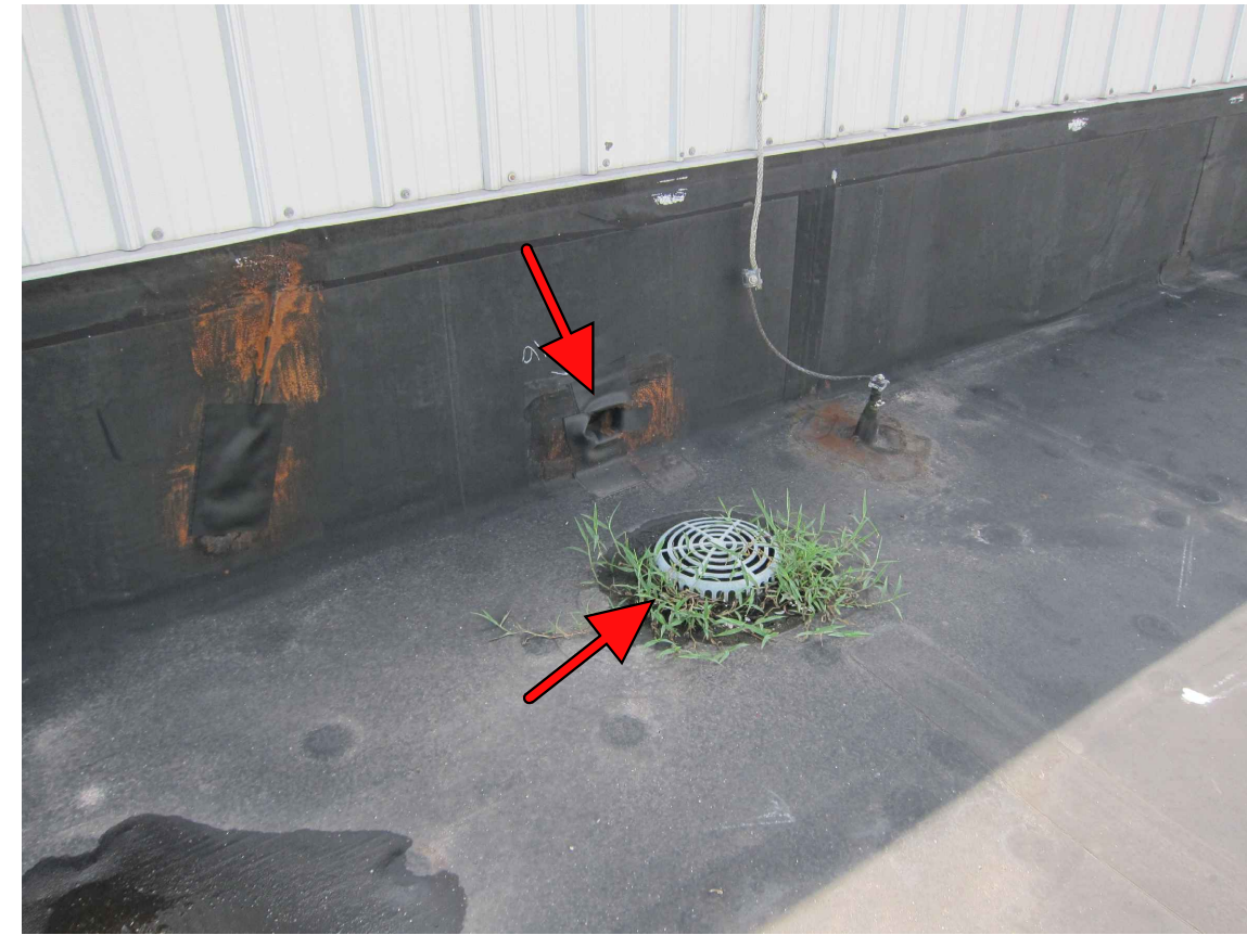
TIPPING FLOOR: EXISTING ROOF DRAIN AND OVERFLOW SCUPPER.
