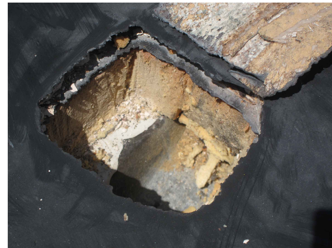
TG #1: ROOF CORE OF EXISTING ROOF SYSTEM.
