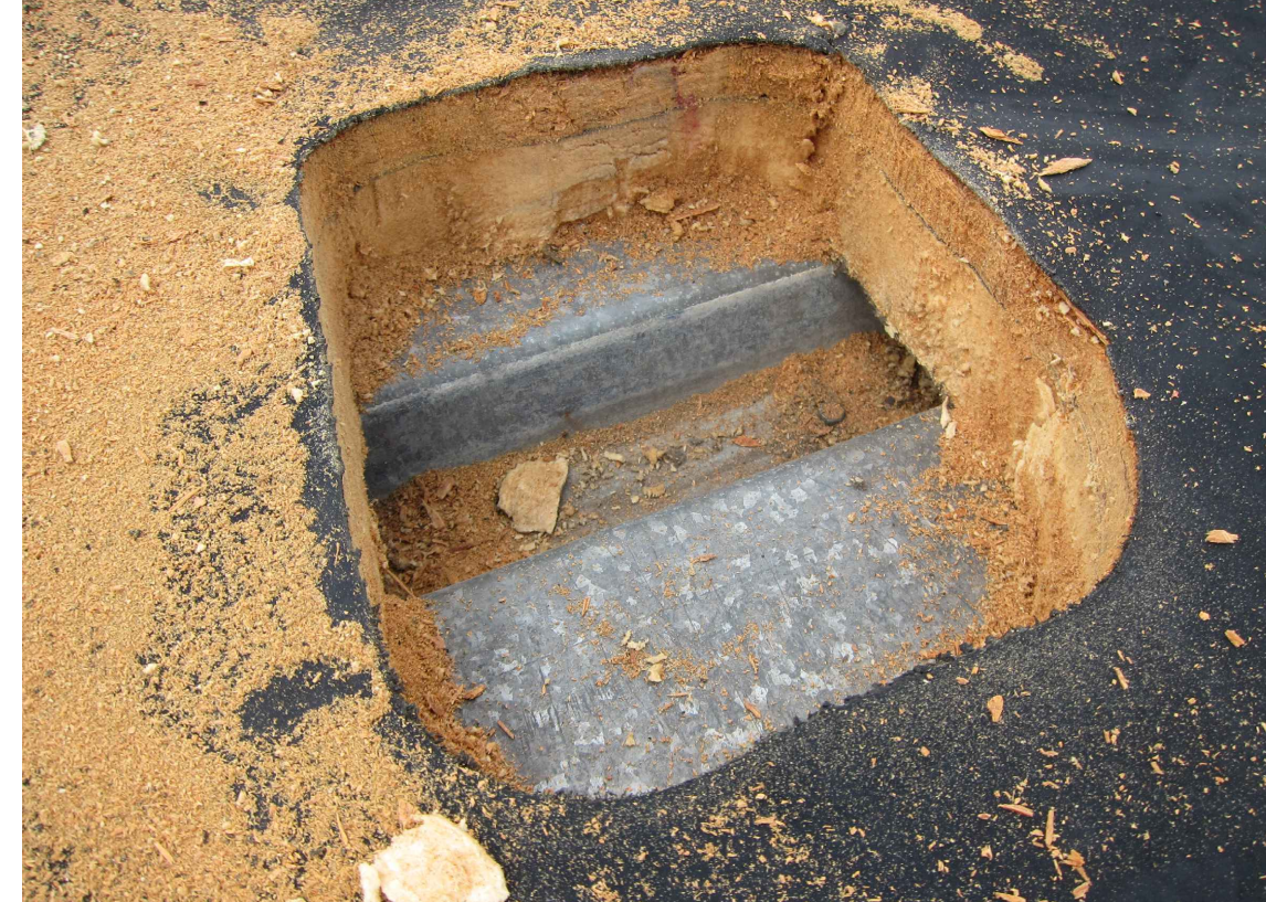
BOILER #1 & #2: ROOF CORE OF EXISTING ROOF SYSTEM.
