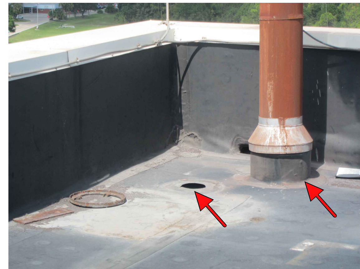
6 BOILER #1 & #2: EXISTING ROOF DRAIN, OVERFLOW SCUPPER AND GAS FLUE.
