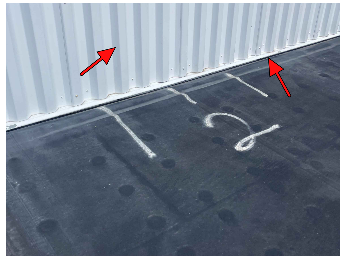
TIPPING FLOOR: EXISTING COUNTER-FLASHING AND METAL SIDING PANEL AT ELEVATION CHANGE.
