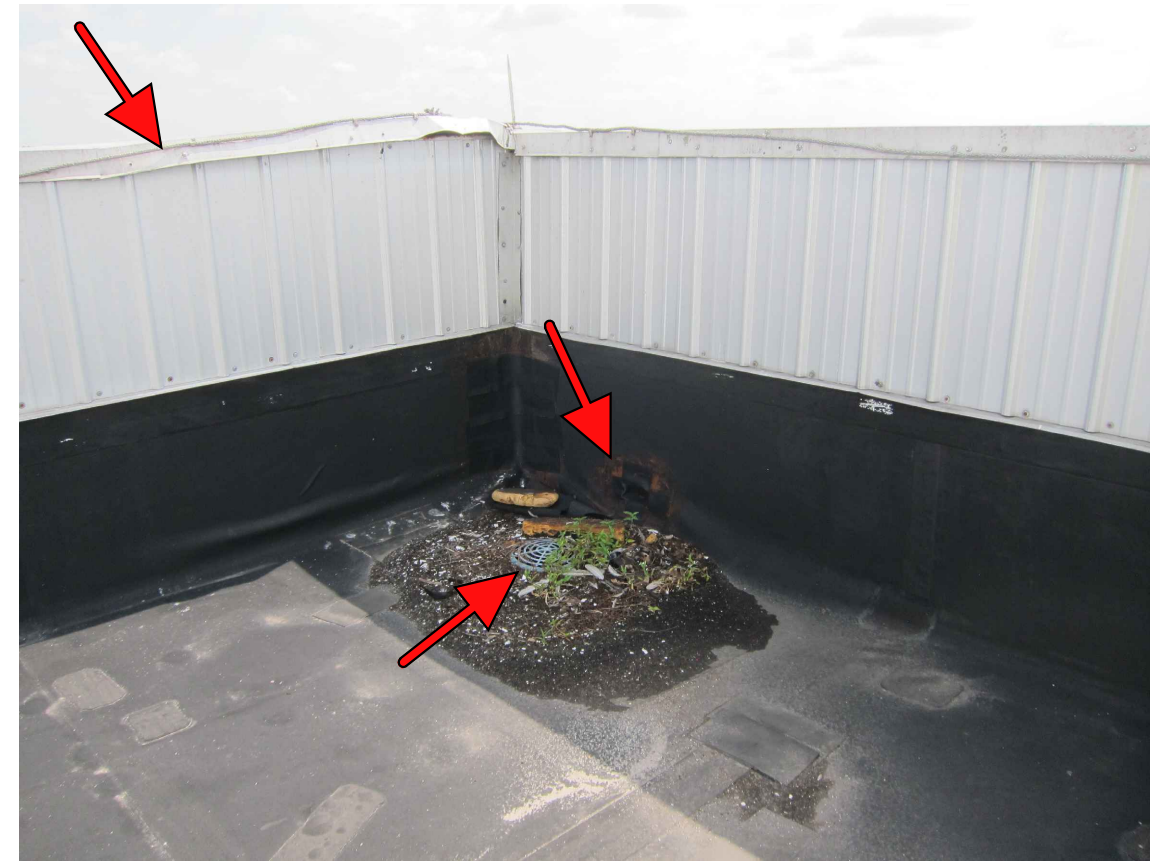
TIPPING FLOOR: EXISTING ROOF DRAIN, OVERFLOW SCUPPER AND PARAPET WALL.
