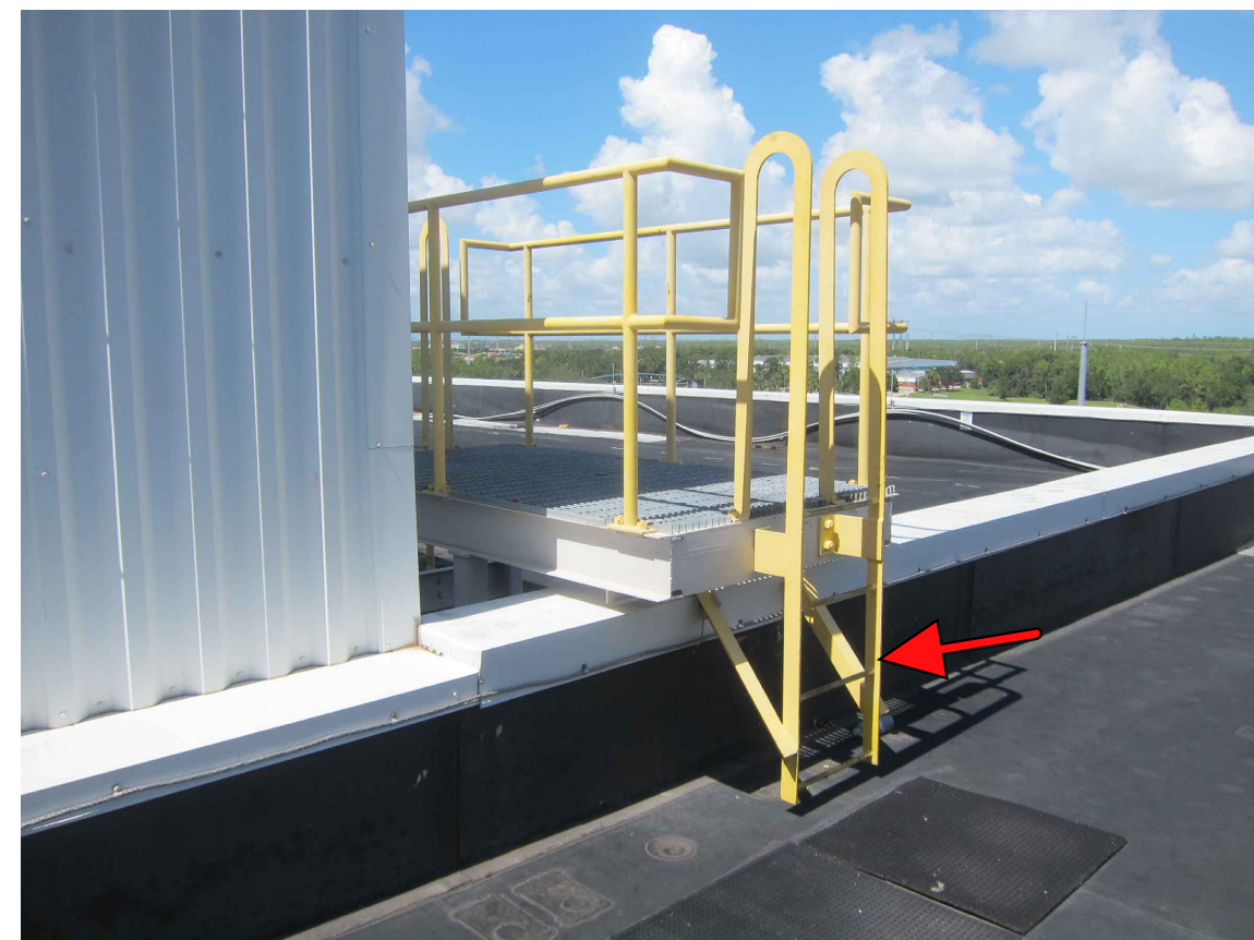
TG #1: EXISTING LADDER OVER PARAPET WALL.
