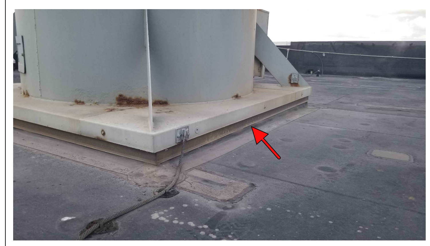
12 BOILER #1 & #2: CLOSE UP AT EXISTING EXHAUST FAN CURB.
