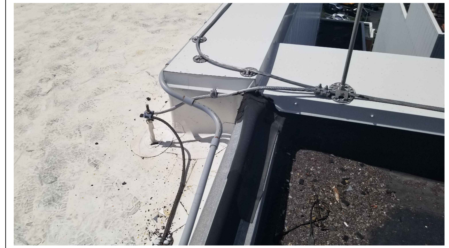
4 BOILER #1 & #2: EXISTING EXPANSION JOINT AT PARAPET INTERSECTION.
