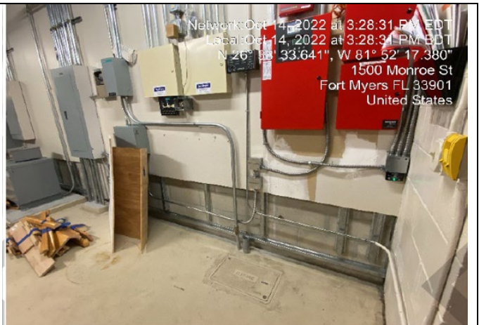
Photo #: 14.03 Description: Electrical Room 103 concrete floor, drywall, vinyl base
