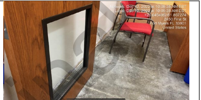
Photo #: 16.01, 16.02, 16.03 Description: Room 126 Head of Circulation carpet tile, baseboard, drywall
