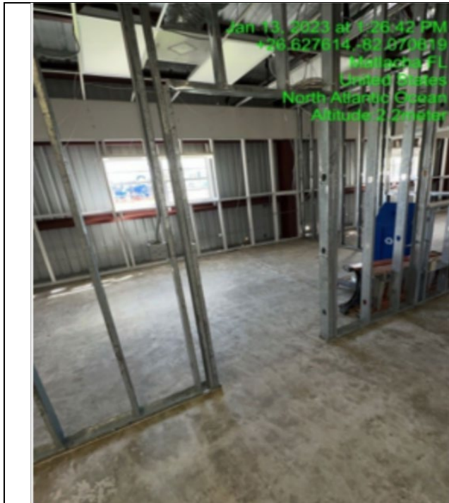
Photo #: 3.02, 3.03, 3.09 Description: Interior door trim
