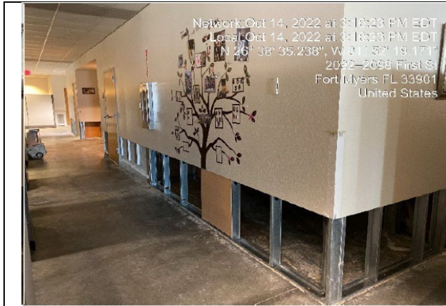
Photo #: 41.01, 41.02, 41.03 Description: Open office 136 flooring, drywall, vinyl base
