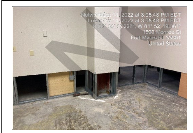
Photo #: 37.01, 37.02, 37.03, 37.04 Description: Office 132 carpet tile flooring, drywall, vinyl base, insulation
