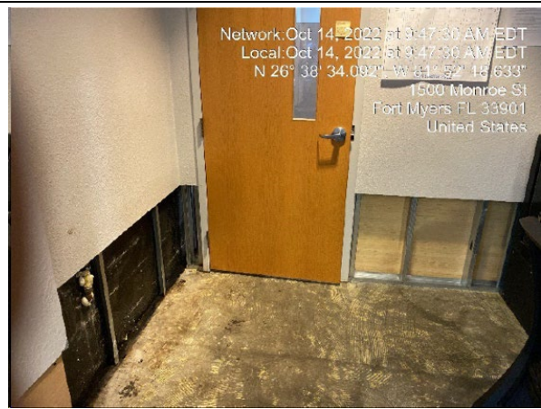
Photo #: 24.01, 24.02, 24.03, 24.04 Description: Cashiers office 119 flooring, drywall, vinyl base, insulation
