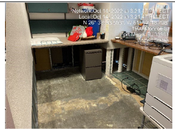
Photo #: 26.01, 26.02, 26.03, 26.04, 26.05 Description: Permit counter (staff side) 121 flooring, drywall, Vinyl base, insulation
