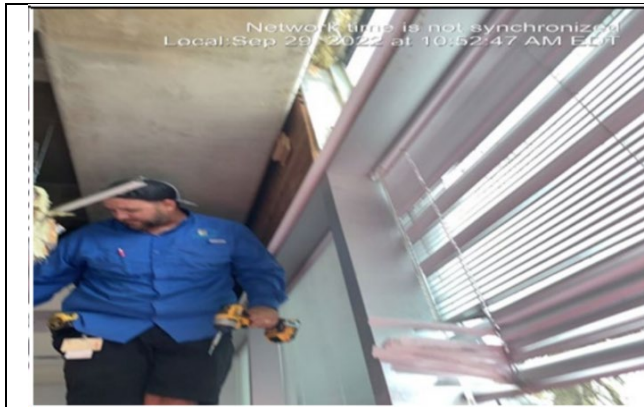
Photo #: 6.01, 6.08 Description: Blind and Double pane tinted glass window
