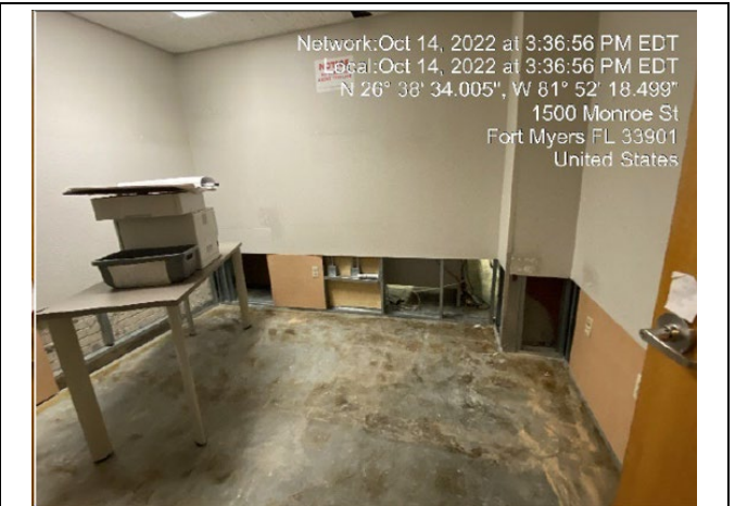
Photo #: 21.01, 21.02, 21.03, 21.04 Description: Mail room 106 vinyl composition tile, drywall, vinyl base, insulation
