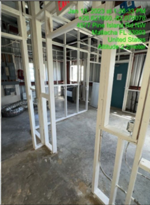
Photo #: 3.13 Description: Interior door trim
