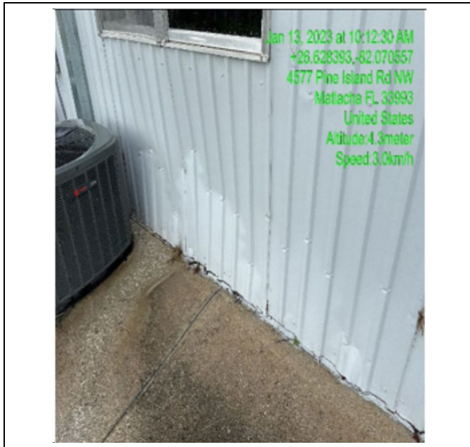
Photo #: 2.06 Description: Siding Northwest (Typical)
