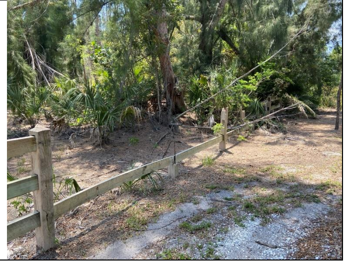
Photo #: 19.02 Description: Pressure treated wood rails
