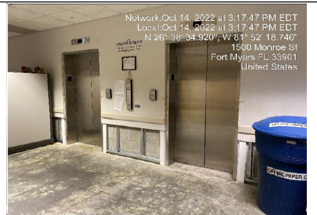
Photo #: 40.01, 40.02, 40.03 Description: Staff Elevator Lobby 135 flooring, drywall, vinyl base
