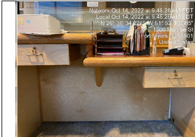
Photo #: 24.01, 24.02, 24.03, 24.04 Description: Cashiers office 119 flooring, drywall, vinyl base, insulation
