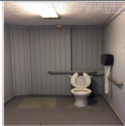
Photo #: 1.04 Description: Concession ADA Bathroom (typical)
