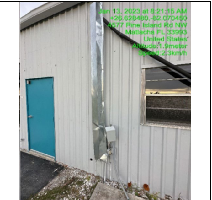
Photo #: 2.05 Description: Siding Southwest side (Typical)
