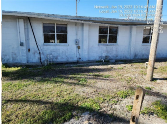
Photo #: 1.24, 1.25 Description: Gutter at rear
