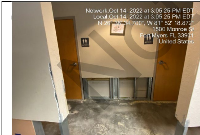
Photo #: 43.01, 43.02, 43.03, 43.04 Description: Toilet Vestibule 138 flooring, drywall, base, insulation
