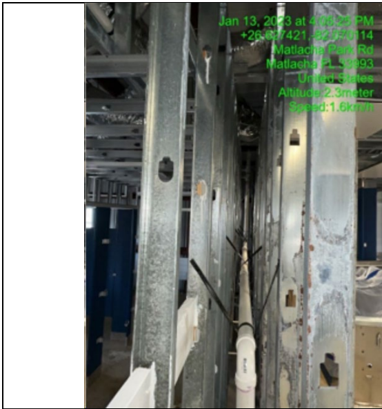
Photo #: 9.02 Description: Sanitary, waste and vent piping.
