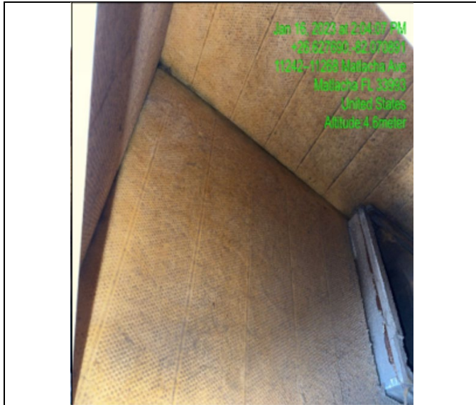
Photo #: 5.08 Description: Duct Board Supply & run
