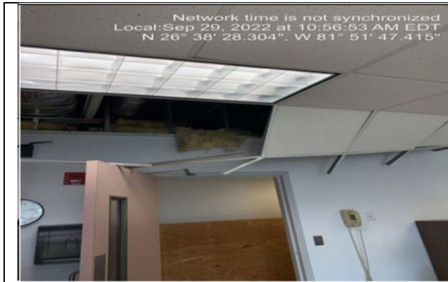
Photo #: 6.03, 6.07, 6.10 Description: Foil Face Fiberglass insulation, ceiling tiles
