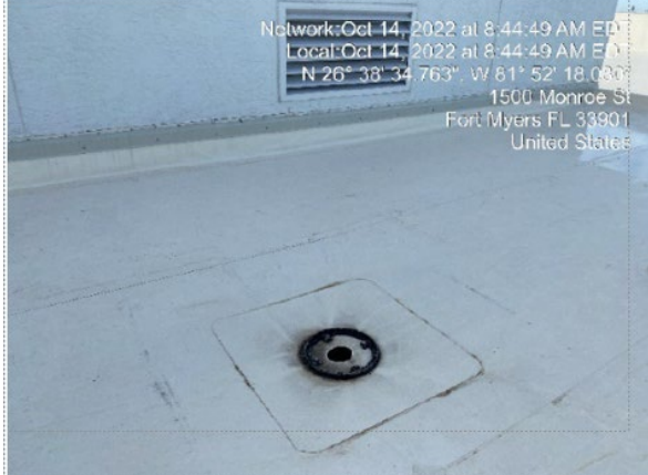
Photo #: Roof 1.03 Description: Plastic roof drain debris cover
