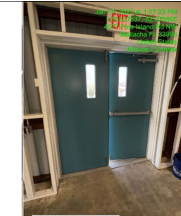
Photo #: 3.11 Description: Exterior door trim
