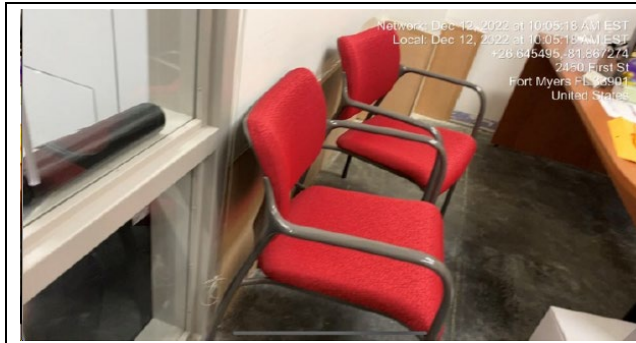
Photo #: 15.01, 15.02, 15.03 Description: Room 125 Regional Manager carpet tile, baseboard, drywall
