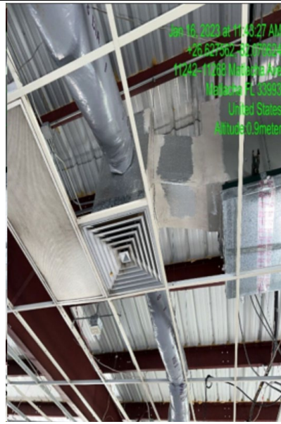
Photo #: 3.01 Description: Acoustical Ceiling Tiles
