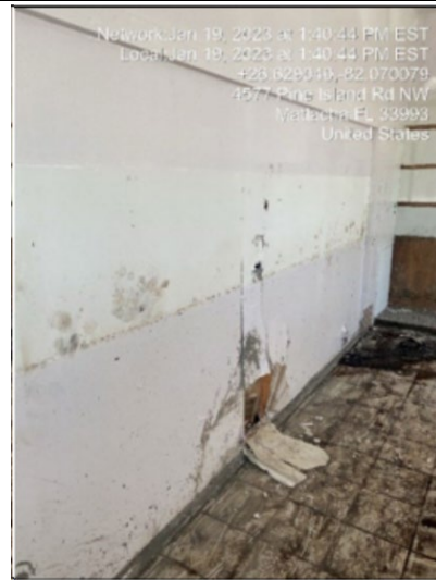
Photo #: 3.03, 3.09 Description: Library inside wall mold growth above high-water mark
