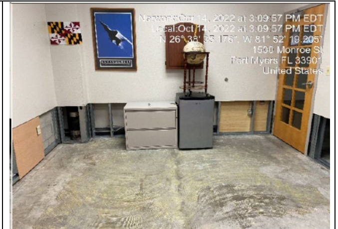
Photo #: 37.01, 37.02, 37.03, 37.04 Description: Office 132 carpet tile flooring, drywall, vinyl base, insulation
