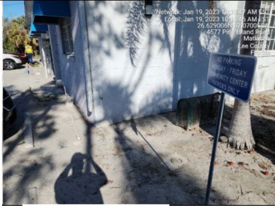
Photo #: 1.25 Description: Gutter downspout
