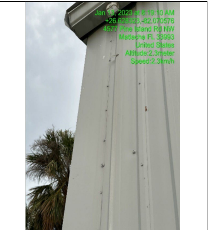
Photo #: 2.01 Description: Downspout Southeast corner (typical)
