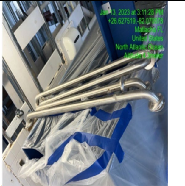
Photo #: N/A Description: Displaced bathroom specialties/accessories
