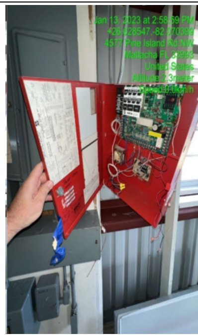
Photo #: 12.01 Description: Fire alarm panel.
