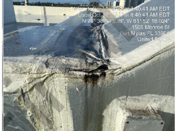
Photo #: Roof 1.01 Description: Metal duct tape/mastic McQuay Air Handler Unit #9
