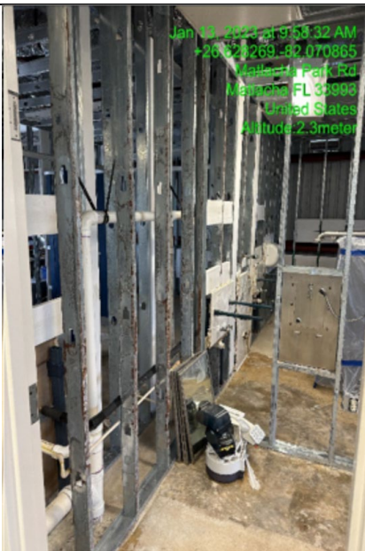
Photo #: 3.02, 3.05 Description: Sheetrock and metal studs
