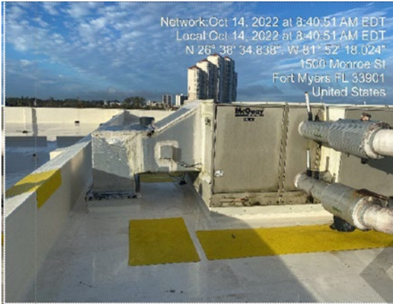
Photo #: Roof 1.01 Description: Metal duct tape/mastic McQuay Air Handler Unit #9
