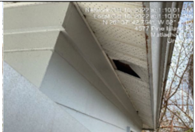
Photo #: 01.02 Description: Northeast corner Soffit
