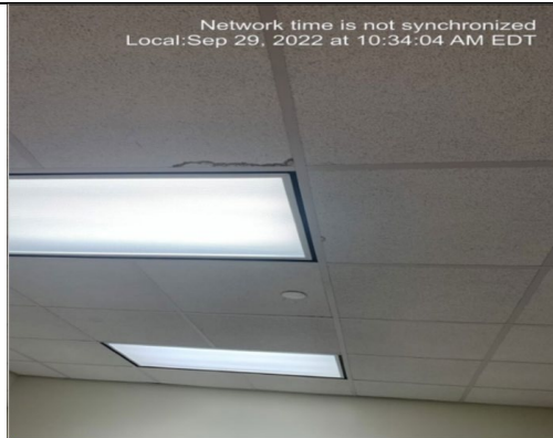
Photo #: 2.01 Description: Ceiling Tiles (Armstrong 807 tegular edge)
