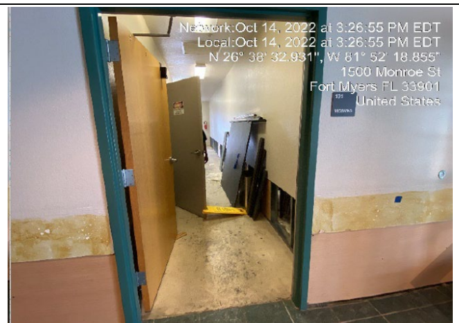
Photo #: 11.02, 11.03 Description: Vestibule 109 floor tile, drywall, ceramic tile base
