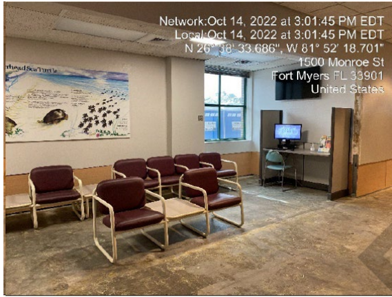
Photo #: 22.01, 22.02, 22.03, 22.04, 22.05 Description: Permitting 117 flooring, drywall, vinyl base, drywall, wood vertical trim
