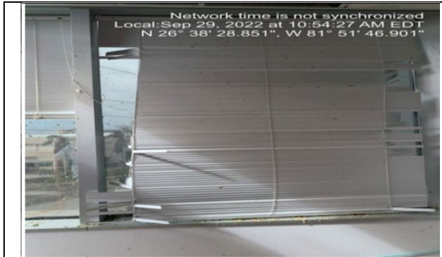
Photo #: 6.02, 6.08 Description: Blind and double pane tinted glass window
