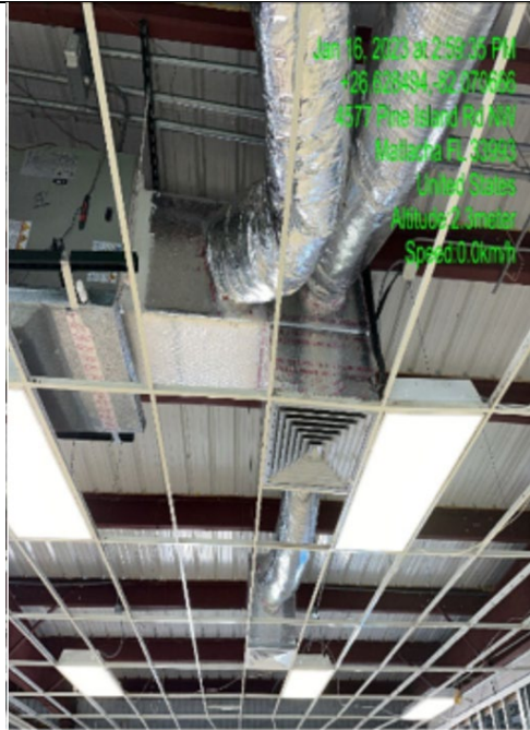
Photo #: 5.02, 5.09 Description: HVAC Air Handler Unit in ceiling space.
