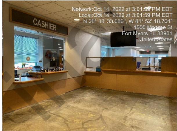
Photo #: 22.06 Description: Permitting 117 temporary wall, counter front panel
