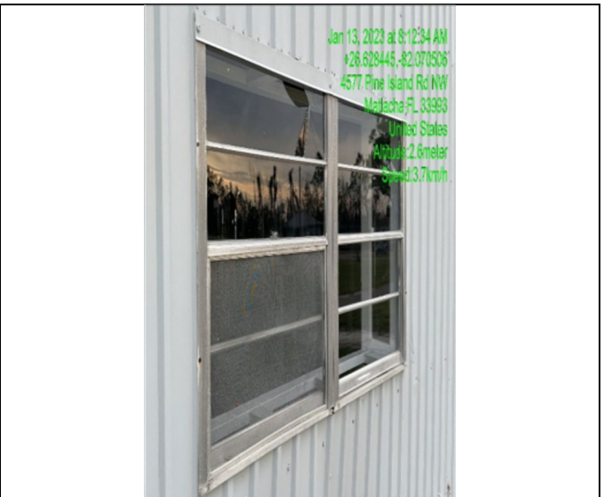
Photo #: 2.07 Description: Window trim exterior Northwest corner (typical)
