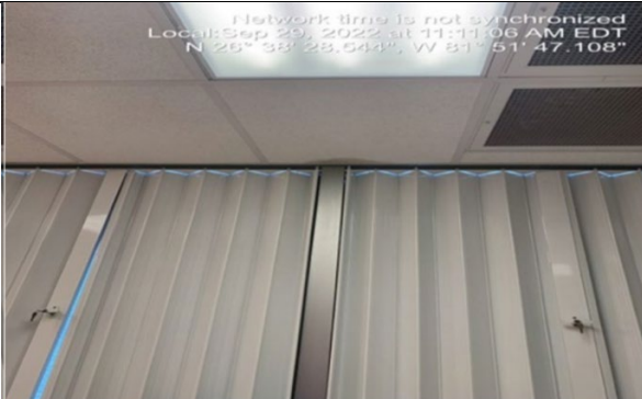
Photo #: 8.01 Description: Ceiling tile (Armstrong 565D)
