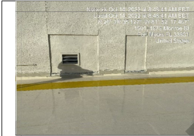
Photo #: Roof 1.04 Description: Stucco and caulking roof penthouse North Exterior wall
