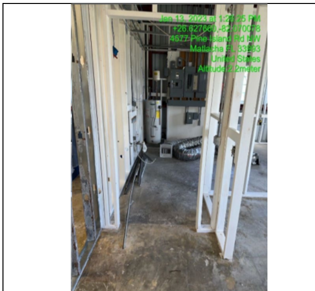
Photo #: 3.13 Description: Interior door trim
