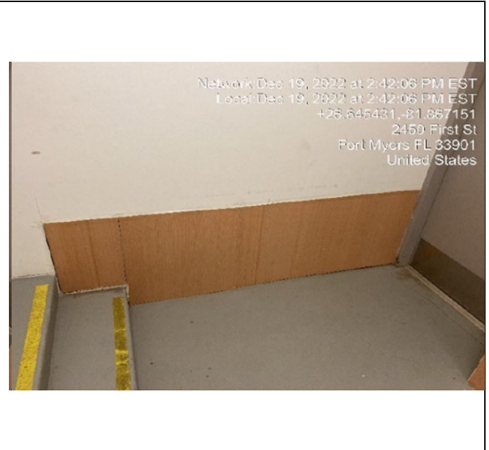
Photo #: 14.01, 14.02 Description: Room 124 Book Return baseboard, drywall
