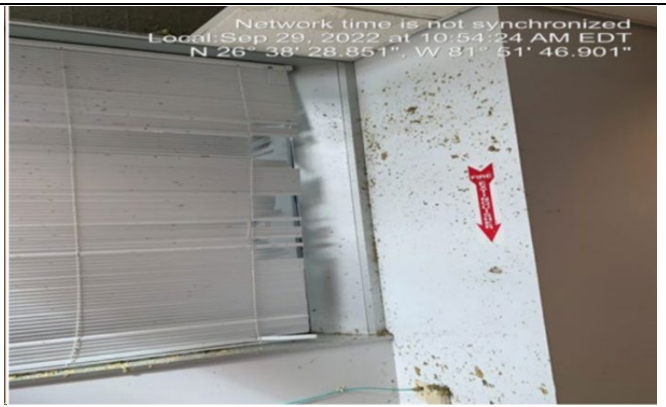
Photo #: 6.02, 6.08 Description: Blind and double pane tinted glass window
