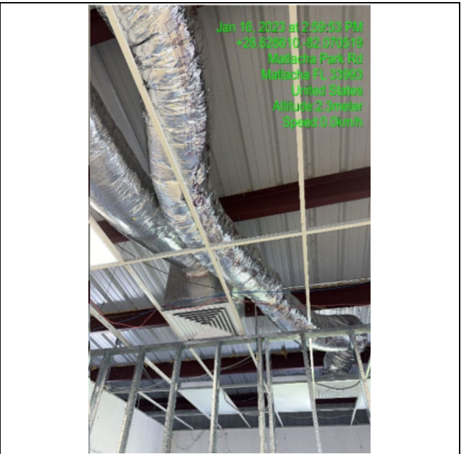
Photo #: 5.10 Description: Flex duct distribution detached/dislodged
