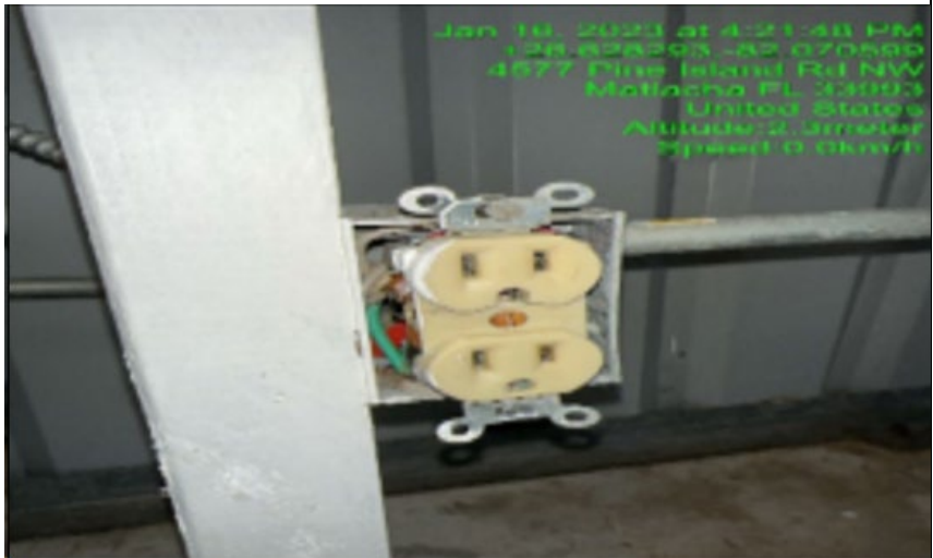
Photo #: 7.04, 7.05, 7.06, 7.08, 7.10 Description: Electrical Outlet, conduit, wiring, all compromised.
