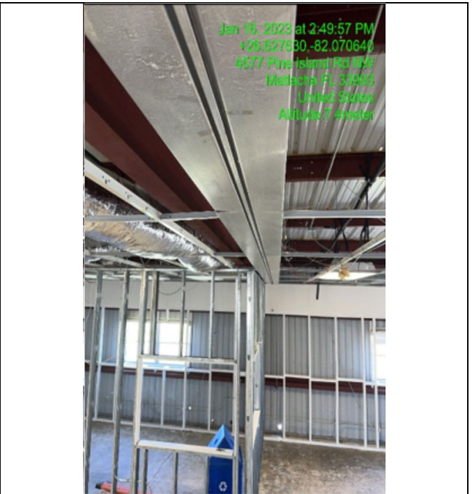
Photo #: 3.08 Description: Folding Room Divider-removed
