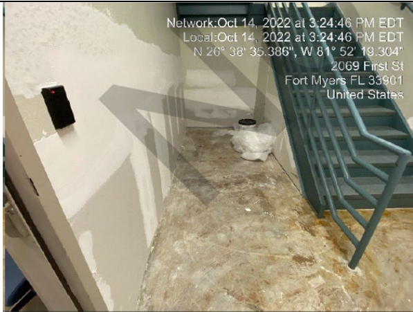
Photo #: 23.01, 23.02, 23.03, 23.04 Description: North stairwell flooring, drywall, vinyl base, insulation
