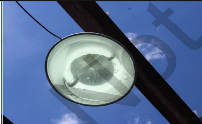
Photo #: 2.01 Description: Low-bay induction type light fixtures with 6' pigtail cords with 20 Amp, twist lock plugs
