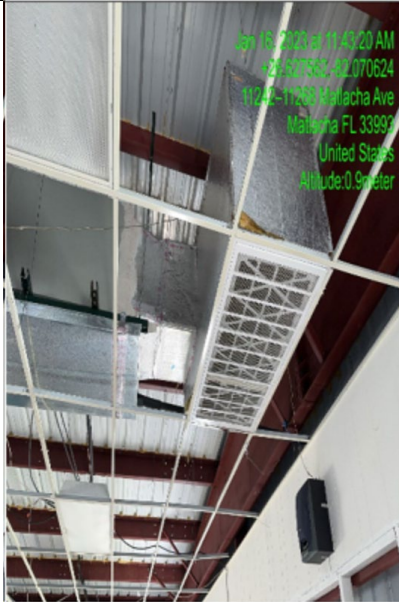
Photo #: 3.01 Description: Acoustical Ceiling Tiles
