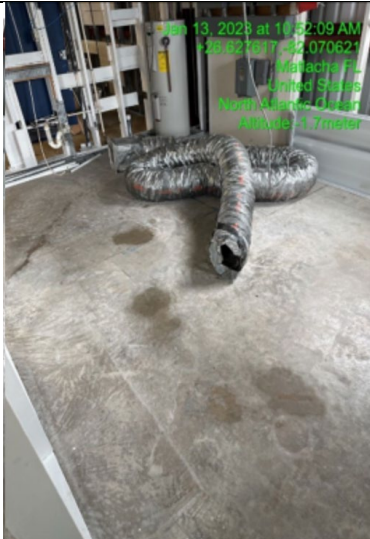
Photo #: 5.01, 5.09 Description: Roof leak observed during rainstorm.
