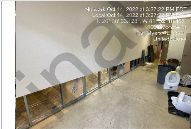
Photo #: 12.01, 12.02, 12.03, 12.04 Description: Receiving 101 flooring, drywall, vinyl base, insulation
