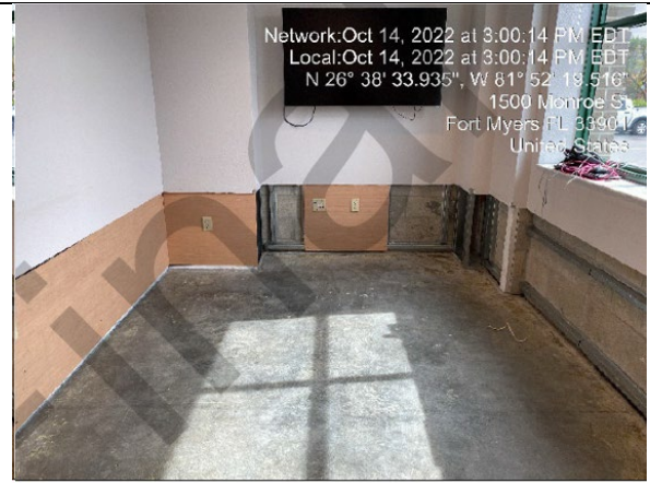
Photo #: 25.01, 25.02, 25.03, 25.04 Description: Conference Room 112 flooring, drywall, vinyl base, insulation
