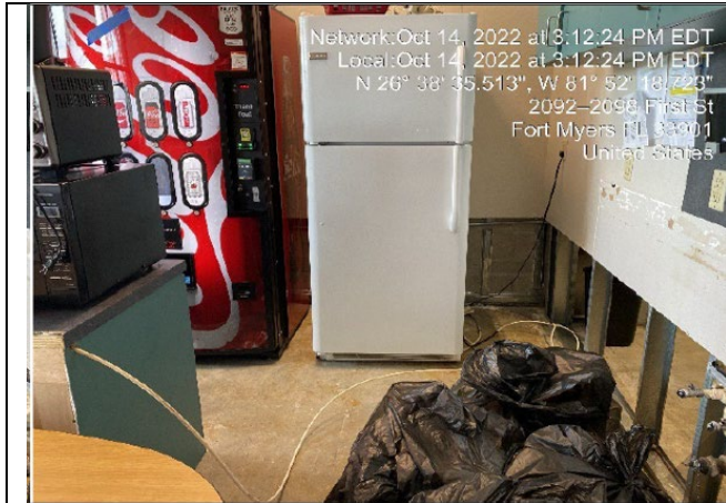
Photo #: 38.01, 38.02, 38.03, 38.04 Description: Break Room 113 flooring, foundation, drywall, vinyl base, insulation
