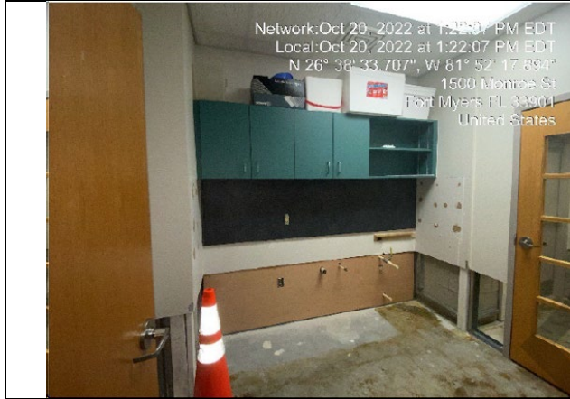
Photo #: 18.01, 18.02, 18.03 Description: Pantry/kitchenette vinyl composition tile flooring, drywall, vinyl base
