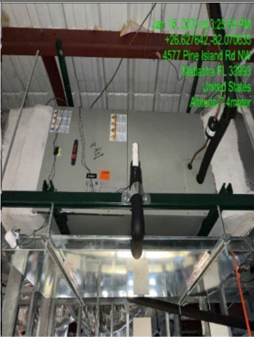
Photo #: 5.01, 5.02, 5.03 Description: HVAC Air Handler Unit in ceiling space.
