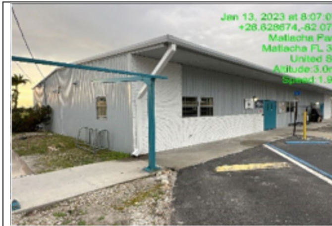
Photo #: 01.01 Description: Roof Southeast corner
