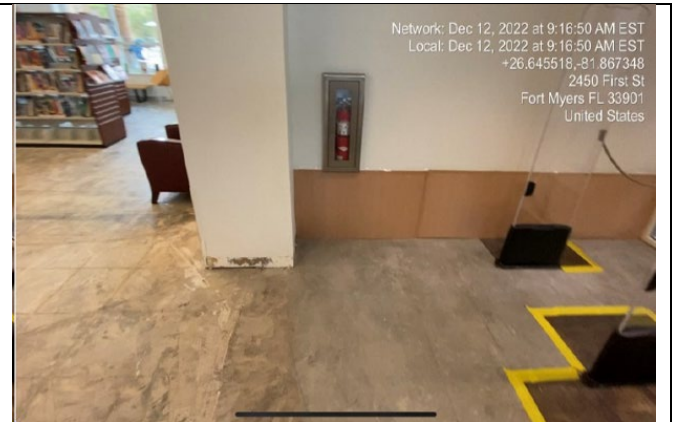
Photo #: 2.01, 2.02, 2.03 Description: Room 105 A Vestibule floor tile, baseboard, drywall
