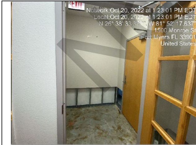
Photo #: 20.01, 20.02, 20.03 Description: Outside Entry hallway vinyl composition tile, drywall, vinyl base
