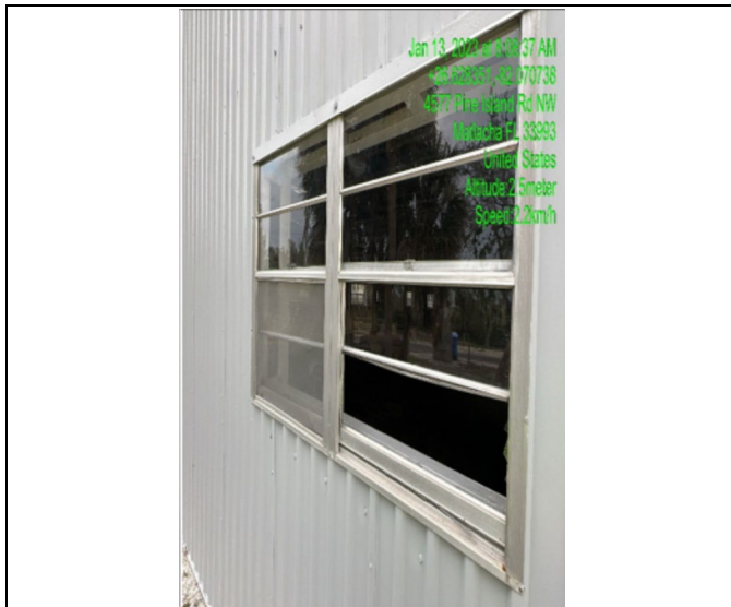
Photo #: 2.07 Description: Window trim exterior Southwest corner (typical)
