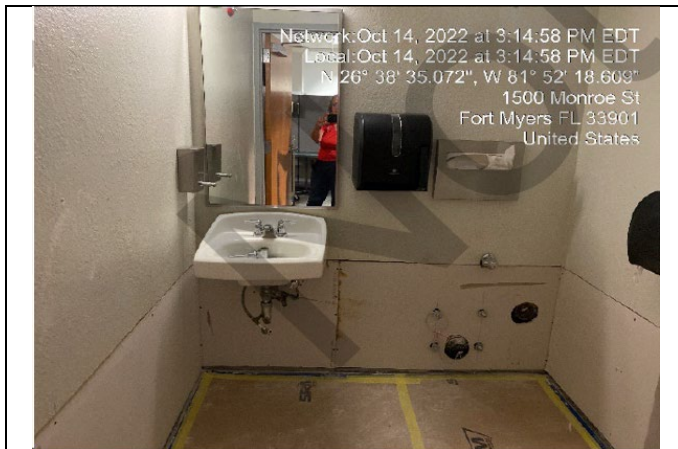
Photo #: 33.01, 33.02, 33.03 Description: Toilet Room 128 flooring, drywall, ceramic tile wall base, insulation
