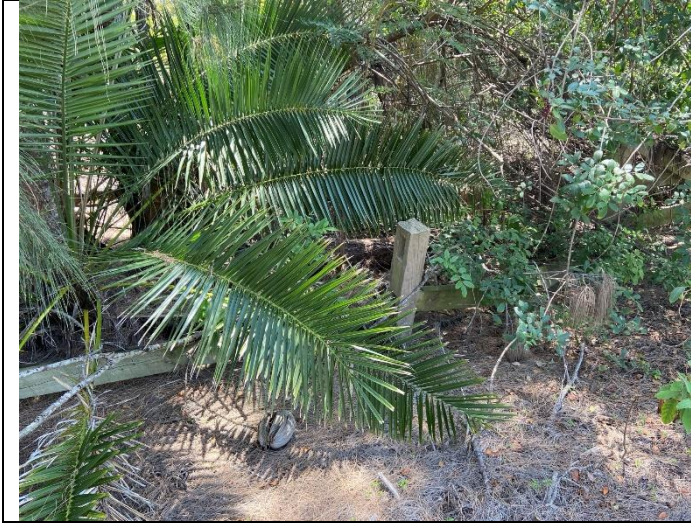
Photo #: 19.01 Description: Concrete fence posts
