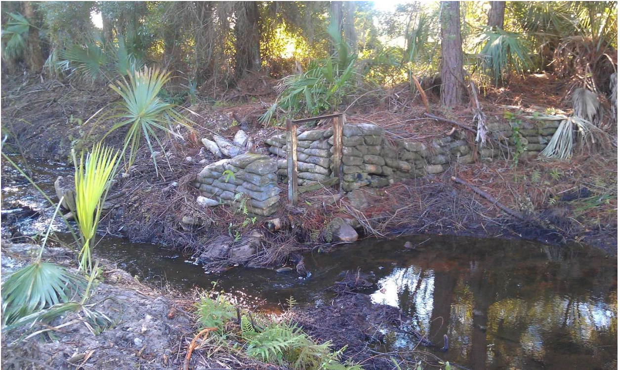
Figure 1: Photos taken of the north weir on 10-06-2011
