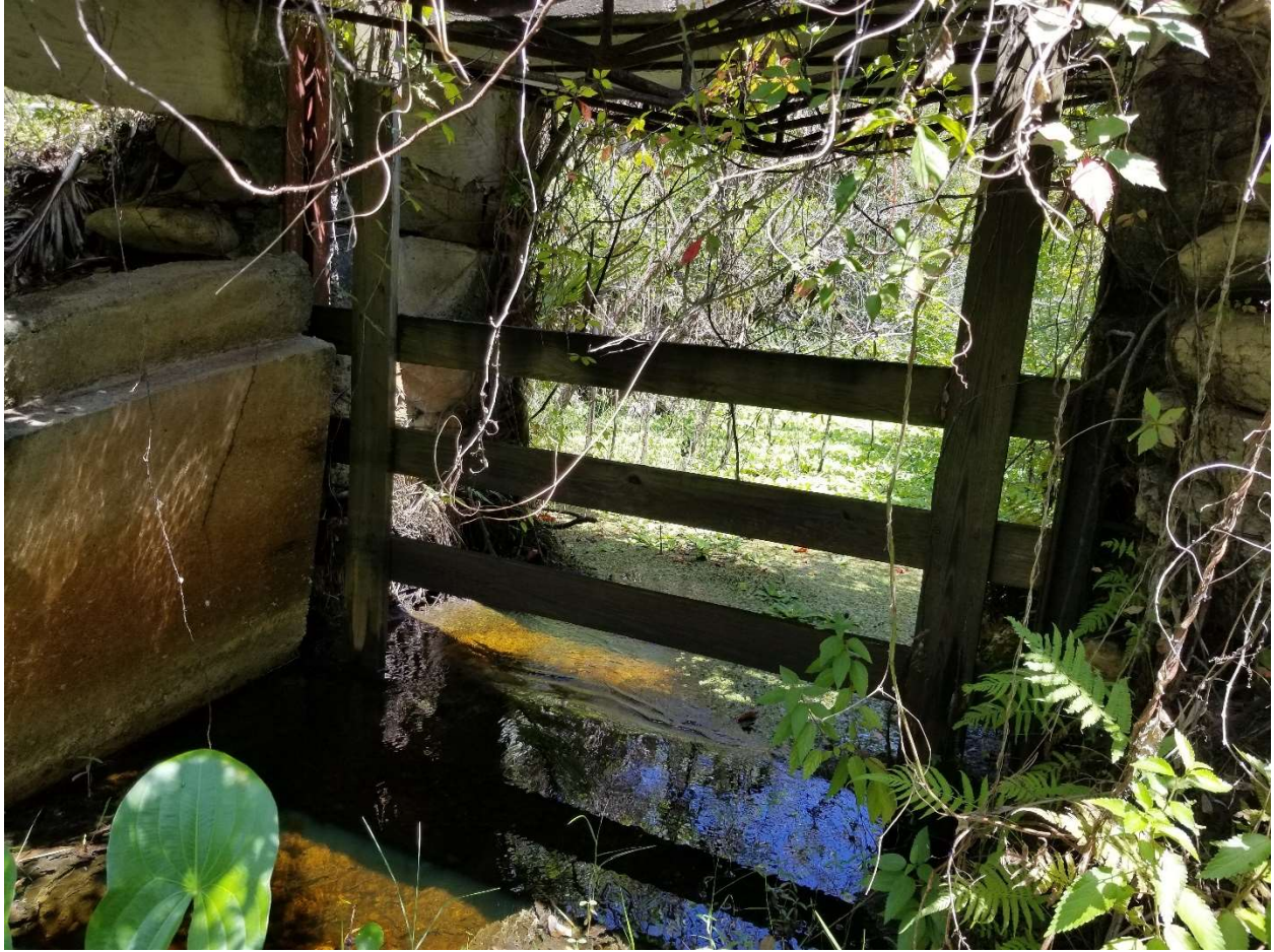
Figure 7: Photo taken of the south weir on 08-25-2023
