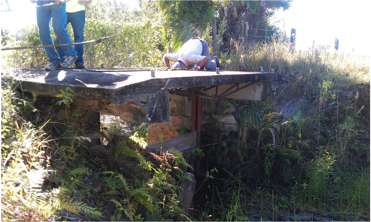
Figure 3: Photo taken of the south weir on 10-06-2011
