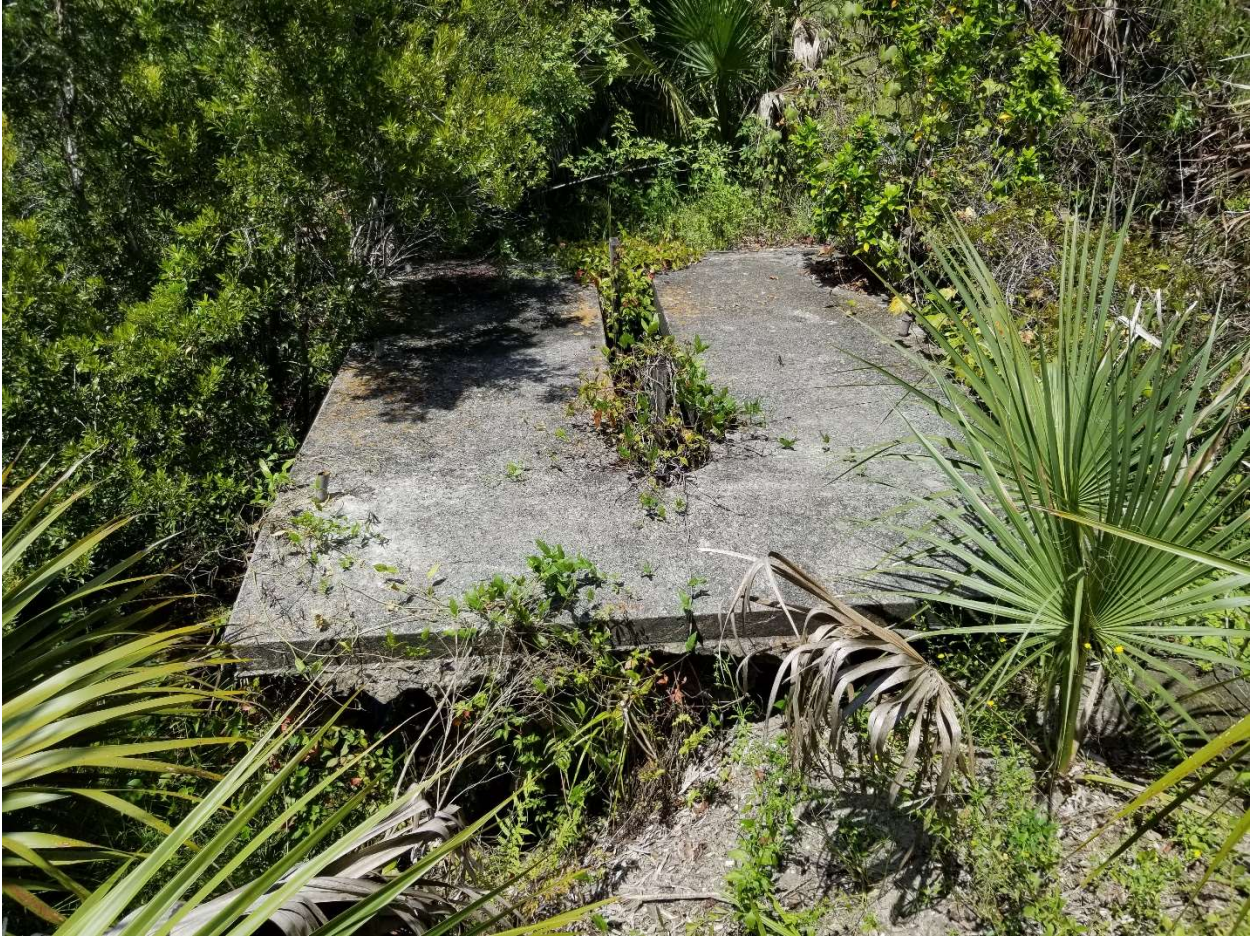
Figure 6: Photo taken of the south weir on 08-25-2023
