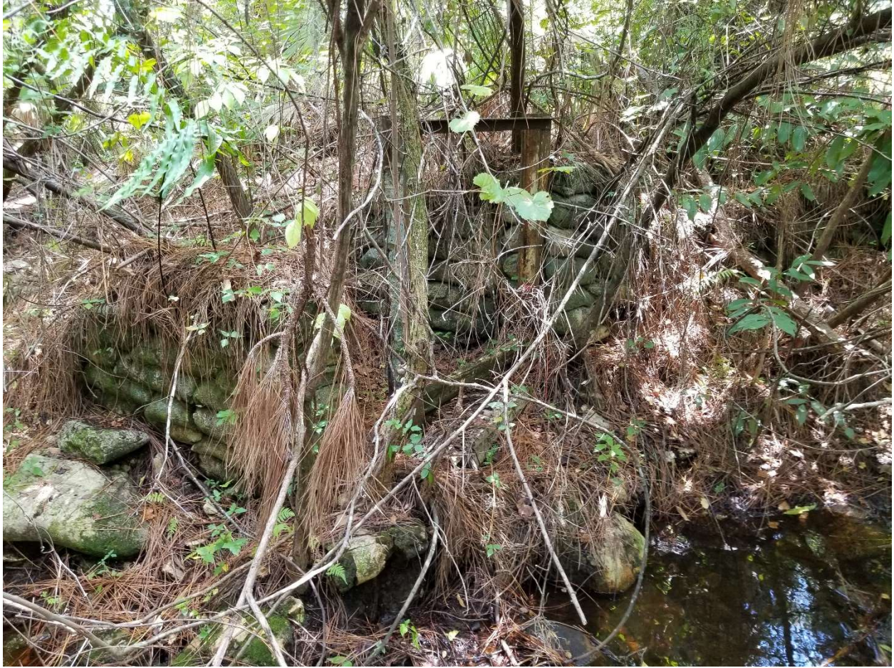
Figure 5: Photo taken of the north weir on 08-25-2023
