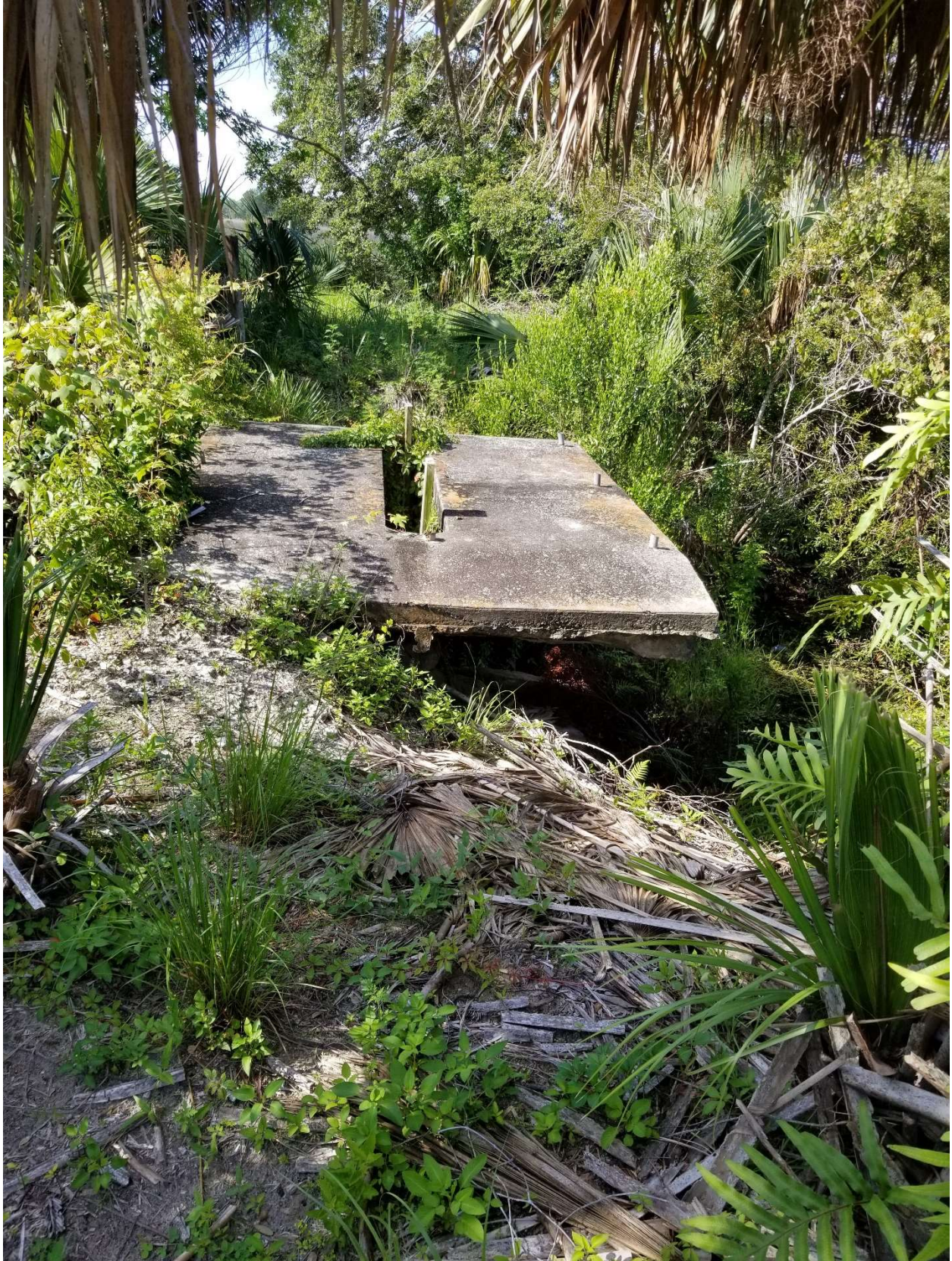
Figure 4: Photo taken of the south weir on 06-19-2018
