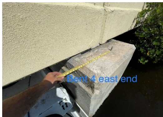
Sample of Pile Caps
