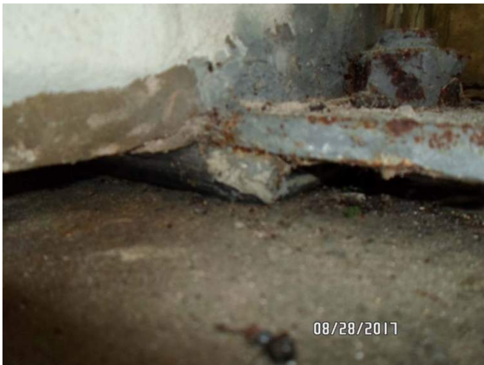
Homogeneous Area #6 (samples 016-018): Black bearing pad-end bent; bridge structure
