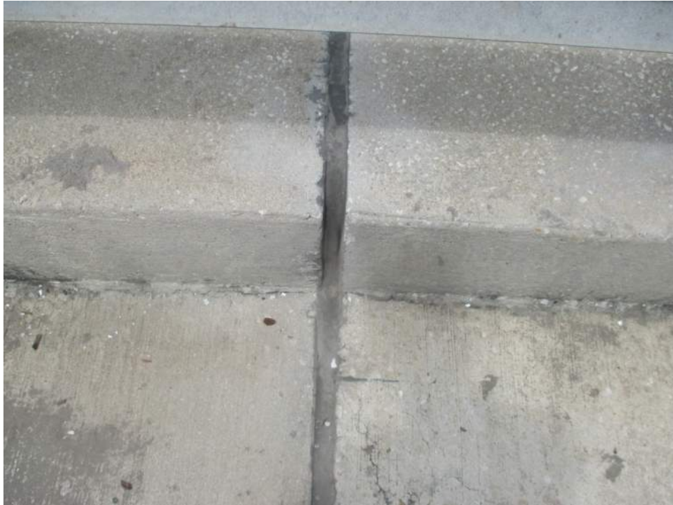
Homogeneous Area #13 (sample 037-039): Gray expansion fill-sidewalk
