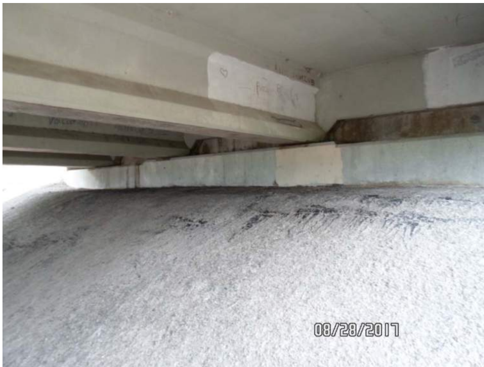
Homogeneous Area #9 (sample 025-027): Gray deck concrete, west end of bridge
