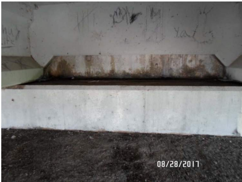
Homogeneous Area #8 (sample 022-024): Gray end bent concrete
