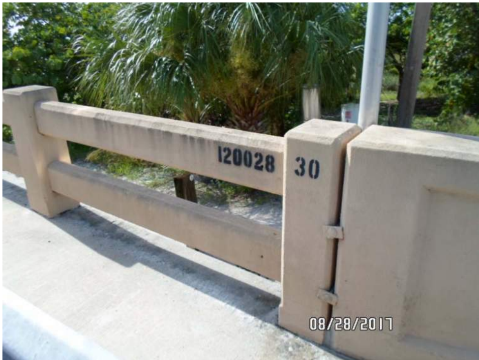
Homogeneous Area #12 (sample 034-036): Gray concrete w/tan paint-guardrail; west end of bridge
