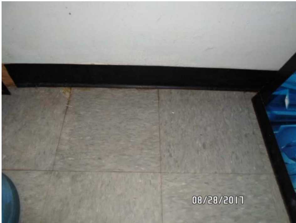
Homogeneous Area #1 (sample 001-003): 12"x12" Gray VCT w/brown mastic; tender house
