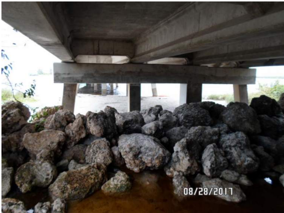
Homogeneous Area #14 (sample 040-042): Gray pile concrete
