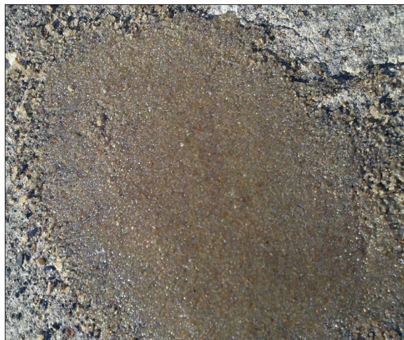
Pit patched with epoxy and sand
