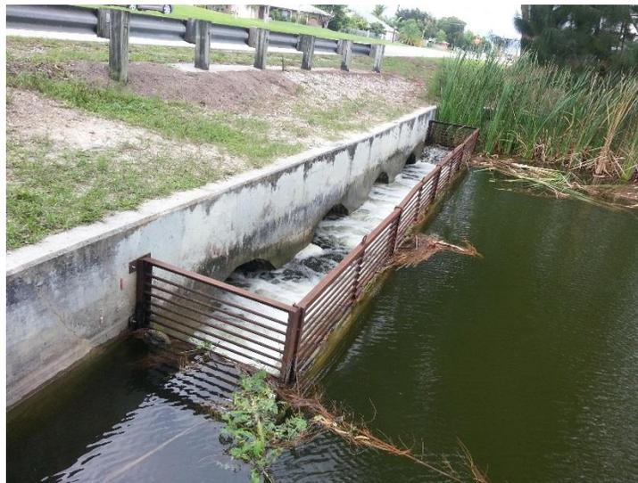
Figure 23. High flows through Weir 20 on 7/16/2014. Culverts are almost full after a short rainfall event. High-water marks are visible well above the culvert crests.
