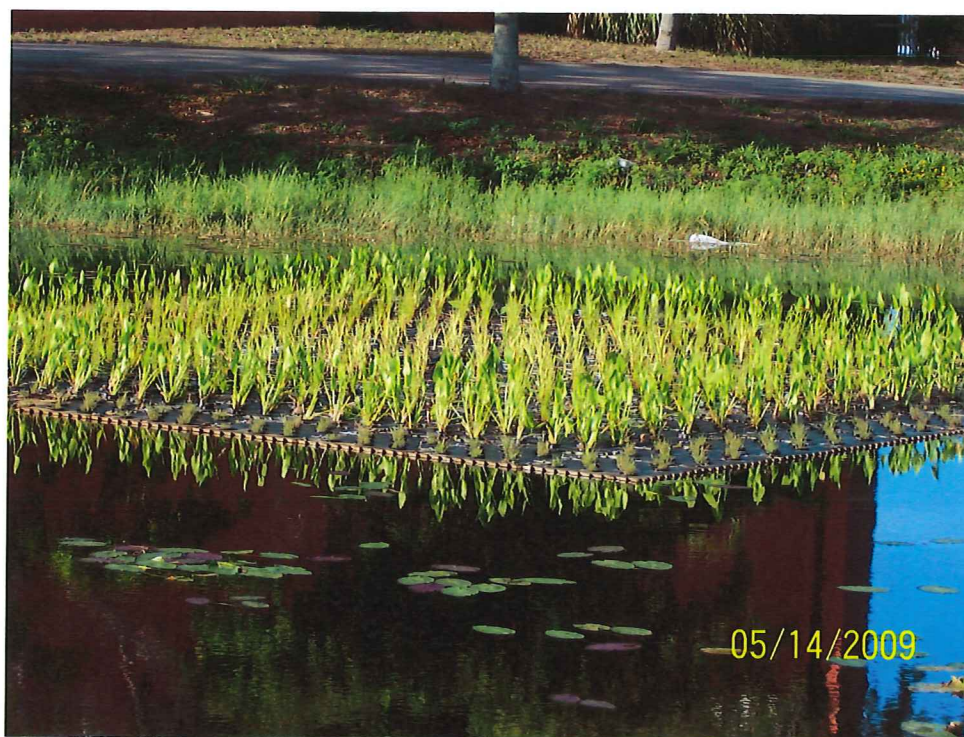
Figure 4: Completed Existing Mat Placement in Mulloch Creek
