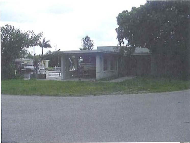
Carport and front elevation
