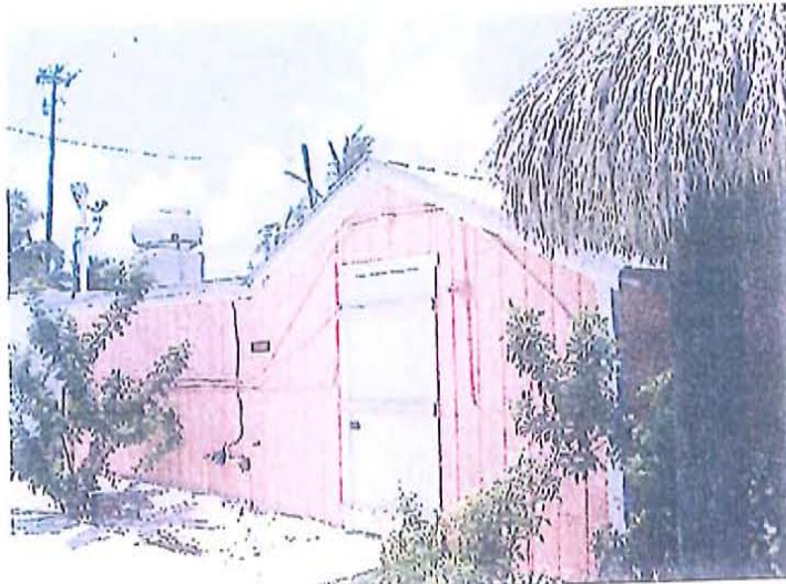
Rear elevation of the Snook Inn view to west
