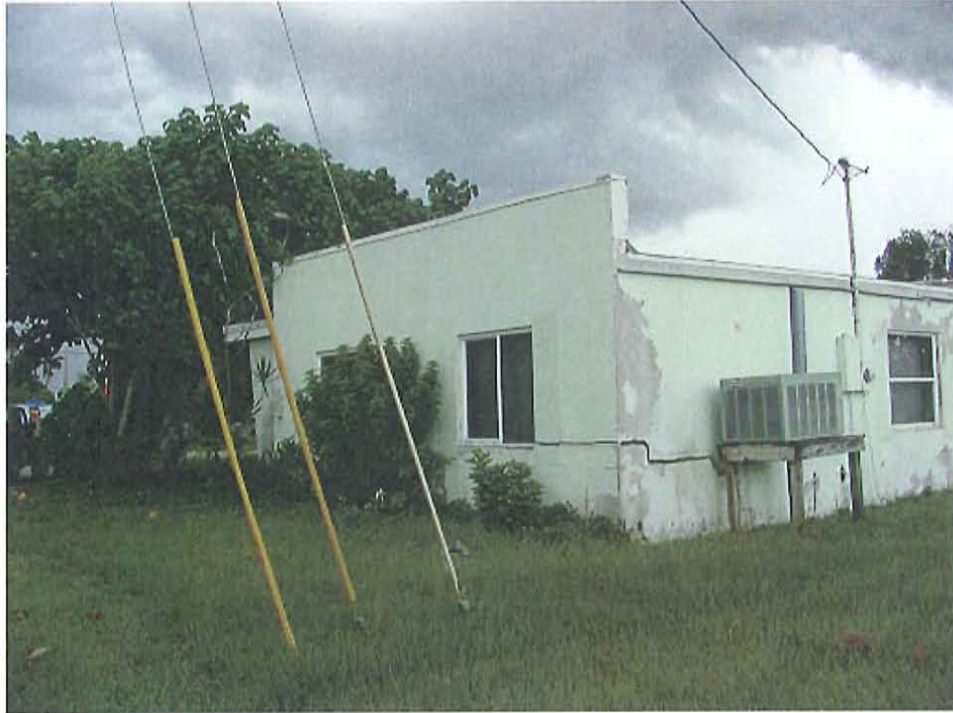
East side and rear elevations (note crack in the wall)
