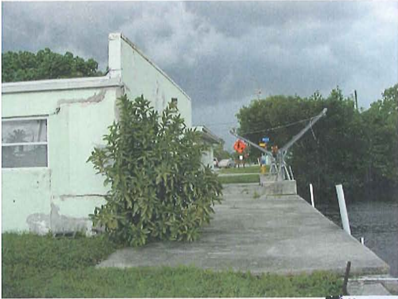
West side elevation by canal
