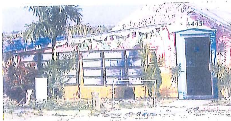
Detail of front façade windows and door
