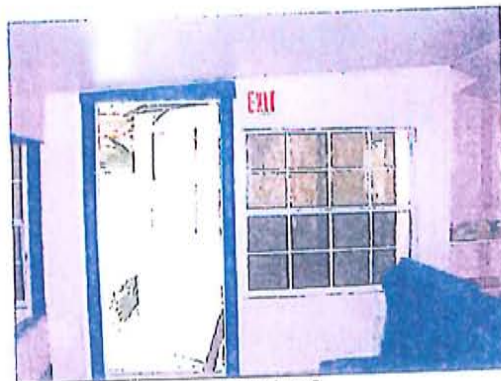
View of south wall of Dining 2
