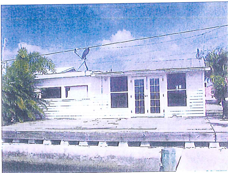
Subject Building: Rear (east) elevation by Matlacha Bay .
