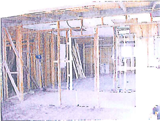
Subject Building: Interior finishes have been removed exposing support systems
