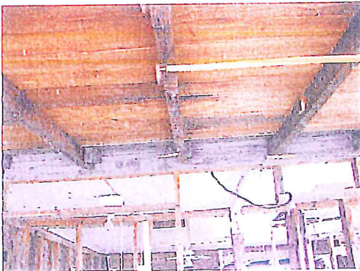
Subject property interior of the roof area at the rear -- this rear roof area was probably a separate addition
