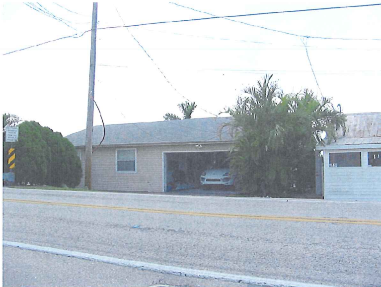
Adjoining property to the north (left) front elevation --
