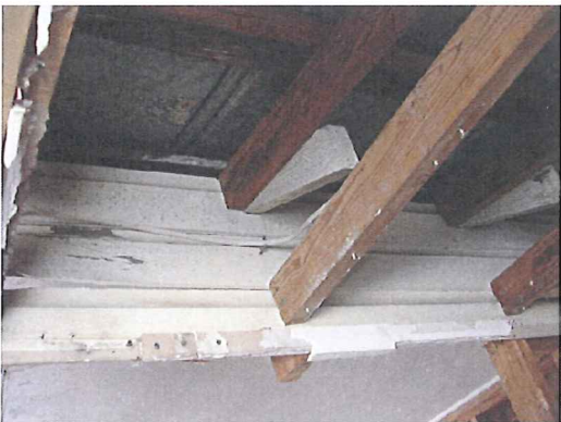
Subject Building -- enclosed porch area: exterior horizontal wood siding is visible
