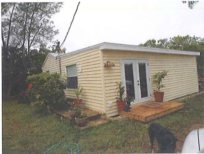
Removal of front door and side window, installation of new double French doors on side
