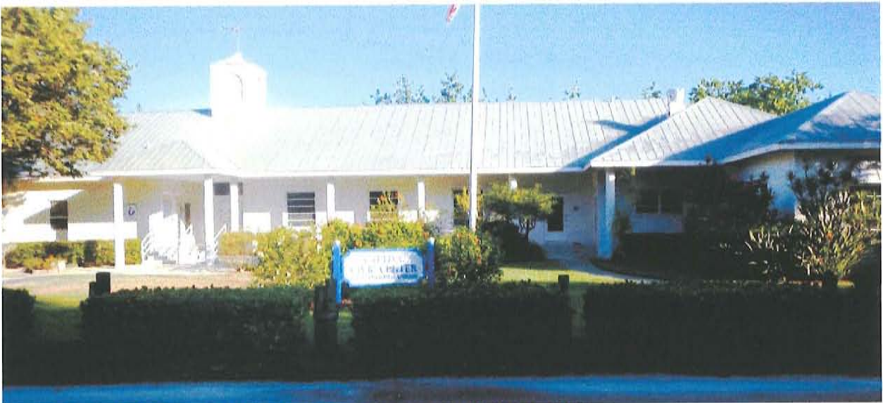
Captiva Community Center: Current Building 2013
