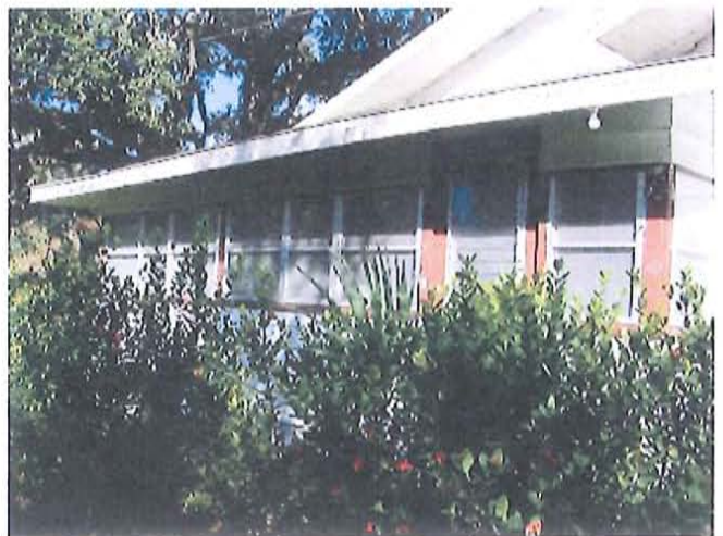
Front (North) elevation by N. River Rd
