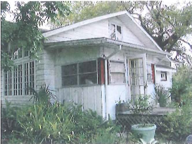
Rear South and partial of side East
