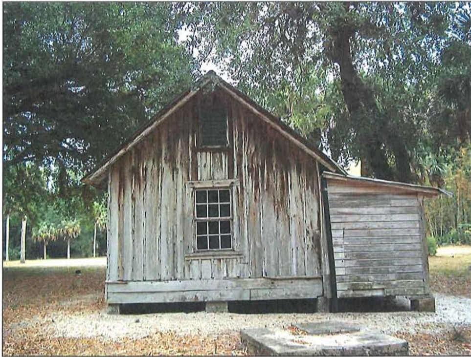
Figure #9 – North façade with septic tank cap in the foreground
