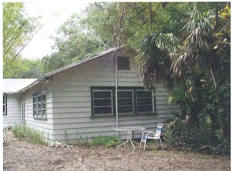
North wing gable end, which is the east elevation
