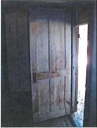
Figure #15a - West Door – Exterior
