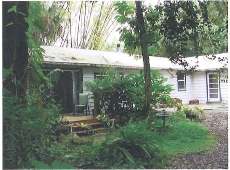
Visible T – intersection of North and South wings (east side)
