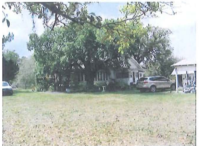
Rear South and partial of side East
