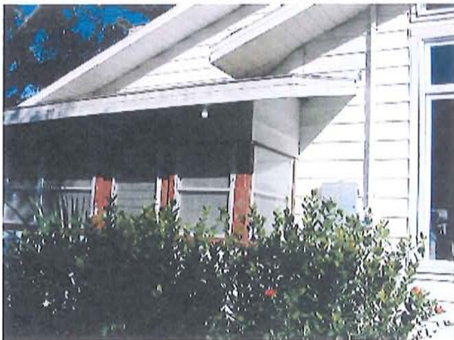
Front (North) elevation by N. River Rd
