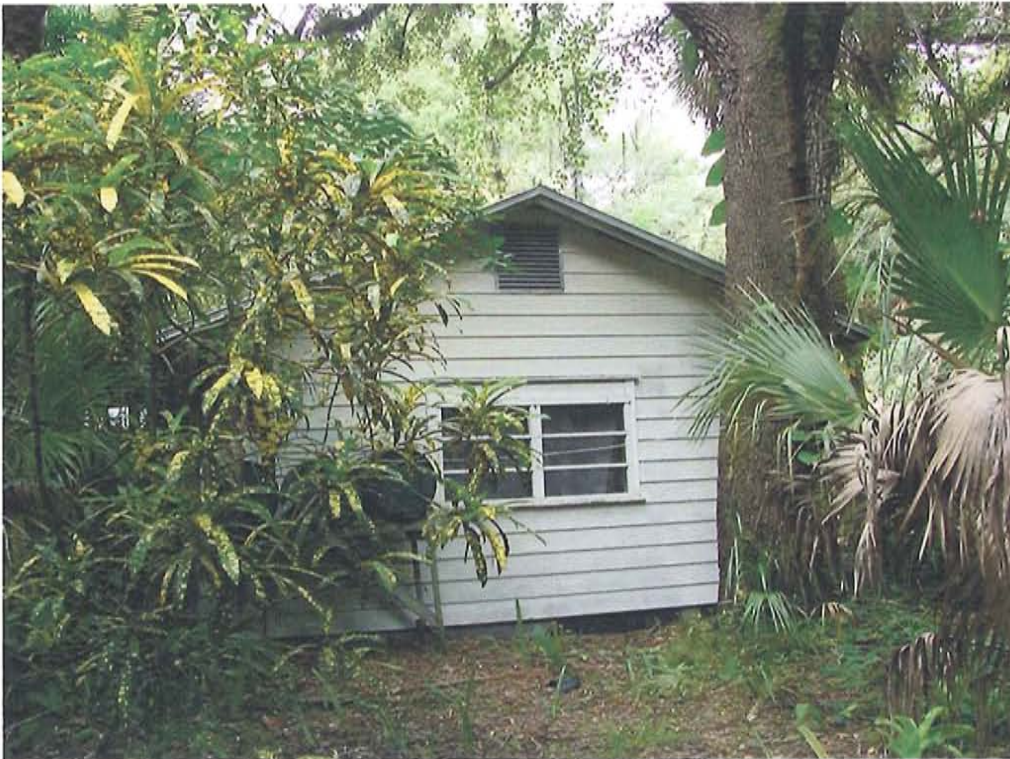
South wing – gable end
