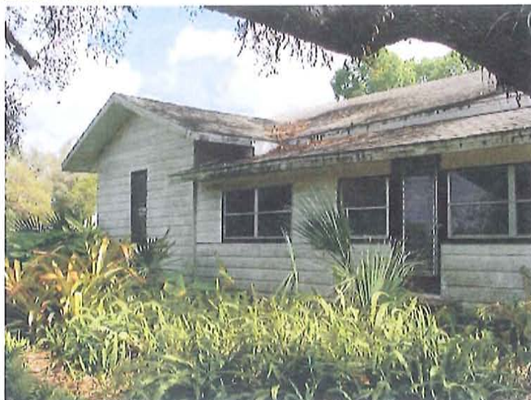
Side (West) facing Telegraph Creek
