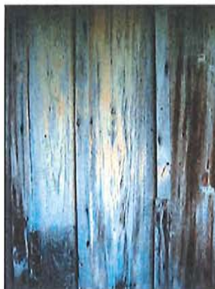
Figure #12 – Paint traces on west façade south of the bathroom addition
