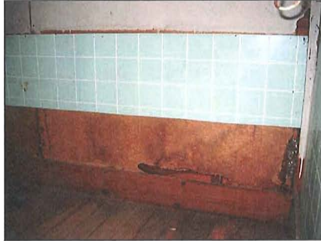
Figure #17b North wall of Bathroom section with plastic wall covering
