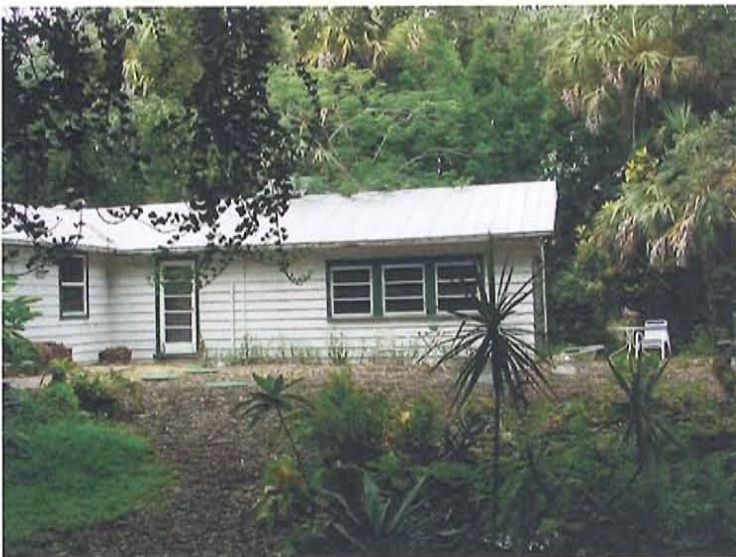
North wing (south side)
