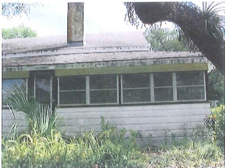
Side (West) facing Telegraph Creek
