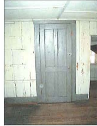
Figure #15b – West Door - Interior
