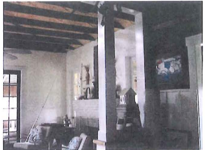
Interior front room
