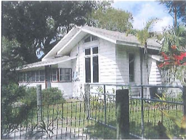
Front (North) elevation by N. River Rd
