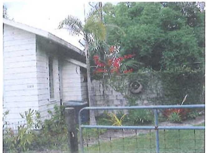
Front (North) elevation by N. River Rd
