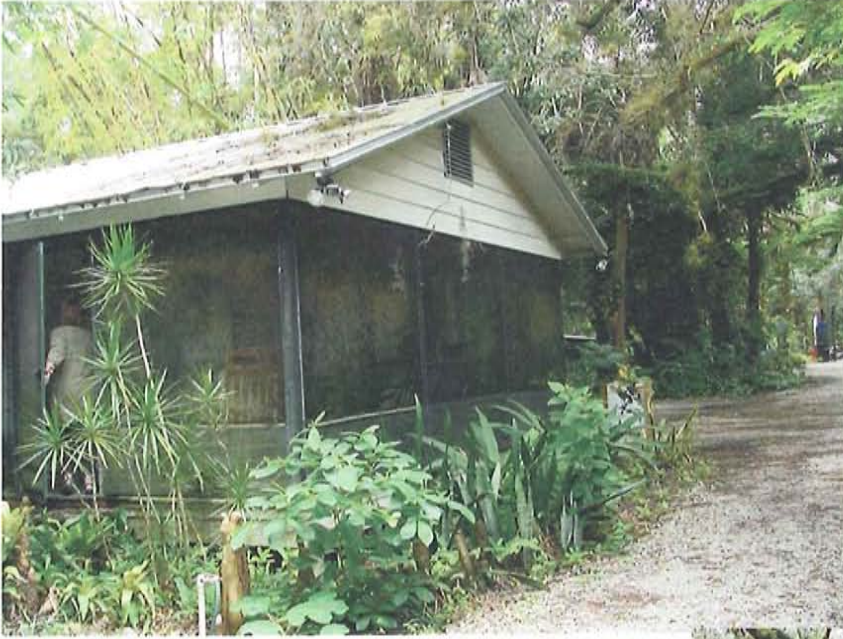
North wing – front screened porch incised under the main roof
