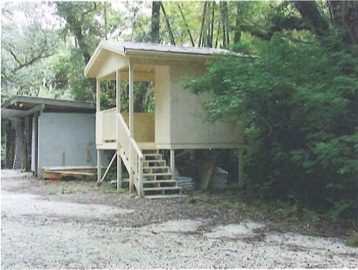
Composting toilet facility
