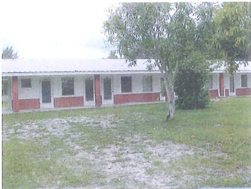
North elevation non-contributing meeting hall
