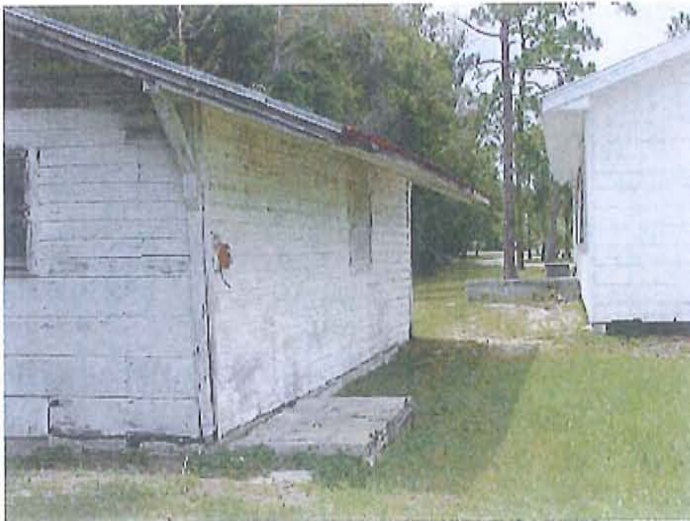
Accessory building east elevation
