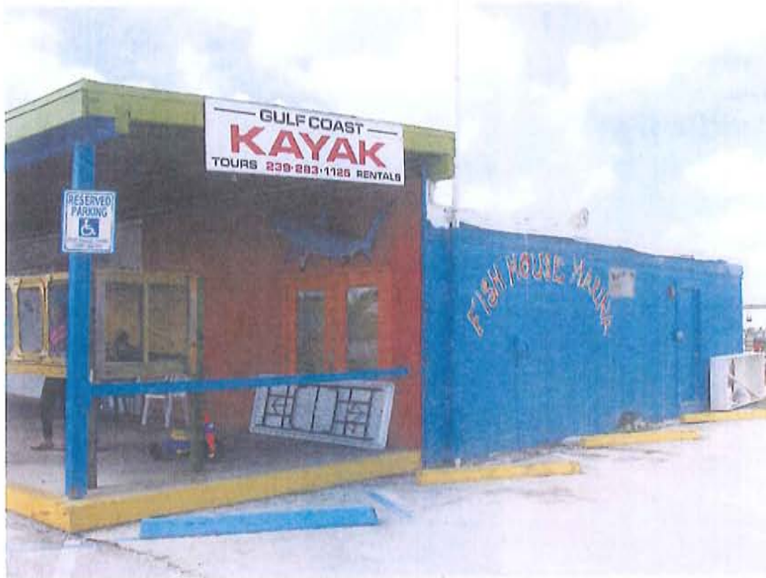
Northeast side of Fish House and end of Loading Dock 2012 – View from parking area (looking west)
