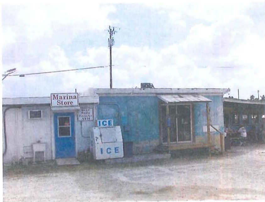
North side of Fish House processing room, (now office and cold storage access) 2012 – View from shell drive (looking south)
