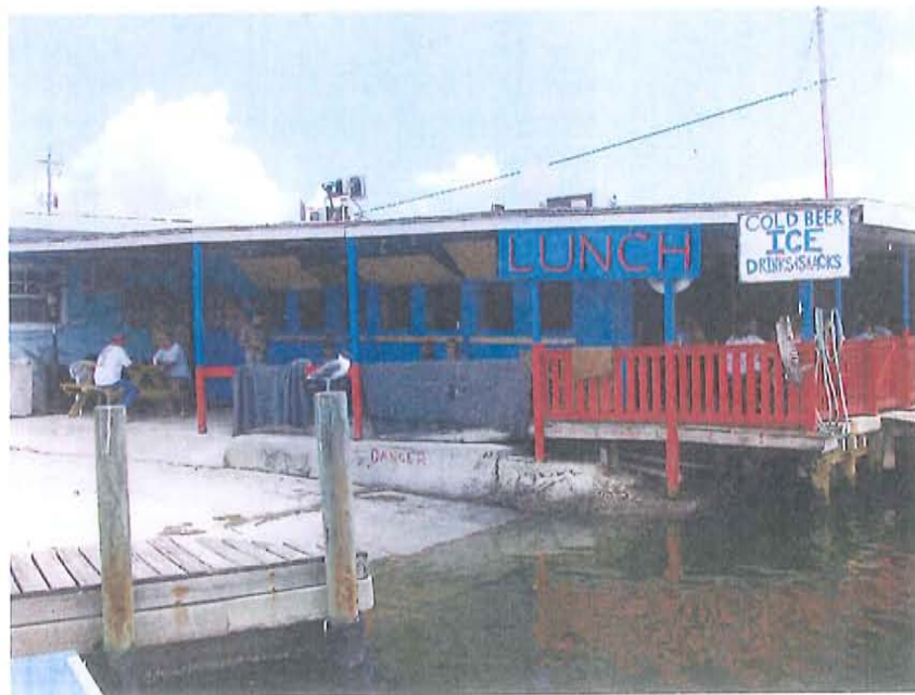
Southwest corner of Fish House, oyster processing wall, fresh catch take-in shed 2012 – View from dock west of boat ramp (looking east)
