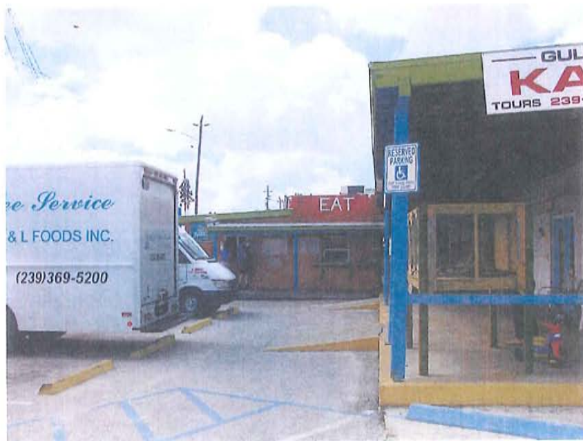
East end of Loading Dock, Take-out beyond 2012 – View from northeast, designated parking area (looking southwest)
