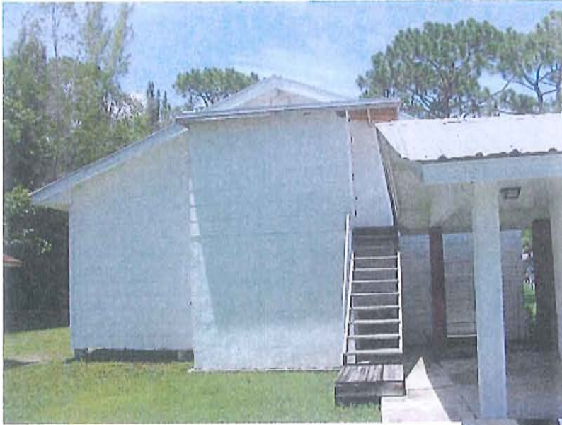
Rear elevation showing stairs leading to the door accessing the Baptismal pool
