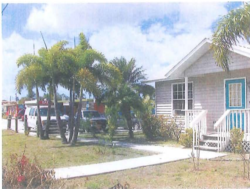
Contributing historic residential structure and parking beyond, 4520 Pine Island Road 2012 – View from northeast (looking west)
