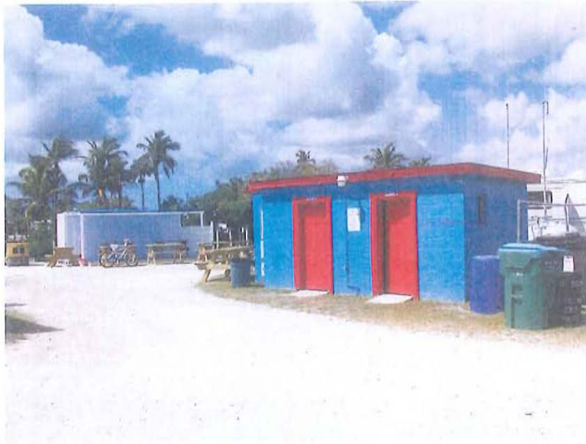
South side of Bath House, picnic tables and storage unit beyond 2012 – View from shell drive, looking toward Matlacha Pass (looking west)
