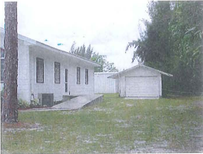
Accessory building north elevation
