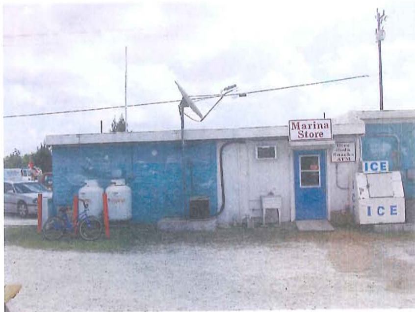
North side of Fish House, cluster blue crab & cold storage room (now Ship's Store) 2012 – View from shell drive, looking toward PI Road (looking southeast)
