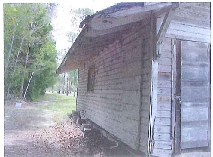
Accessory building west elevation
