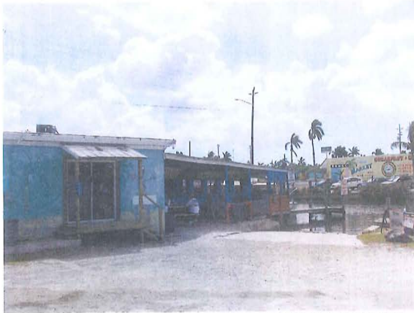
North side of Fish House, oyster processing wall, fresh catch in-take shed 2012 – View from shell drive, looking toward Pine Island Road & Matlacha Pass (looking south)
