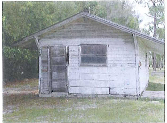
Accessory building south elevation
