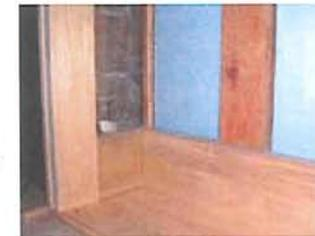
**Recommended:** [54] This rigid insulation has been correctly installed in the wall cavity so that when the gypsum board is hung the original proportion and relationship of the wall to the trim will be retained.
