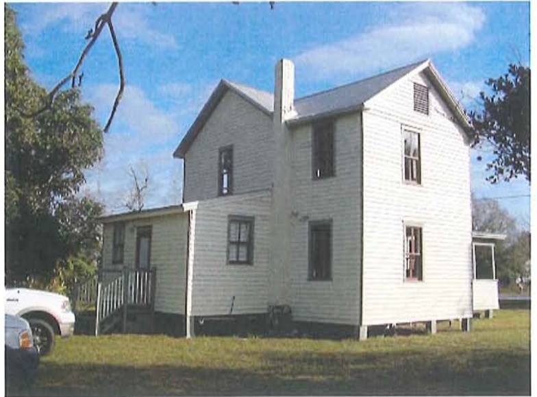
Rear (West) Side (South)
