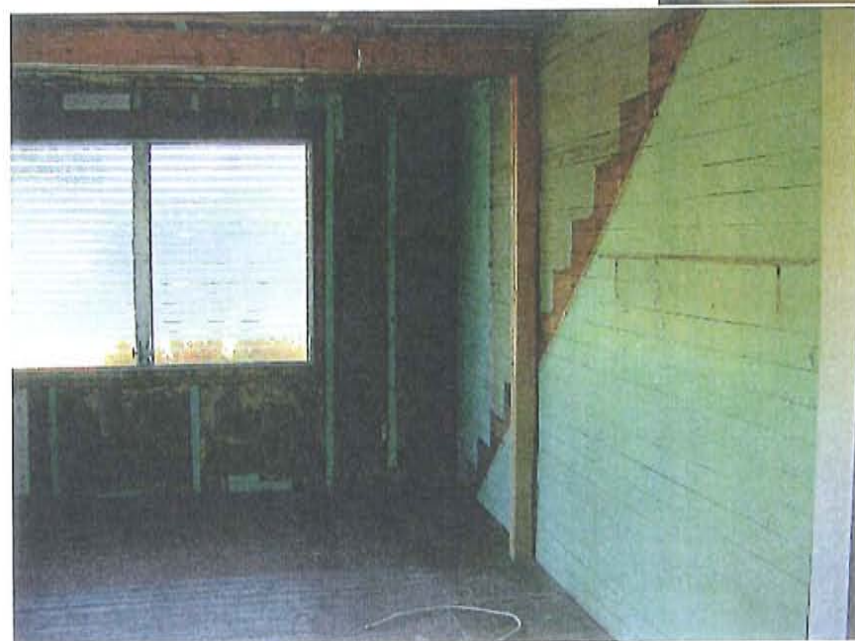
Existing living area showing the house originally is likely to have had interior stairs to the attic
