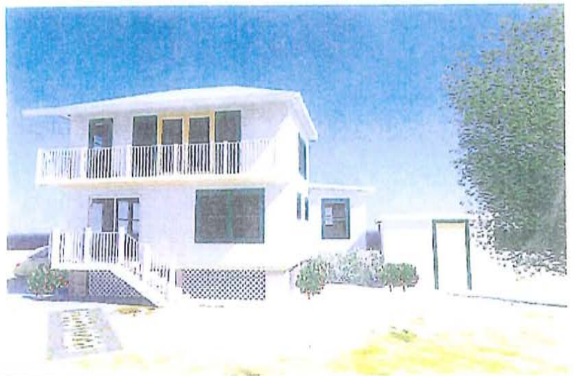
Rear (East) Side (North)
