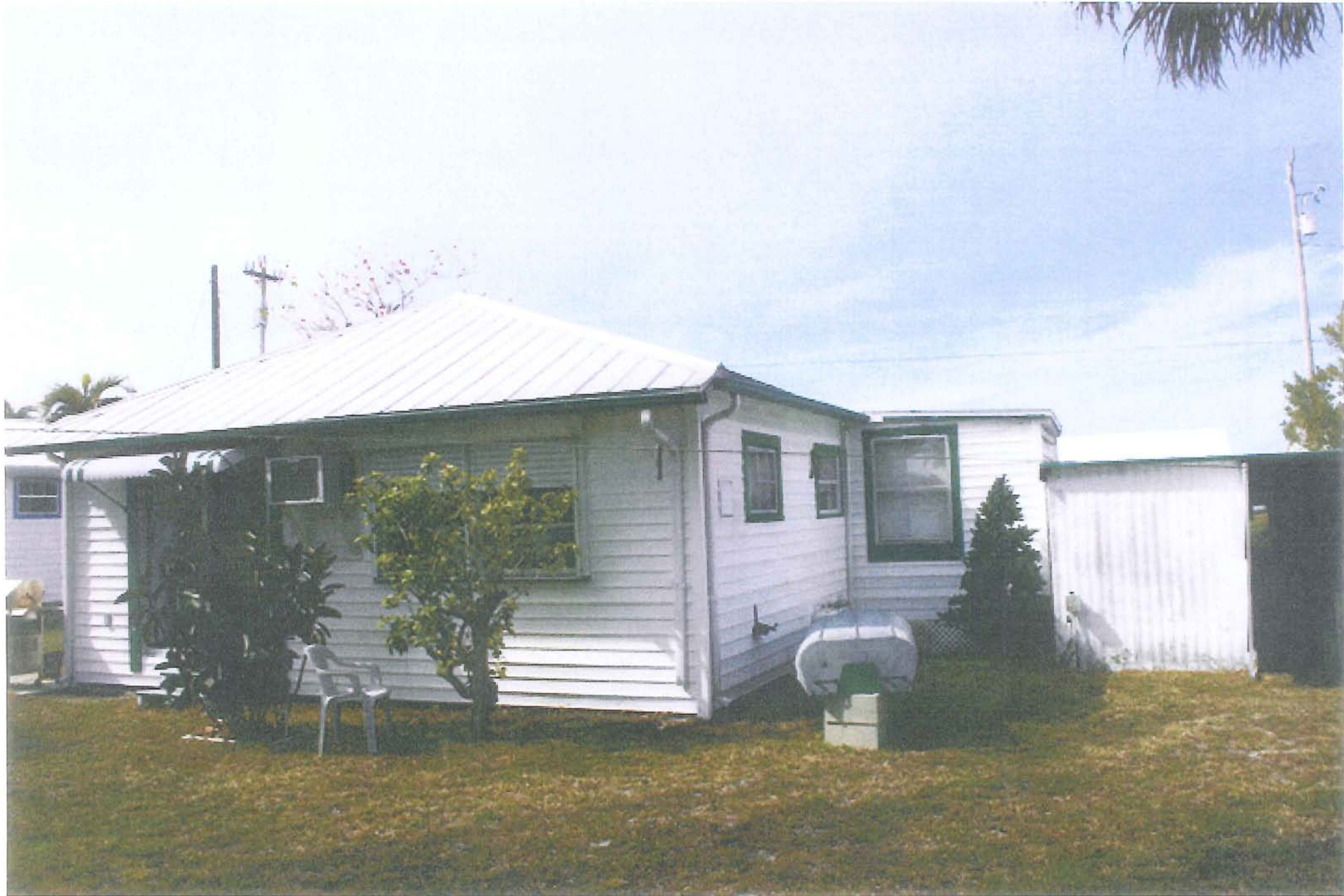
EXISTING HOUSE - REAR (EAST) SIDE (NORTH)
