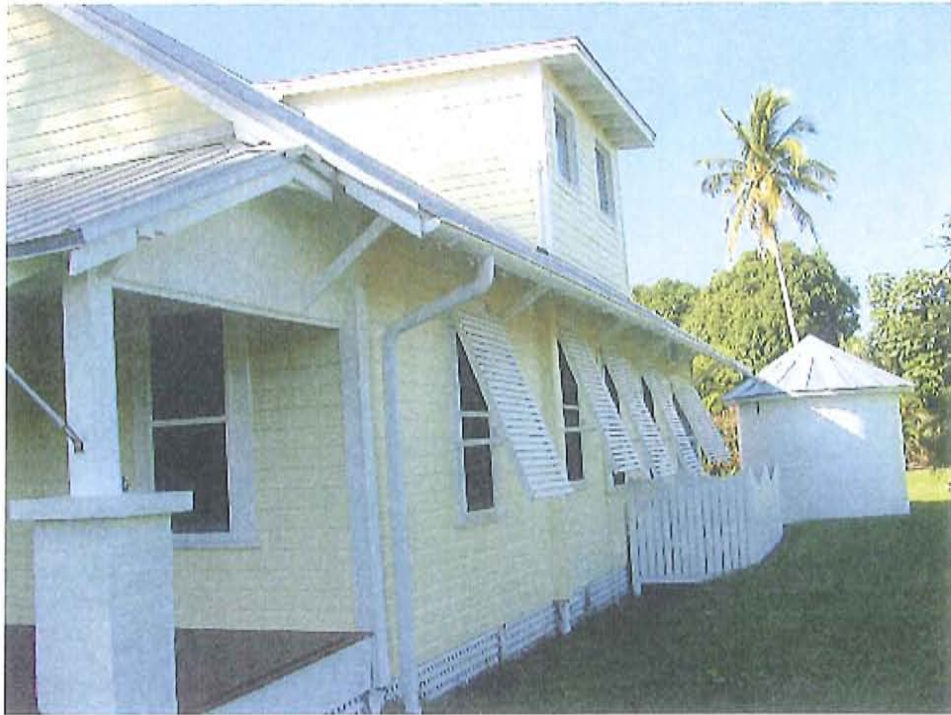
Side North (partial of the front elevation and cistern at the rear)
