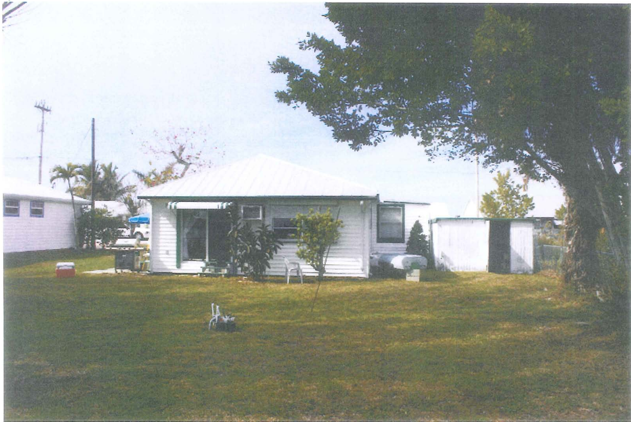
EXISTING HOUSE - REAR (EAST) SIDE (NORTH)
