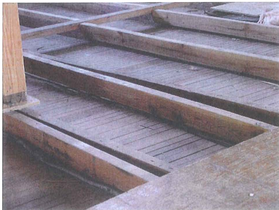
Structural problems on the floor system of the second level
