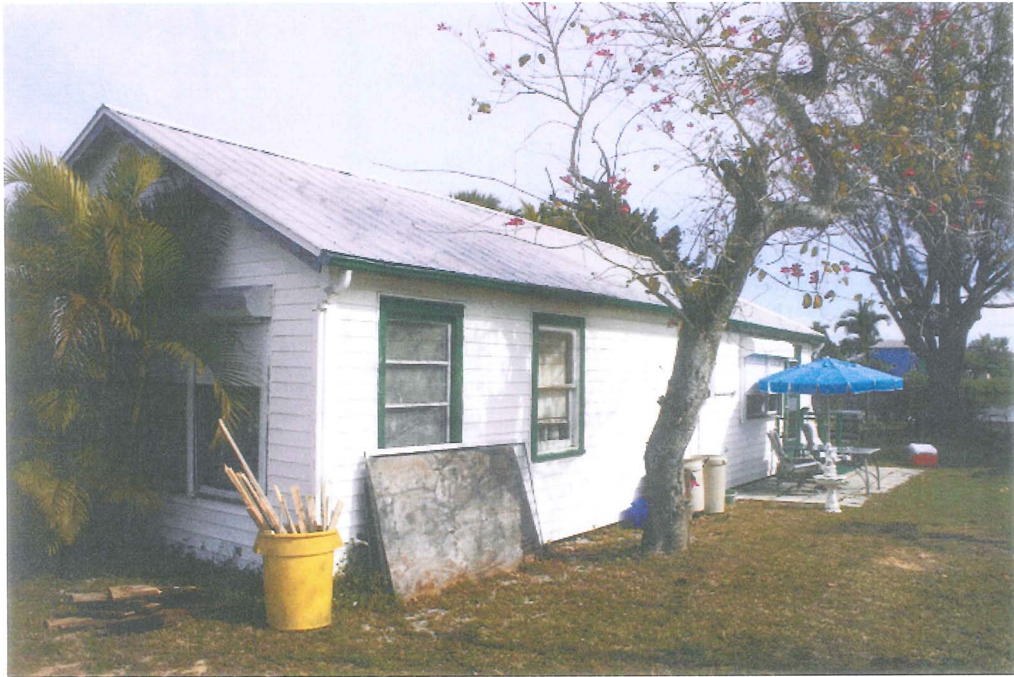
EXISTING HOUSE - SIDE (SOUTH)
