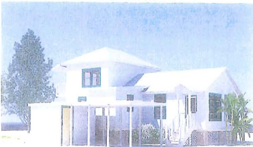
Rear (East) Side (North)
