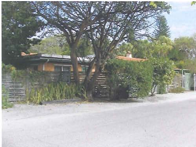
Site # 6 920 Palm Ave. West (side) elevation
