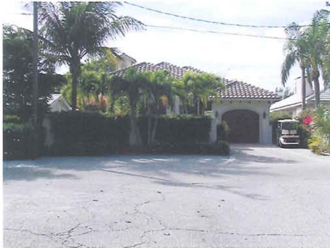
Site # 5 801 Palm Ave. East (front) elevation
