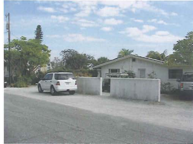
Side (north) elevation on 9 th St E
