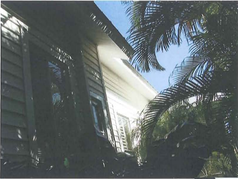
South side of the subject property
