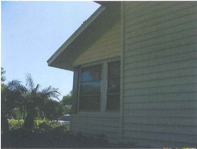
North side of the subject property on 3 rd St.
