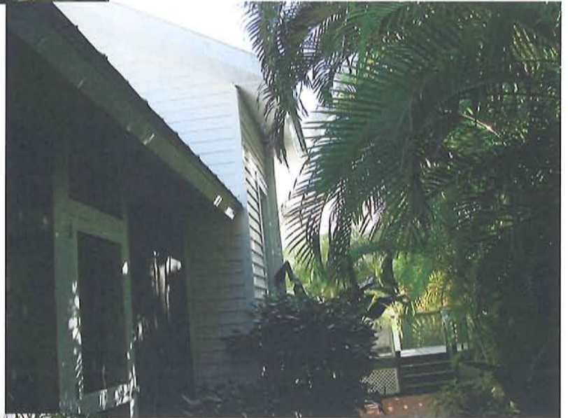
South side deck to be removed
