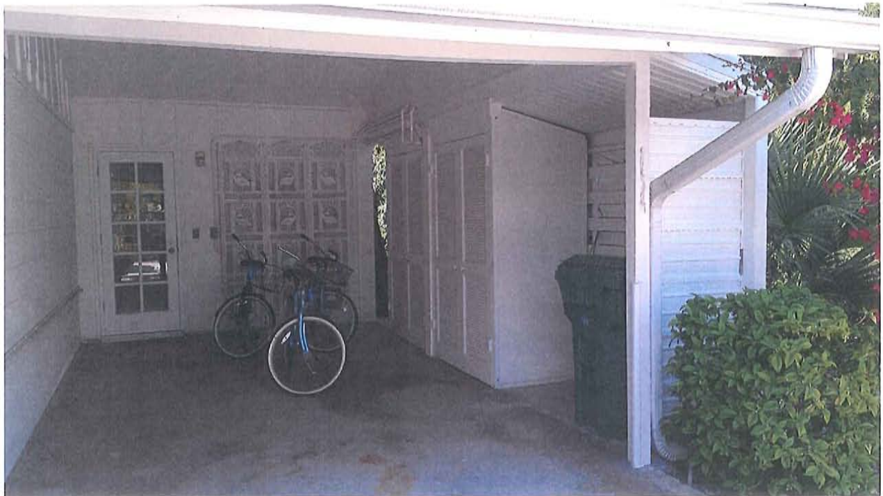
Side (North) Interior of carport
