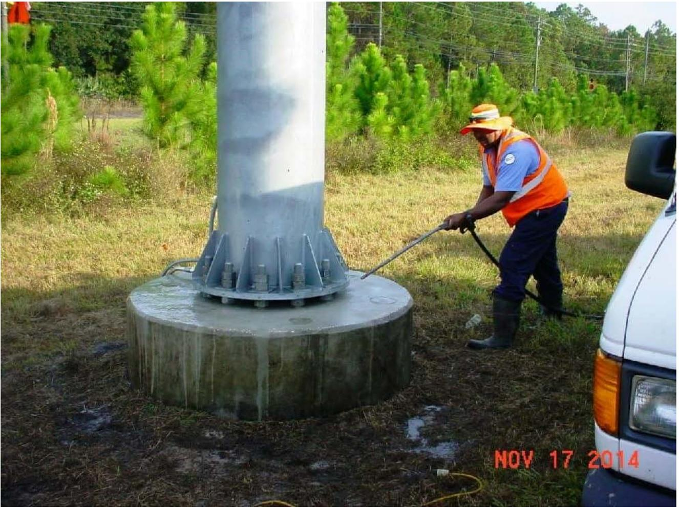
**The water and any residue is then blown off with high pressure air.**
