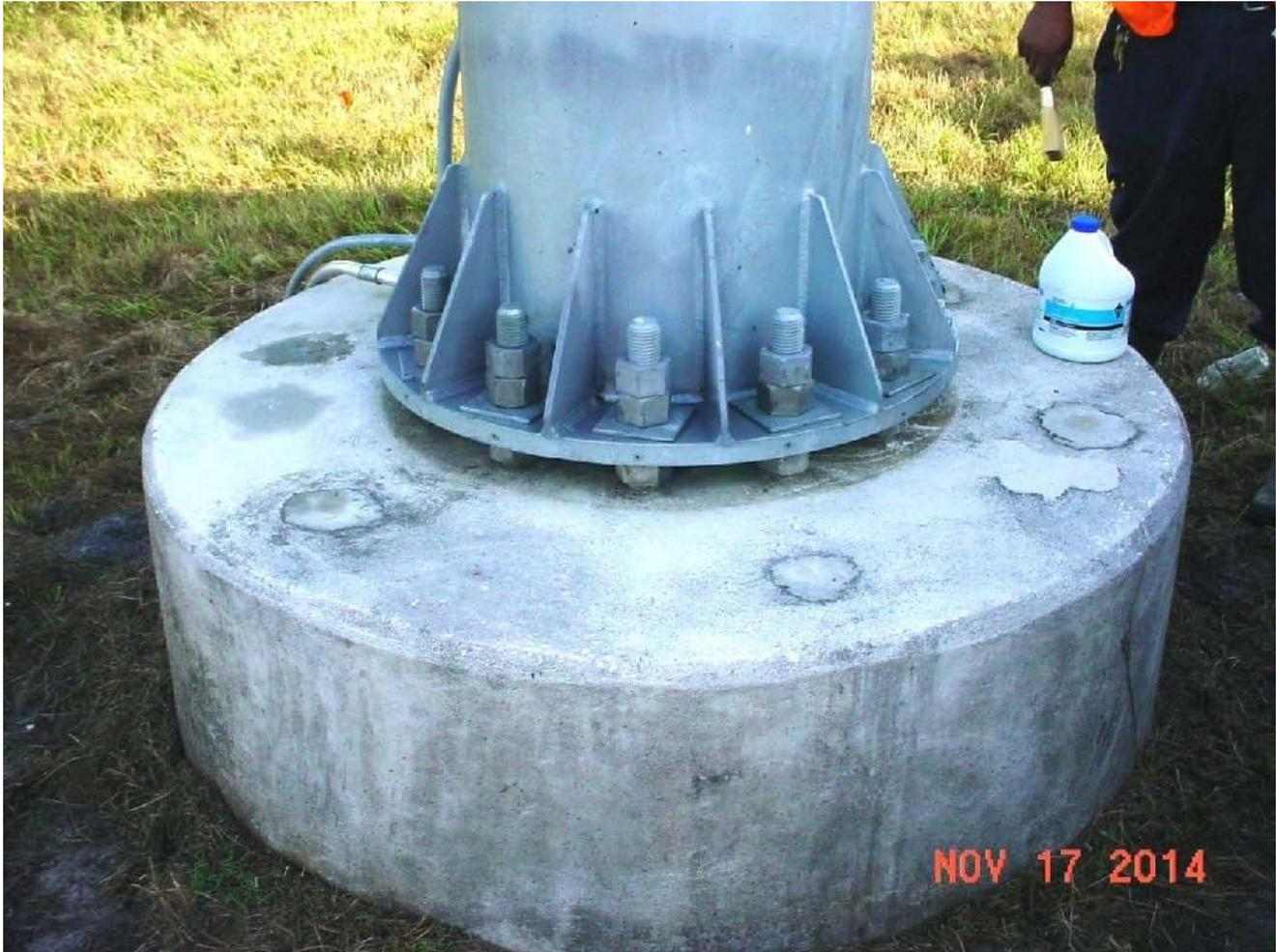
**If Foundation has mildew on top and under the structure.**
