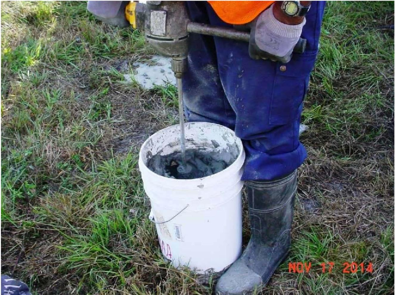
**A suitable mixing container with a mixing paddle is used with this bag pour.**
