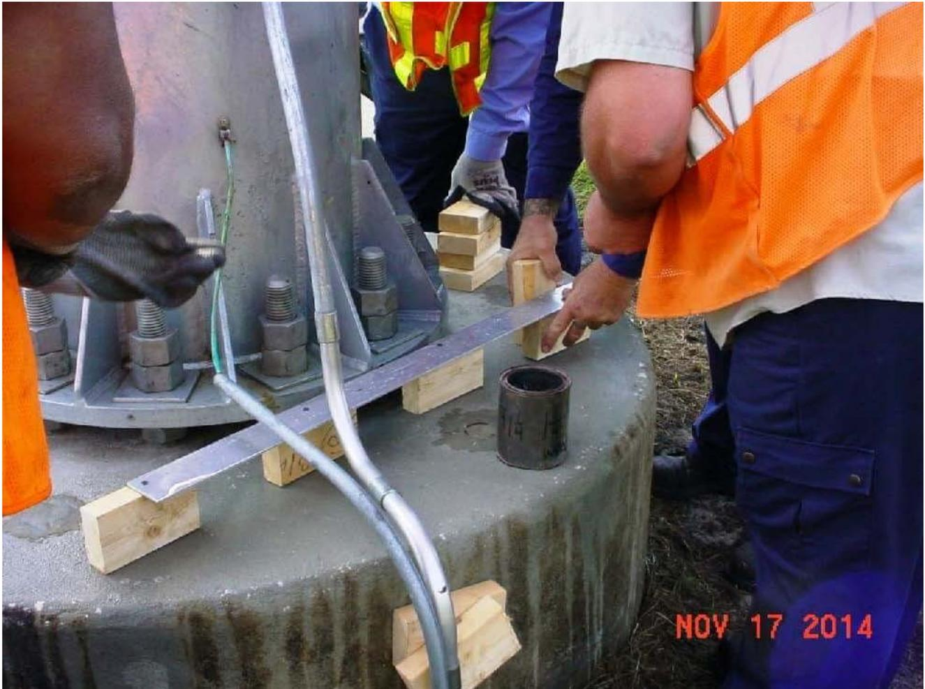
**Forms can be constructed from old aluminum signage or bender board.**
