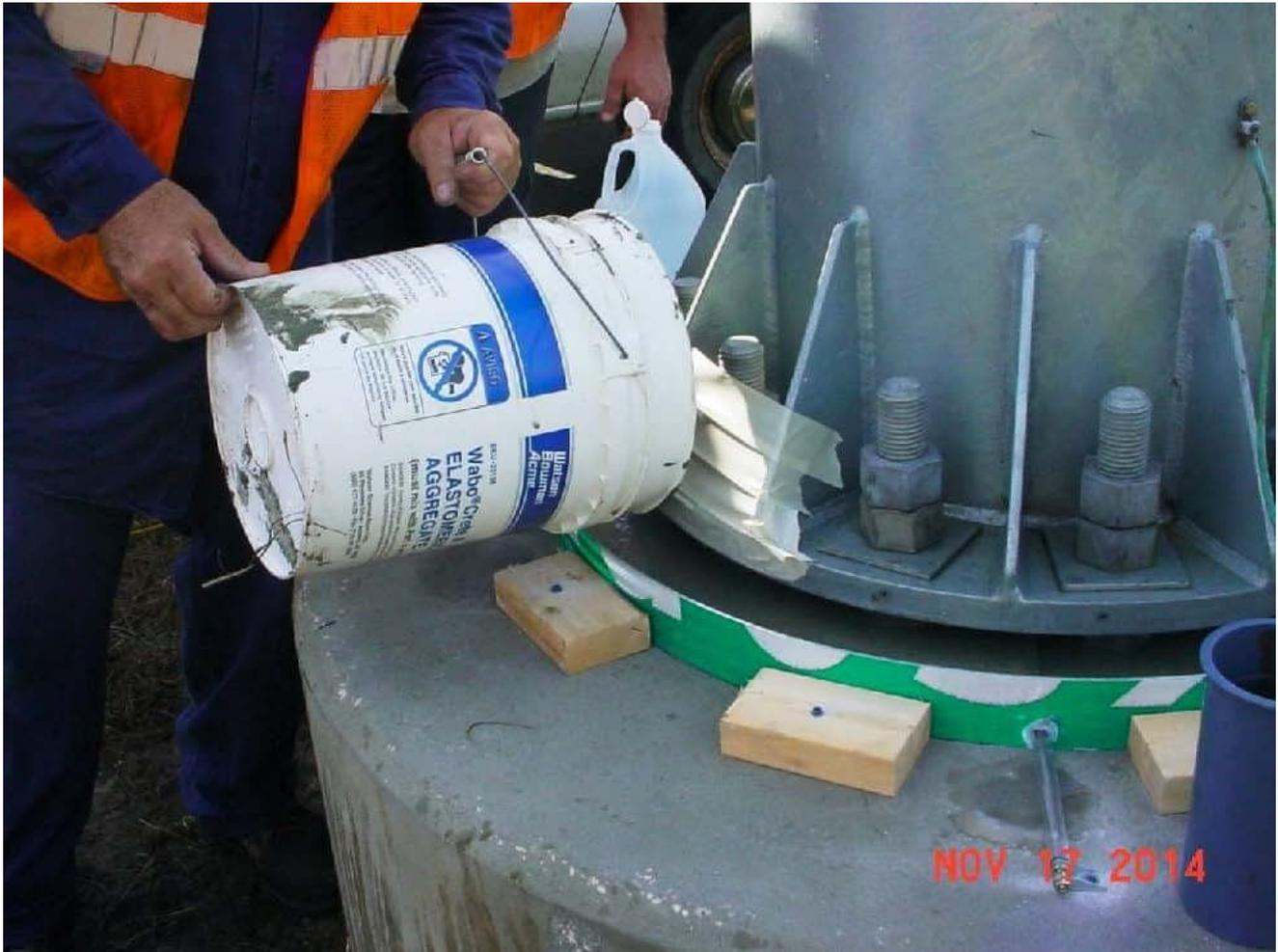
**The grout is then poured on one side as much as possible.**
