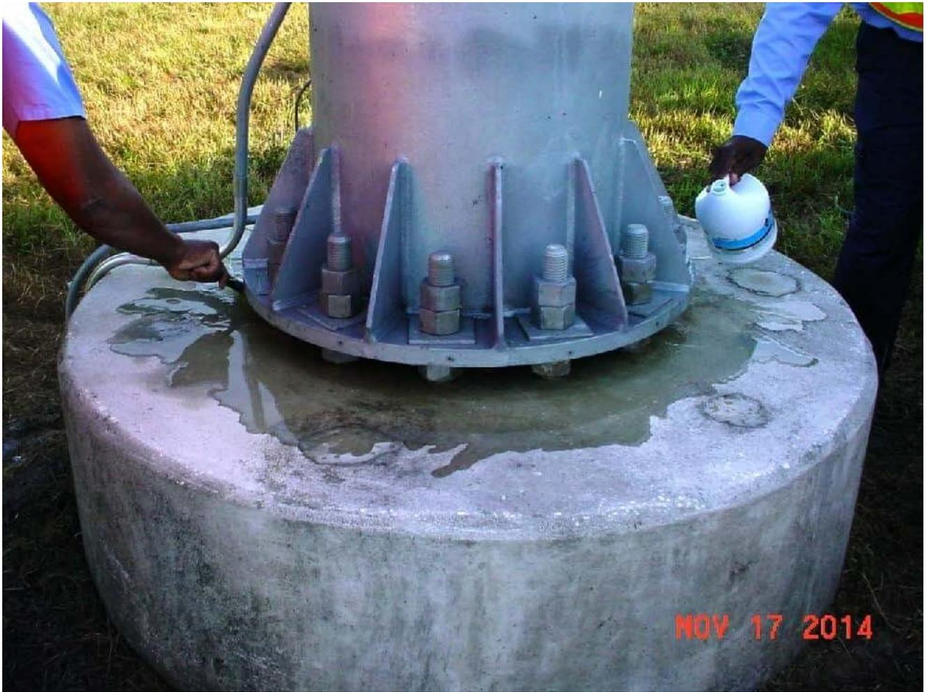
**A chlorine solution is used to remove the mildew from the top of the foundation.**
