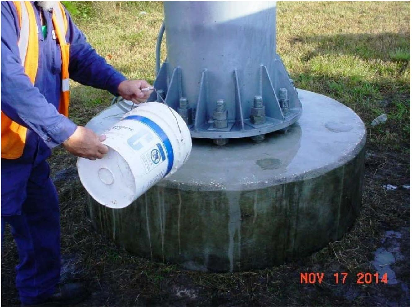
**The chlorine solution is then washed off.**
