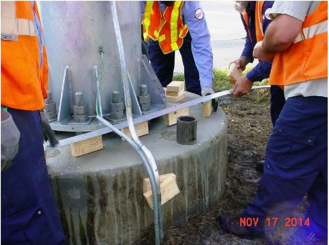
**Blocks are screwed to the form for mounting of the form to the top of the foundation.**
