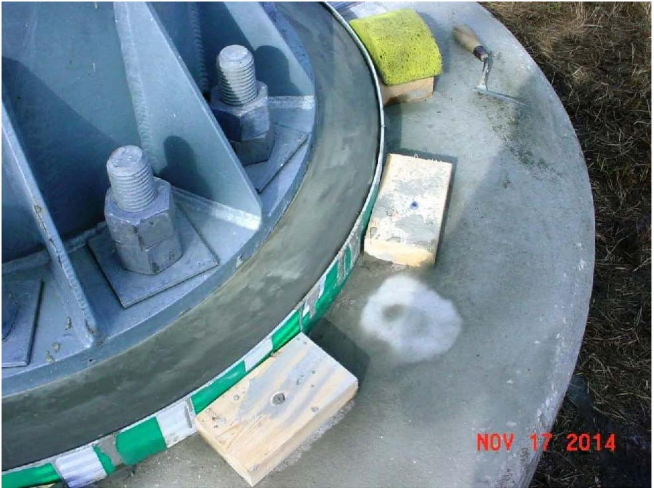
**With a trowel the outside top edge is rounded as the grout is setting.**
