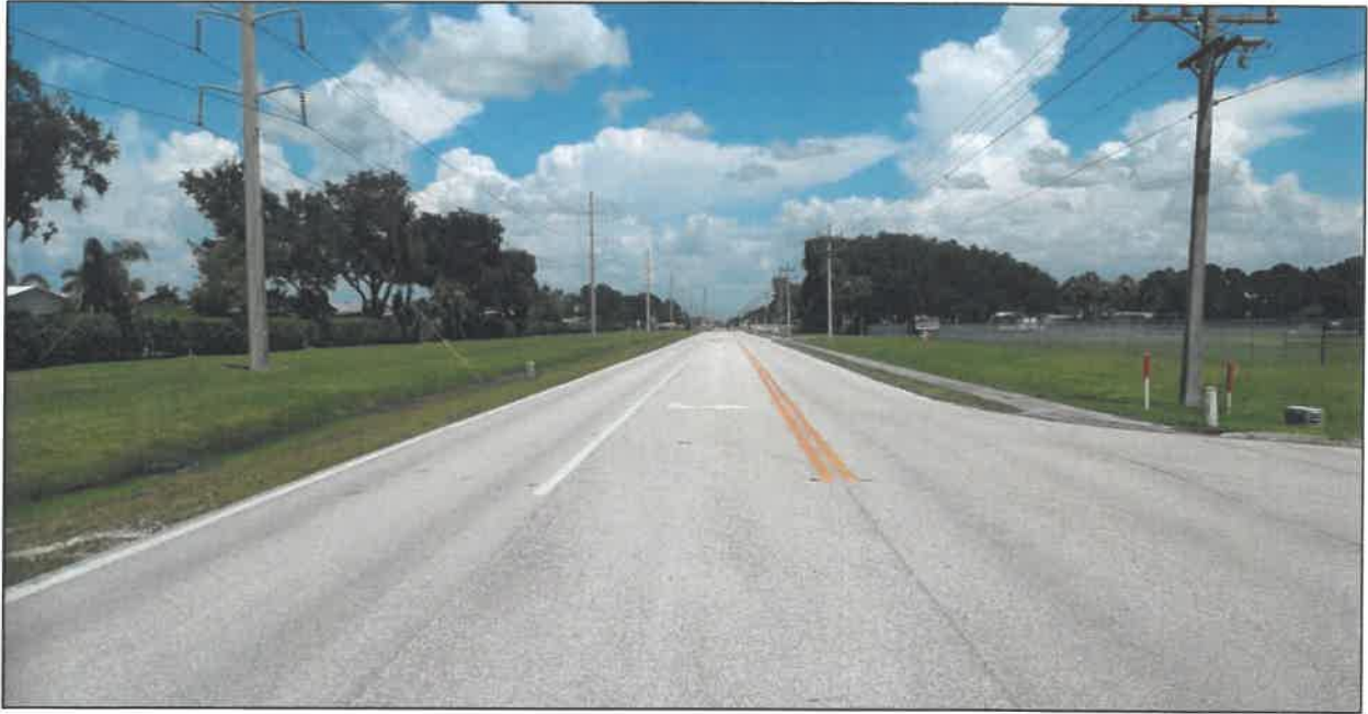
Figure 2-2 - Littleton Road Looking East from Hutto Road
