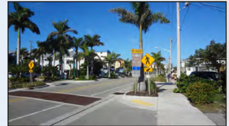
North End - Estero Boulevard
